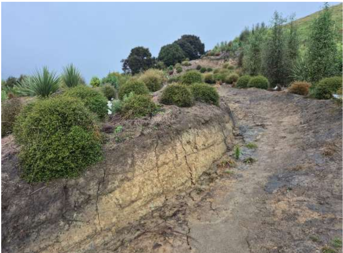
Photo 6. Tension cracks within Zone C.
