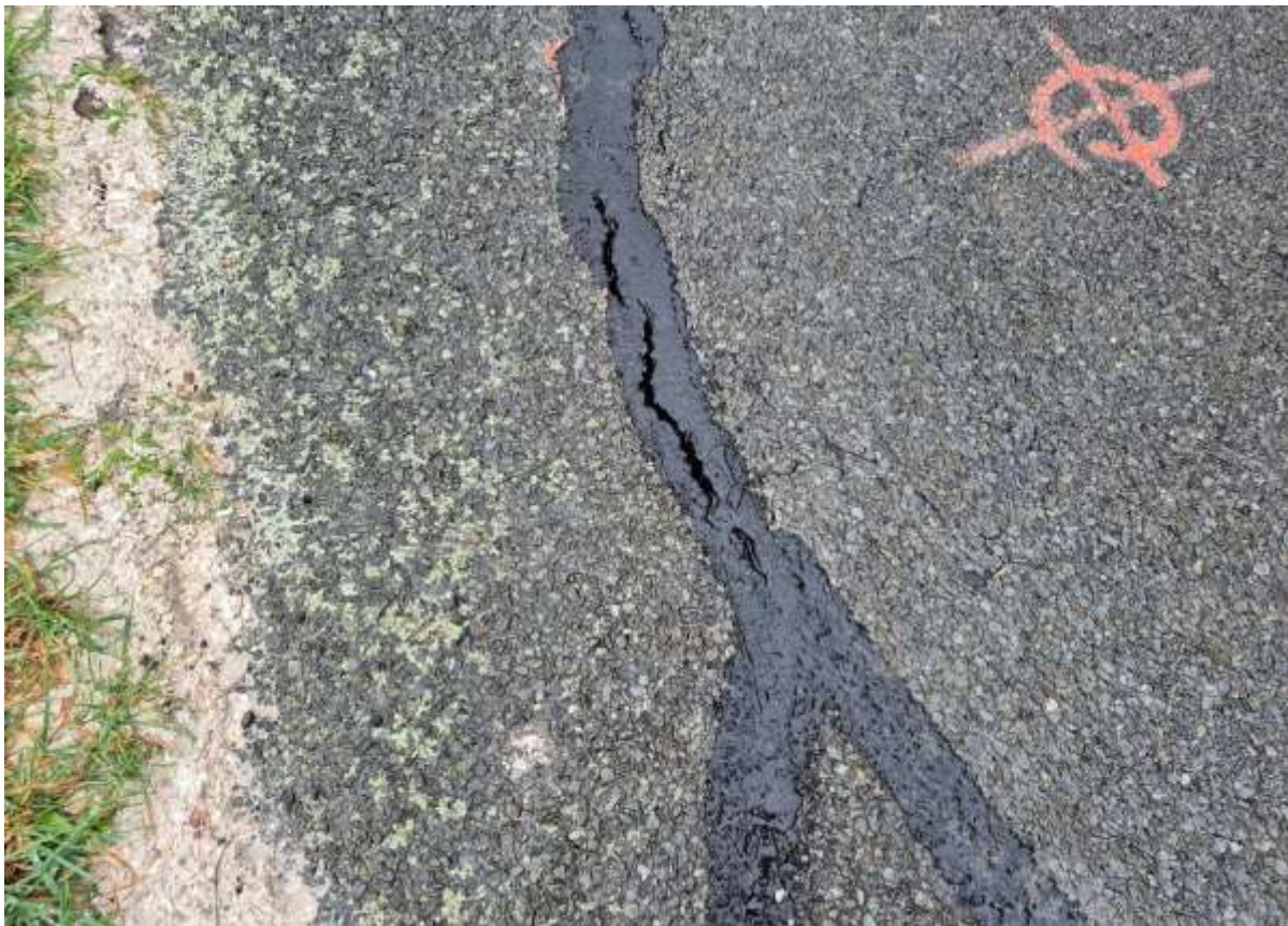
Photo 3 & 4. Evidence of continued movement in tension cracks within Lighthouse Road.
