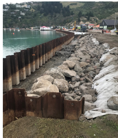
Above: rock revetment construction
