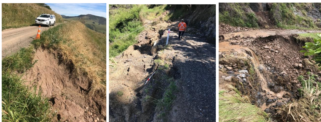
Above: The sides of the road have dropped away.
