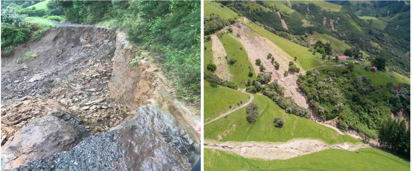
Above: Goughs Road, where approximately 30 metres of the road dropped away to 12 metres below its original position.
