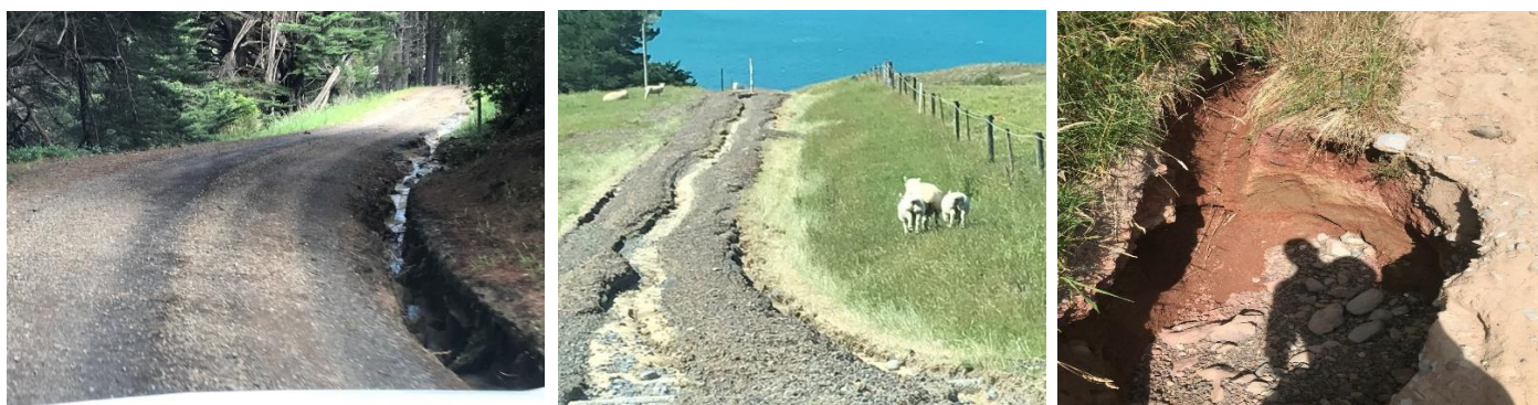
Above: Water has scoured out the road.
