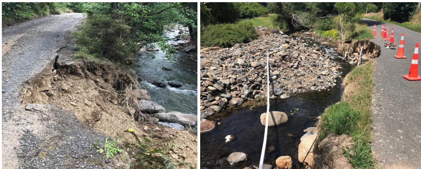
Above: The original path of water has changed and scoured out the road.
