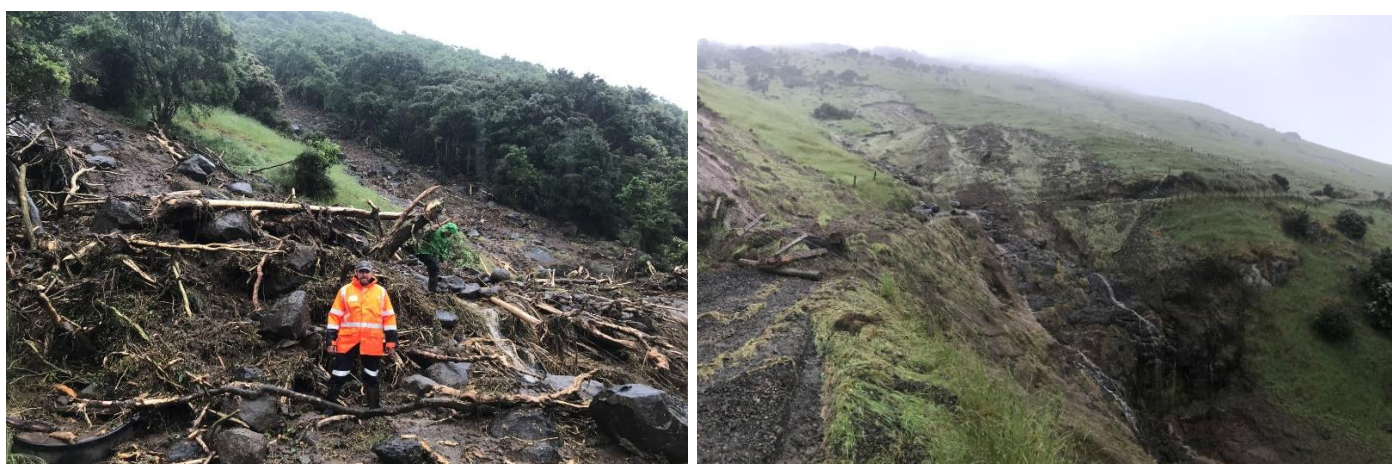
Above: Material has slipped down the hillsides and covered the road.
