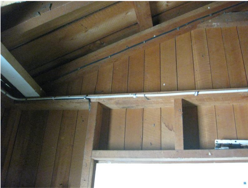
Photo 5: Typical social room vertical tongue and groove lining
