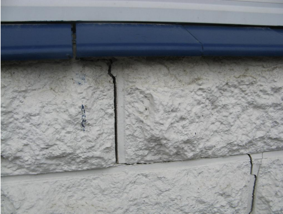
Photo 9: Damage to block wall cladding.
