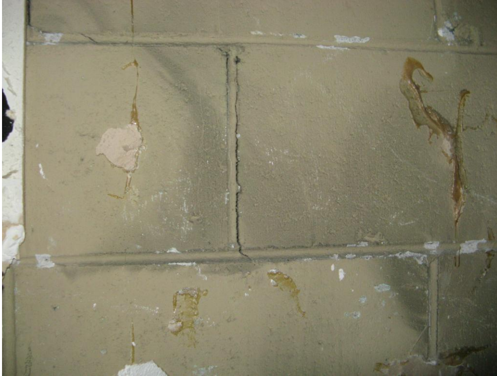
Photo 11: Damage to concrete masonry walls between units 2 and 3.
