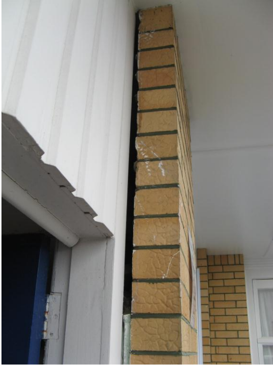
Photo 7: Separation of brick veneer cladding from timber framed wall.
