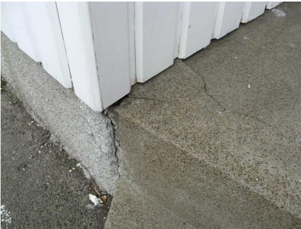
Photo 10: Damage to raised concrete slab.
