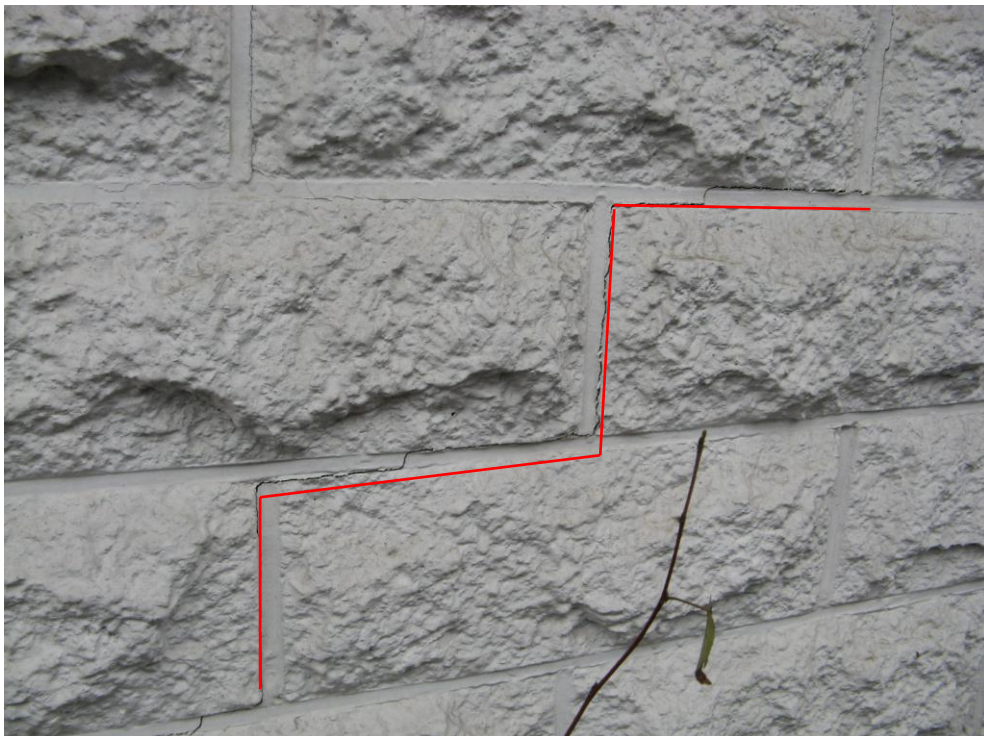
Photo 15: Damage to block wall
