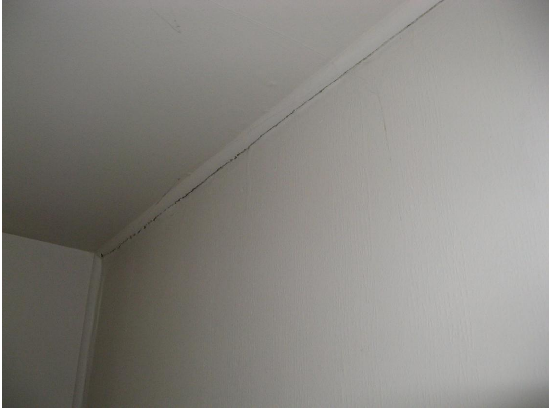
Photo 18: Typical damage at plasterboard ceiling connection to masonry walls.
