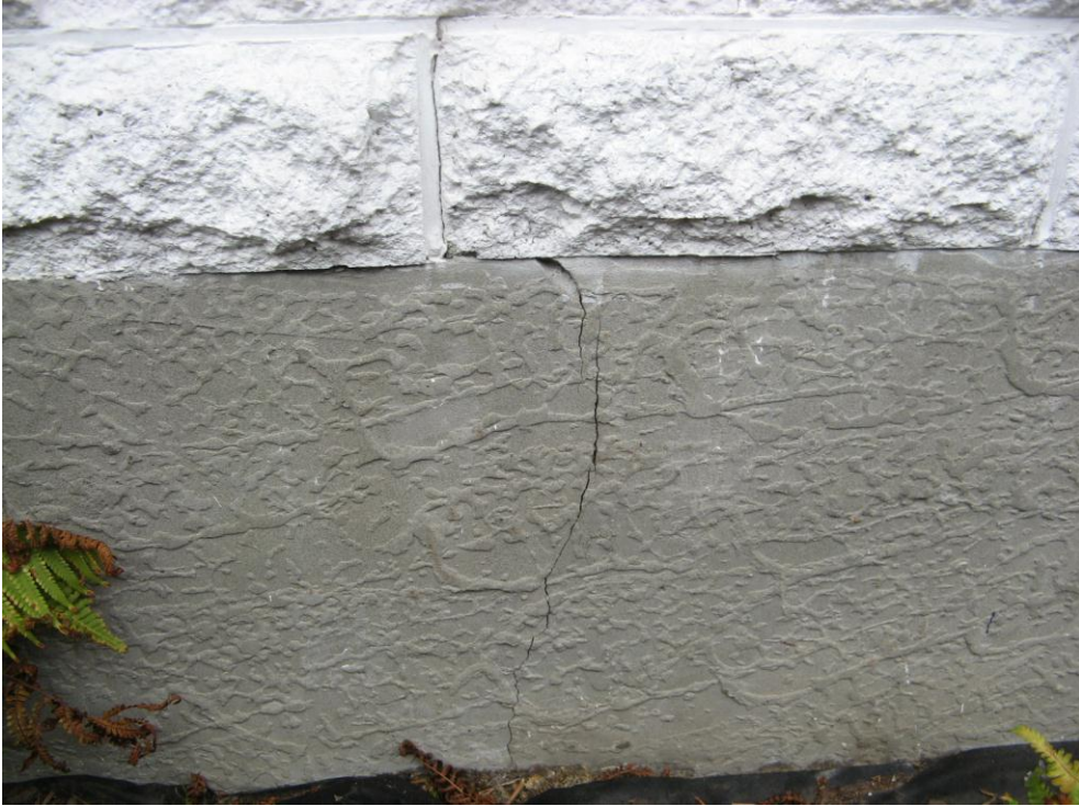
Photo 16: Damage to perimeter foundation.
