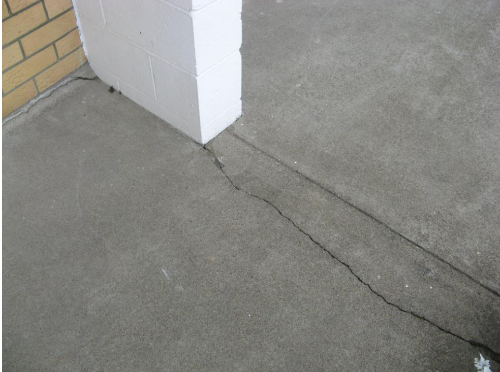
Photo 3: Damage to external raised slab.
