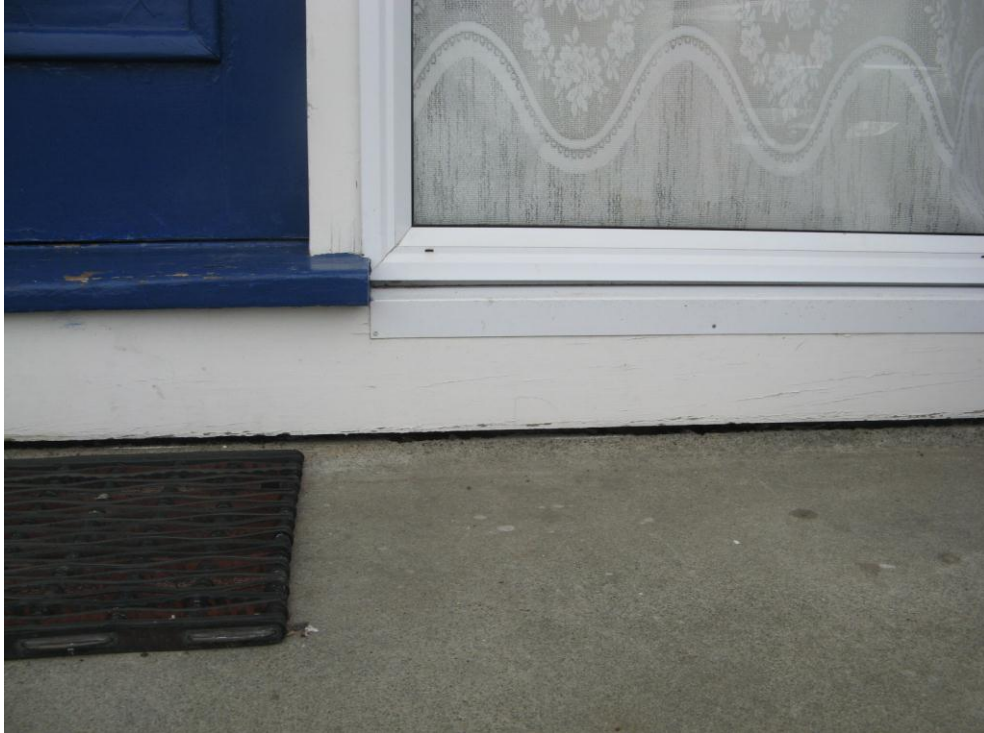
Photo 14: Separation of wall from ground slab at the entrance to unit 6. Shows differential settlement may have occurred.
