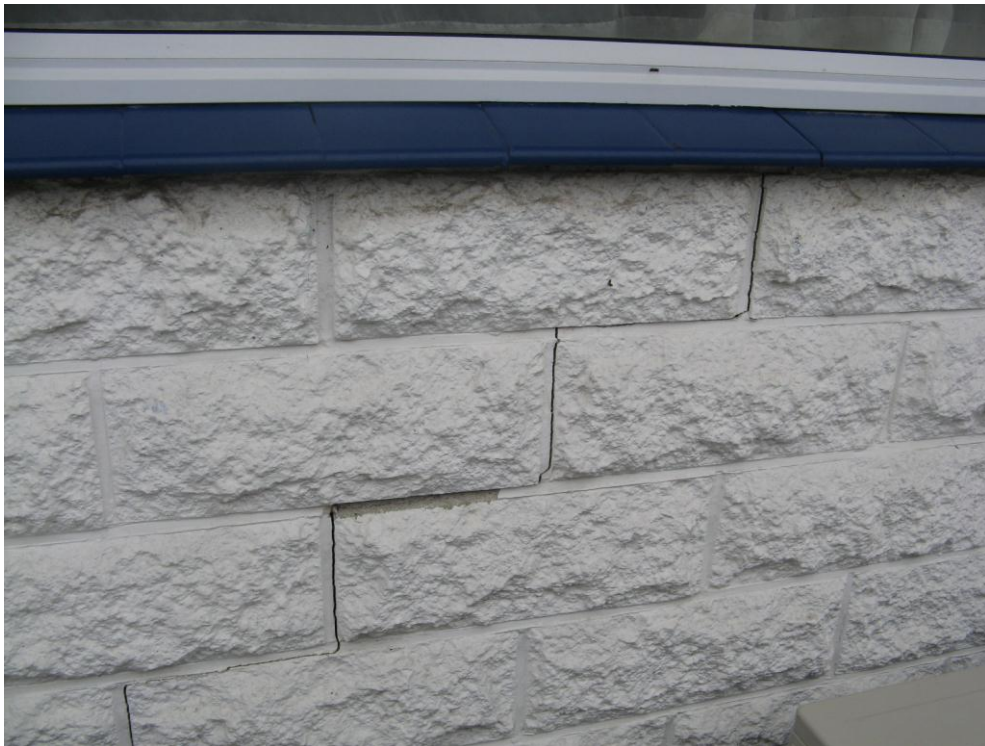
Photo 2: Damage to 90 block wall cladding
