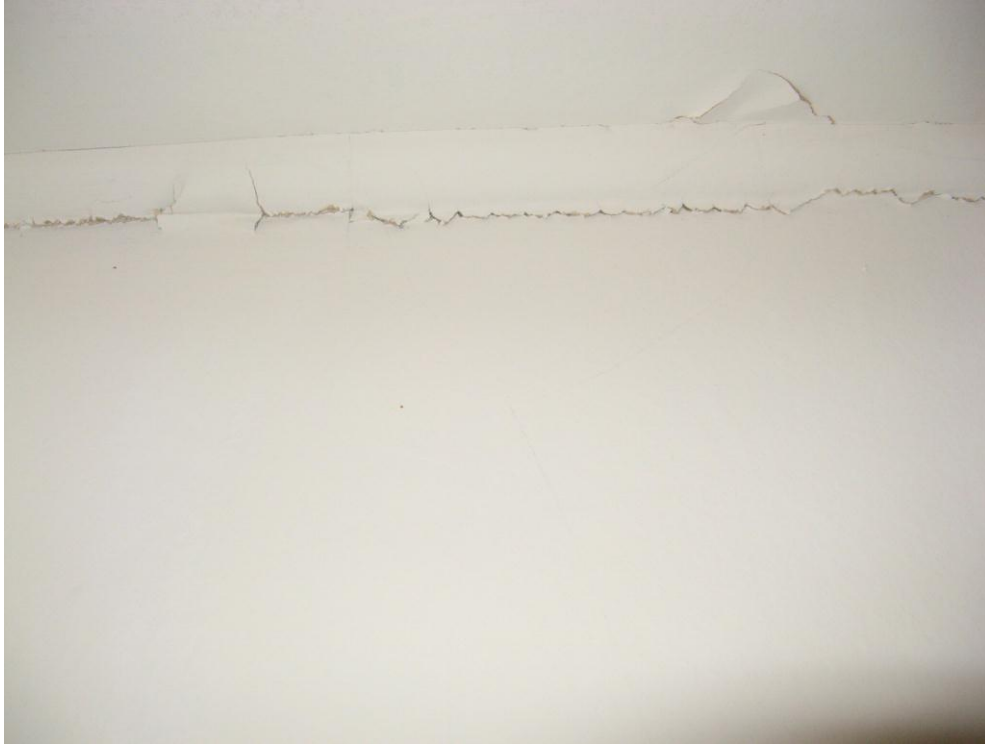
Photo 5: Typical damage at plasterboard ceiling connection to masonry walls.
