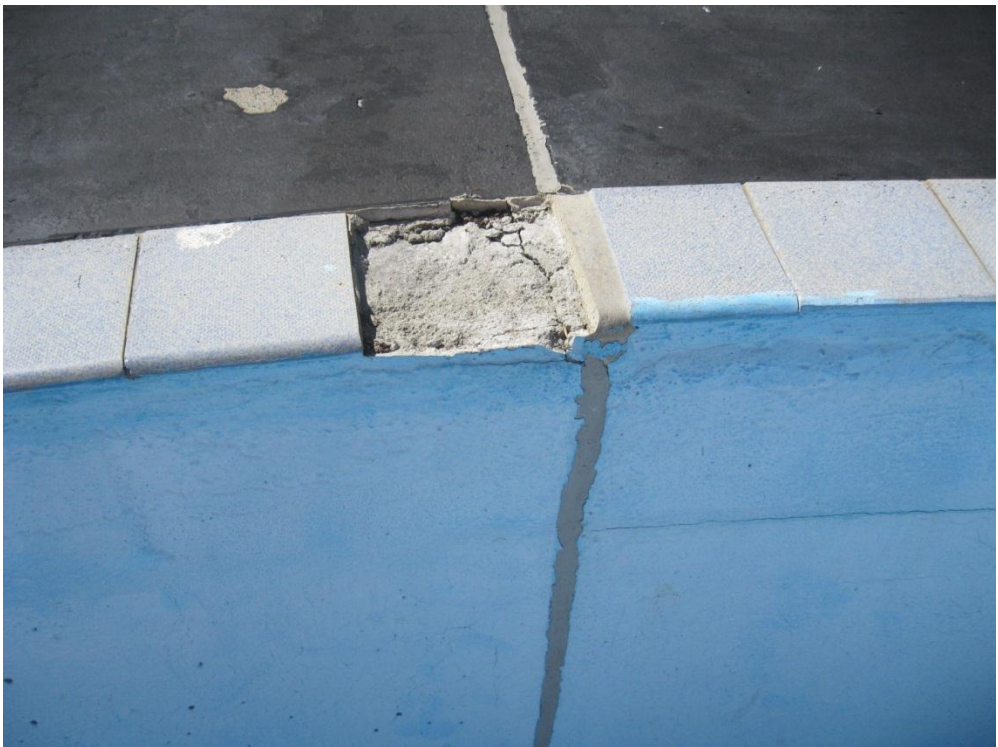
Photograph 4: Damage to tile at top of tank wall.
