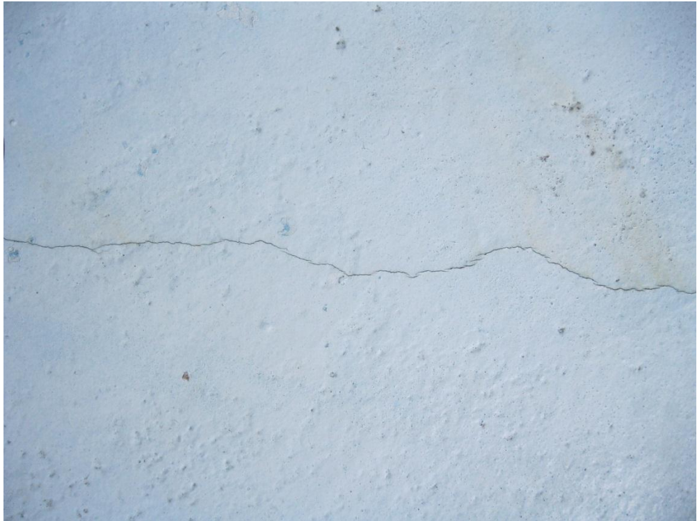
Photograph 7: Shrinkage crack in reinforced concrete tank wall.
