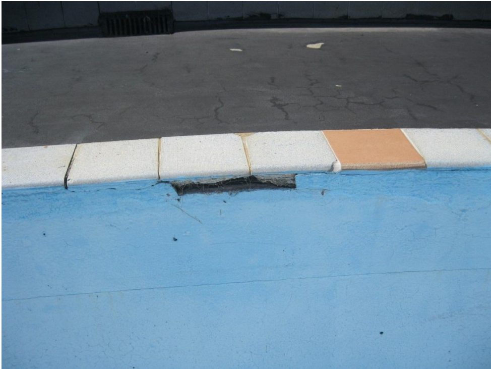
Photograph 5: Damage at top of tank wall.
