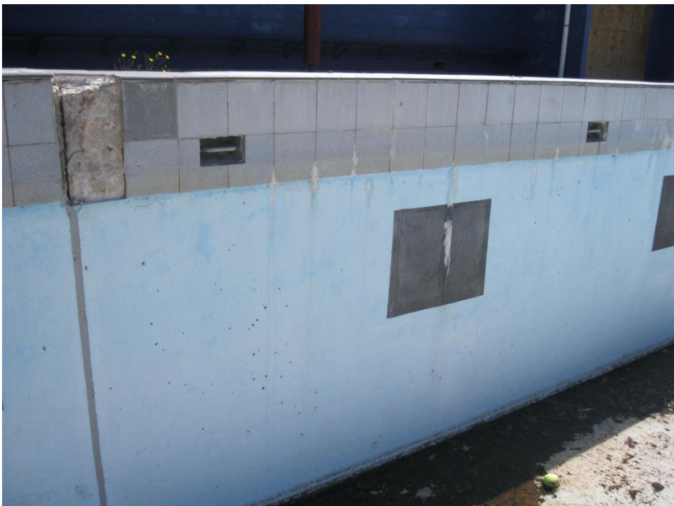
Photograph 6: Damage to mortar surrounding concrete block bund at top of tank wall.
