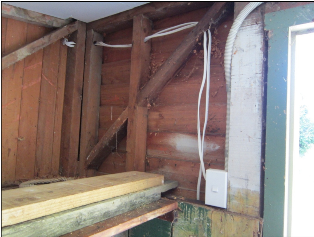
Photo 3: View of a let-in timber brace in the storage room
