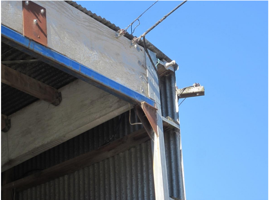
Photograph 7: Top of southern steel frame post. Note steel beam (painted blue) underneath deep timber beam.
