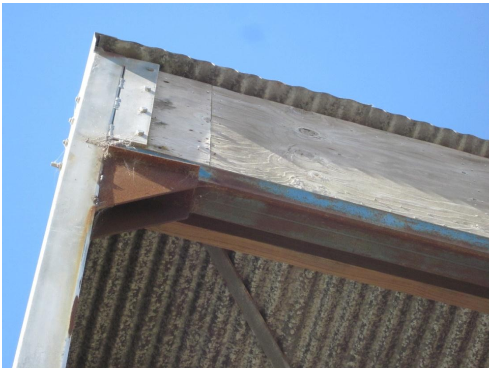
Photograph 6: Top of northern steel frame post at beam connection. Note steel beam (painted blue) underneath deep timber beam.
