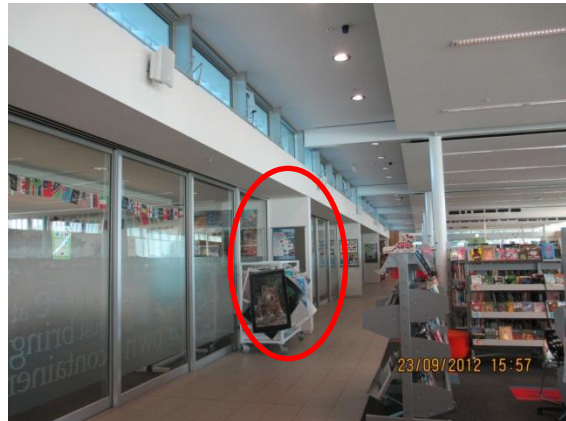
Internal view of the precast concrete tilt up wall panels in the southern end of the building.
