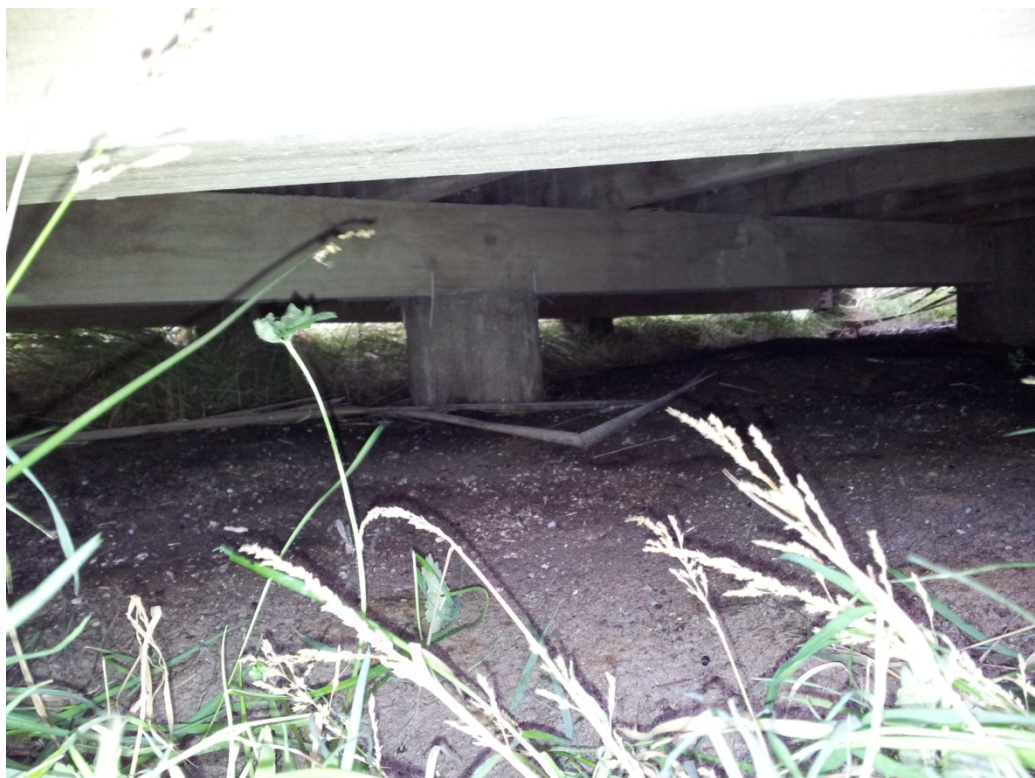
■ Figure 13 – Foundation details of the bird hide
