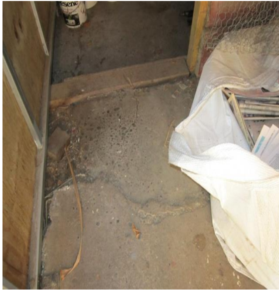
Photo 49: Unlevelled surface of concrete slab inside the barn.
