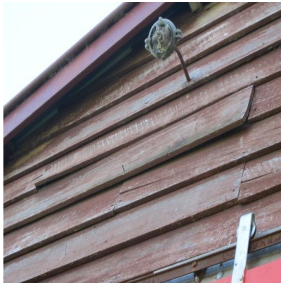
Photo 23: Bowed weatherboards on east timber wall.
