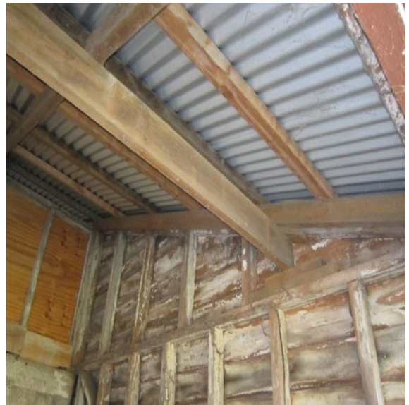
Photo 12: Timber roof rafters at 600mm spacing and external timber wall with 150x50mm posts at 600mm spacing.
