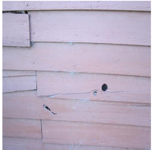
Photo 16: Cracking to timber weatherboards on east wall.
