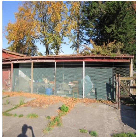
Photo 22: West section of building with three equally spaced steel hollow section posts.
