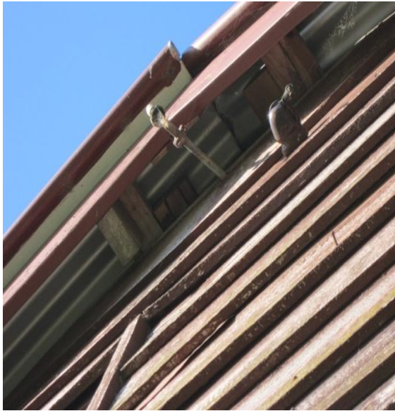
Photo 41: Soffit on west side with exposed corrugated roof sheeting and timber roof rafters.
