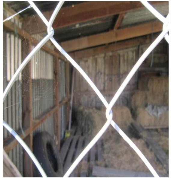
Photo 34: Internal layout of north extension showing corrugated metal external walls with timber posts and internal timber walls.
