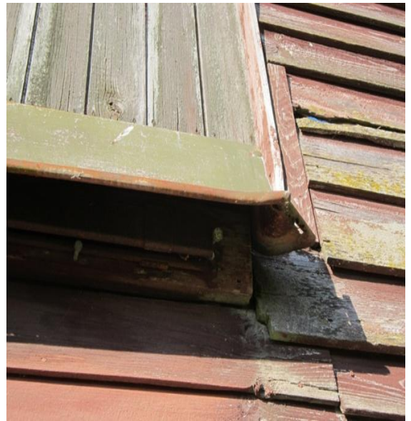
Photo 38: Rusted roller door elements on west wall.
