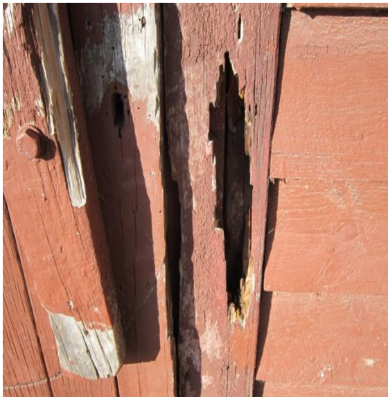
Photo 43: Existing damage to timber members on west wall.
