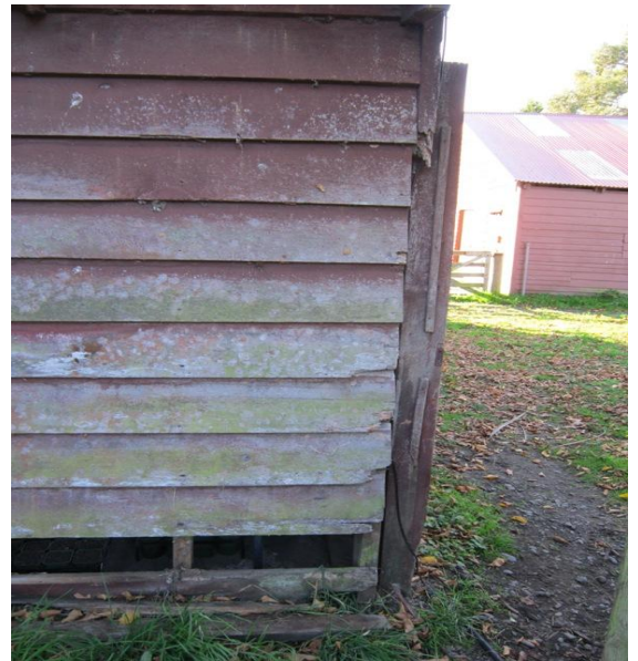
Photo 30: Missing weatherboard on south side of south lean-to.
