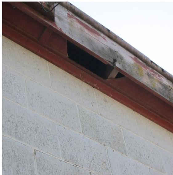
Photo 27: Soffit element missing on north side.
