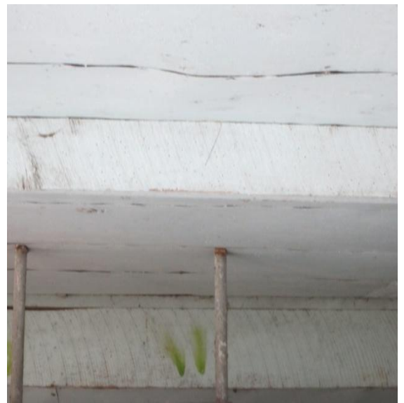
Photo 24: Internal steel hollow section props in the west section.
