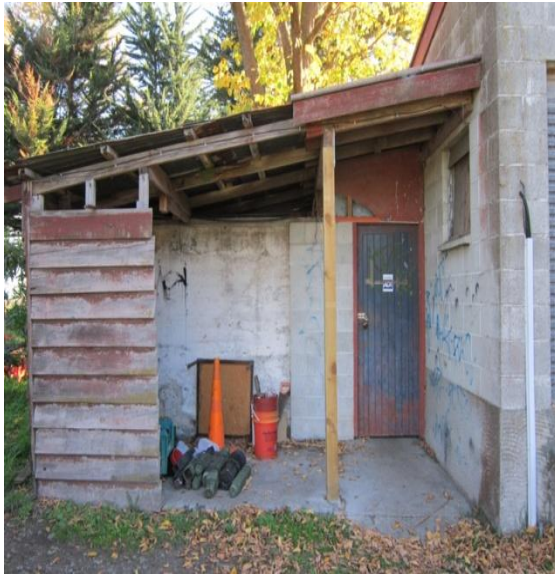
Photo 9: Lean-to on the south of the building with a timber-framed roof and corrugated metal roof.
