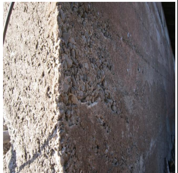
Photo 40: Large aggregate sizes in concrete wall on southwest corner.
