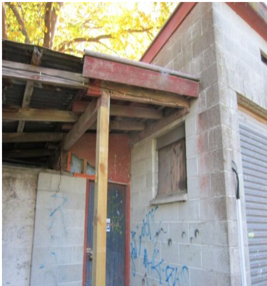
Photo 11: Lean-to on the south of the building with a timber-framed roof and corrugated metal roof.
