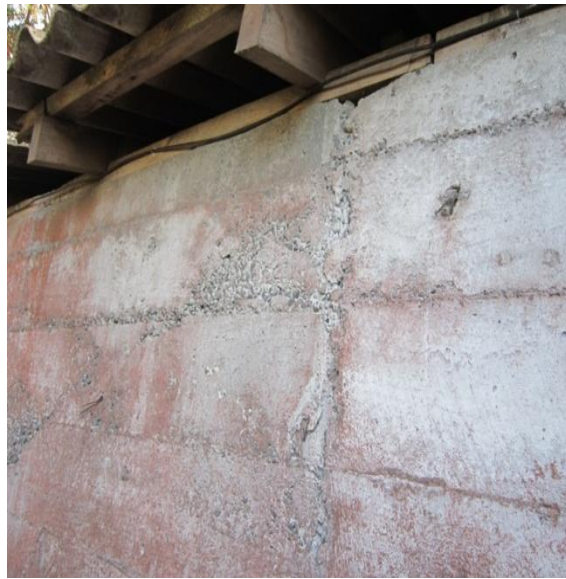
Photo 37: Spalling of south concrete wall due to large aggregate sizes. Timber roof elements also shown.
