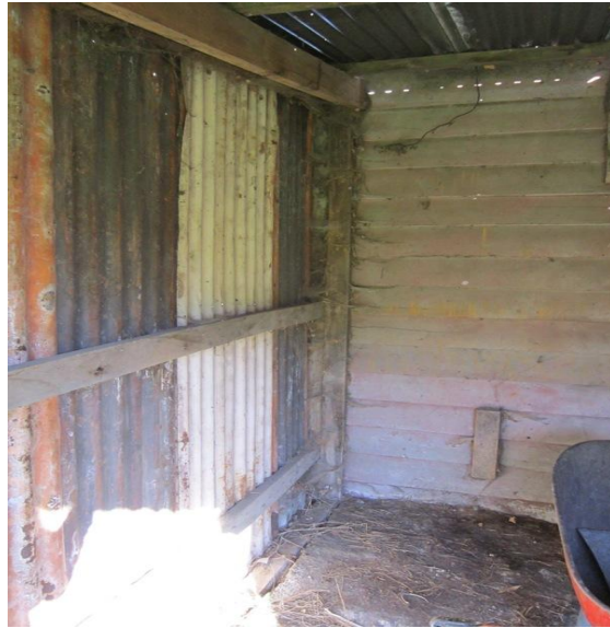
Photo 29: External corrugated metal and timber wall members of north extension.
