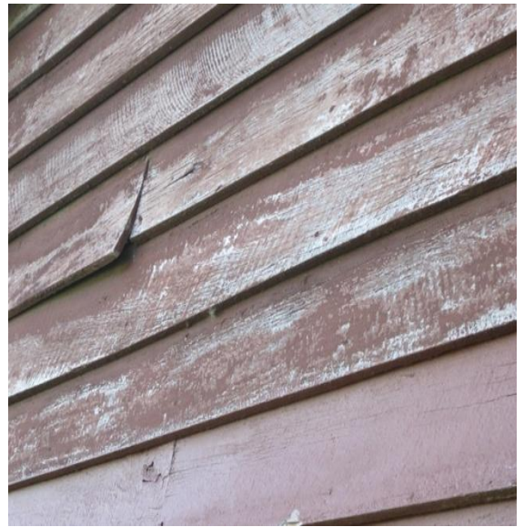
Photo 18: Bowed weatherboards on east timber wall.
