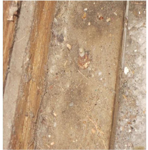
Photo 54: Timber wall base anchored into concrete slab.
