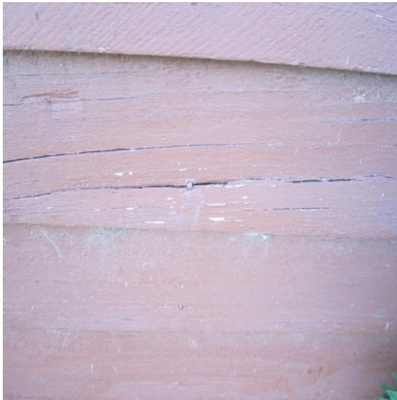
Photo 15: Cracking to timber weatherboards on east wall.
