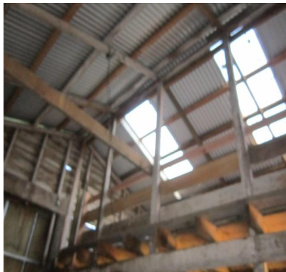
Photo 59: Exposed corrugated roof sheeting and timber roof rafters, with internal timber beams and columns shown providing support to the roof elements.
