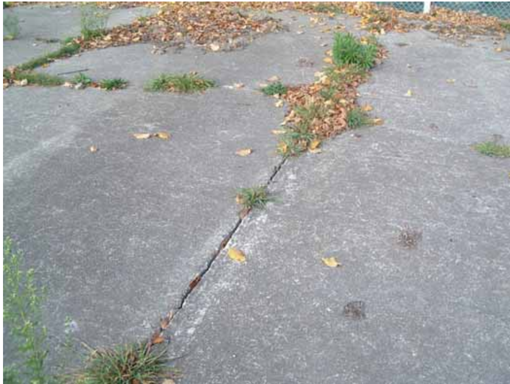
■ Figure 16 - Noted damage to the concrete paving
