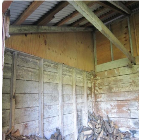
Photo 10: Internal timber walls with 150x50mm posts at 600mm spacing.
