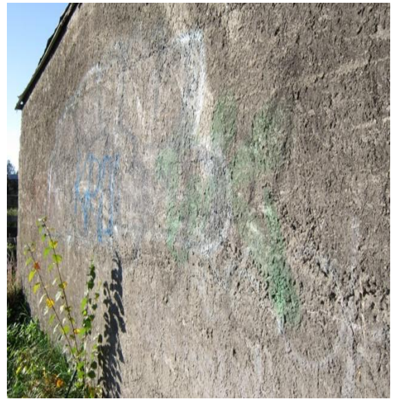
Photo 42: Large aggregate sizes in west concrete wall.
