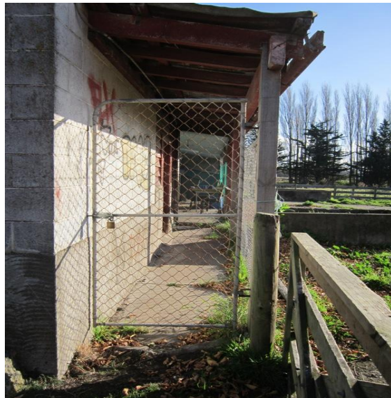
Photo 21: East masonry section of north wall with extended lightweight roof.
