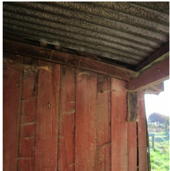
Photo 32: Internal timber wall of north extension with corrugated metal roof.
