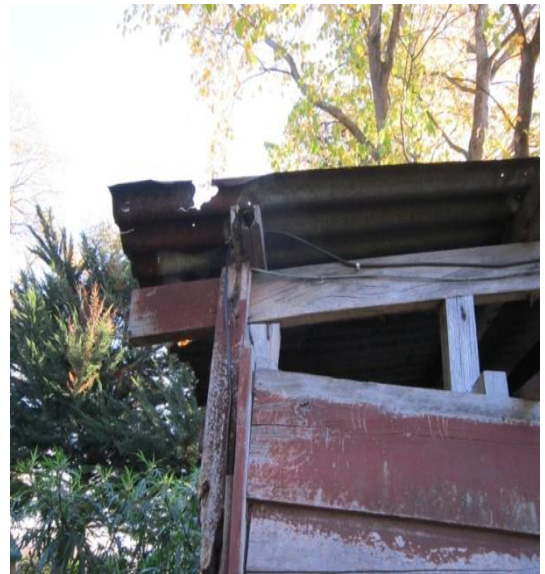
Photo 12: Lean-to on the south of the building with corroded metal roof sheeting.
