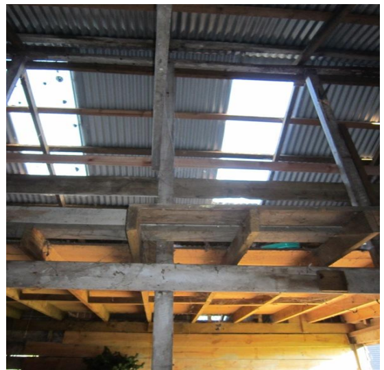
Photo 60: Exposed corrugated roof sheeting and timber roof rafters, with internal timber beams and columns shown providing support to the roof elements, by raised platform.
