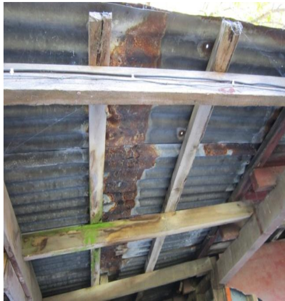
Photo 29: Rusted corrugated roof sheeting on south lean-to.
