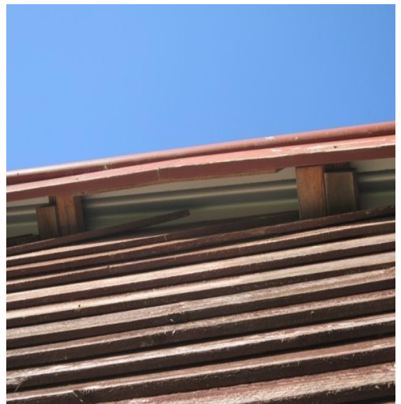
Photo 40: Soffit on west side with exposed corrugated roof sheeting and timber roof rafters.
