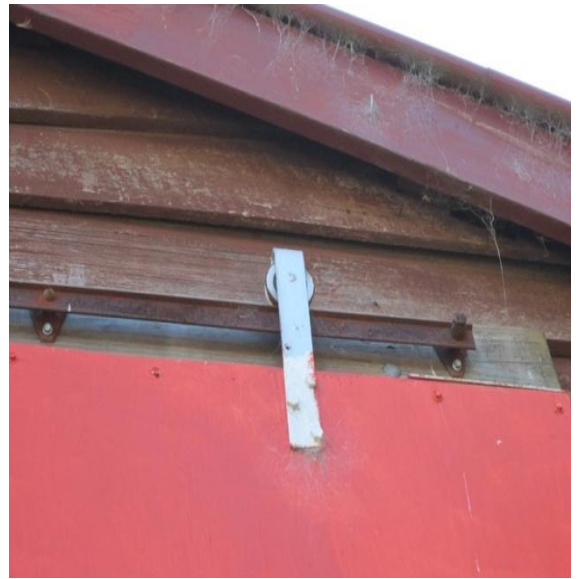
Photo 22: Rusted steel elements of building.
