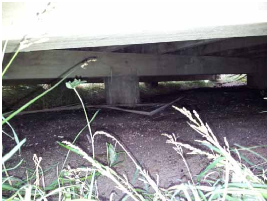
■ Figure 13 – Foundation details of the bird hide
