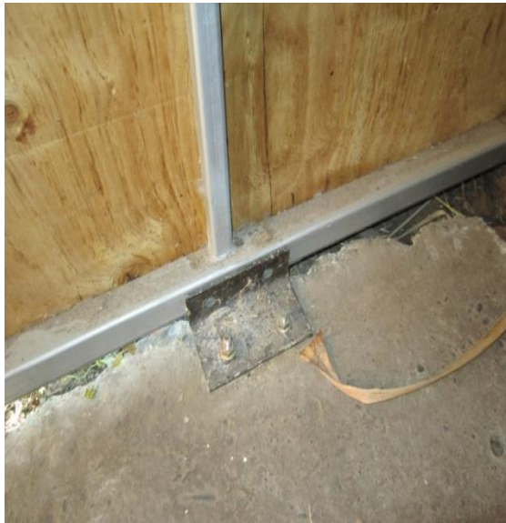
Photo 51: Anchors in concrete slab in west roller door support.
