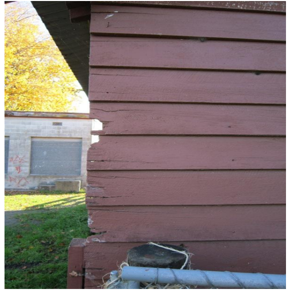
Photo 14: Existing impact damage to timber weatherboards on southeast corner.
