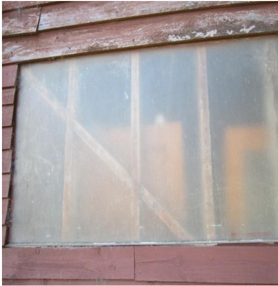
Photo 25: Window on east wall showing diagonal timber bracing member.
