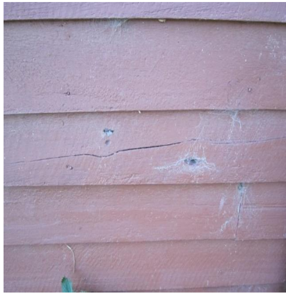
Photo 17: Cracking to timber weatherboards on east wall.
