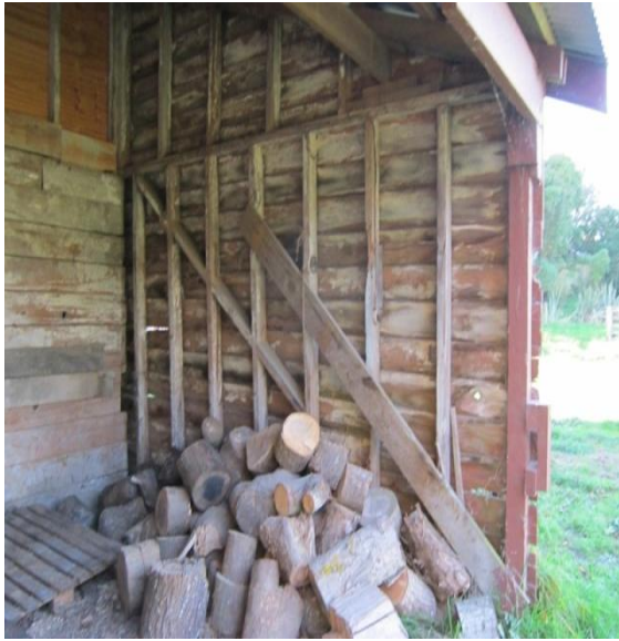
Photo 13: Timber wall in southeast corner of building with timber diagonal bracing.
