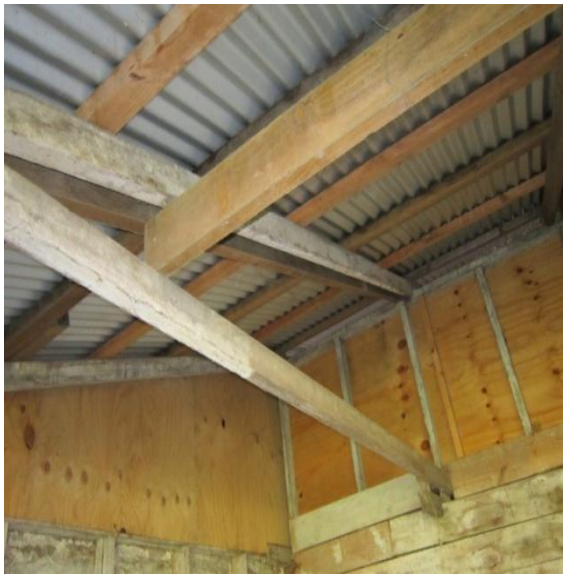
Photo 11: Timber roof rafters at 600mm spacing.
