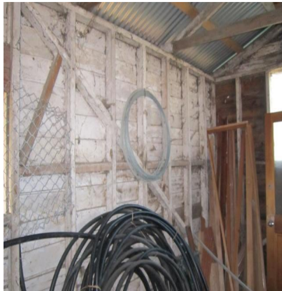
Photo 57: Diagonal timber wall brace on internal wall shown.
