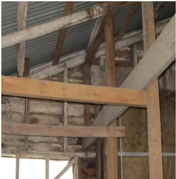
Photo 55: Exposed corrugated roof sheeting with timber roof rafters. Internal timber beams and columns also shown.
