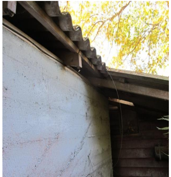
Photo 36: South concrete wall of west section, with timber roof rafters shown under corrugated roof sheeting.
