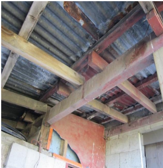
Photo 15: Lean-to on the south of the building with a timber-framed roof and rusted corrugated metal roof.
