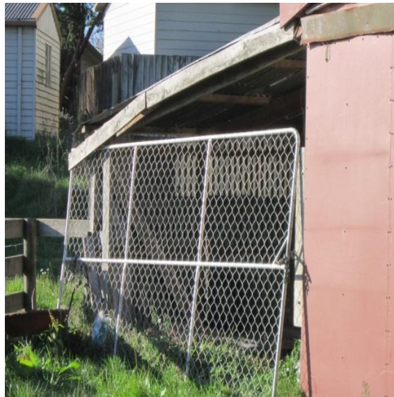
Photo 45: Displaced timber roof beam over west entrance to northern extension.
