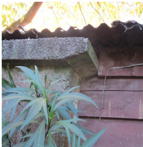
Photo 31: South timber wall joins with south concrete wall.
