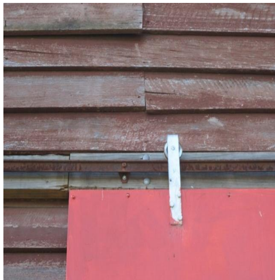
Photo 19: Bowed weatherboards on east timber wall and roller door entrance to building.
