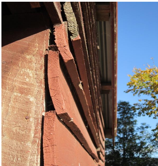
Photo 39: Bowed weatherboards on west wall.
