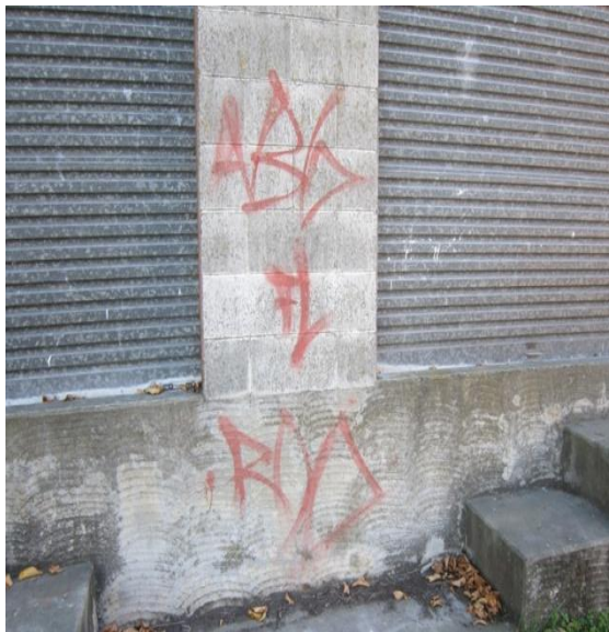
Photo 19: East masonry wall with two garage doors and concrete strip footing.
