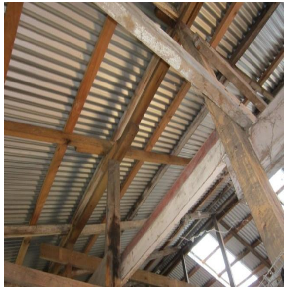
Photo 58: Exposed corrugated roof sheeting and timber roof rafters, with internal timber beams and columns shown providing support to the roof elements.
