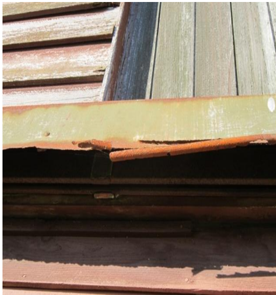
Photo 37: Rusted roller door elements on west wall.
