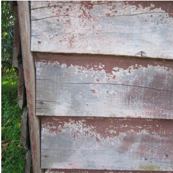
Photo 13: Cracking in timber weatherboards on south lean-to.
