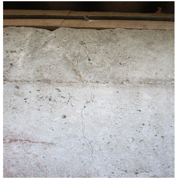
Photo 38: Vertical hairline crack on south concrete wall.
