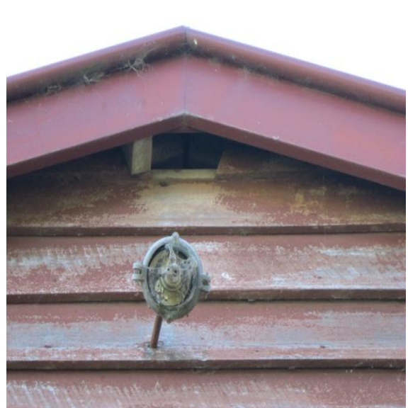
Photo 20: Missing weatherboards at roof apex on east wall.
