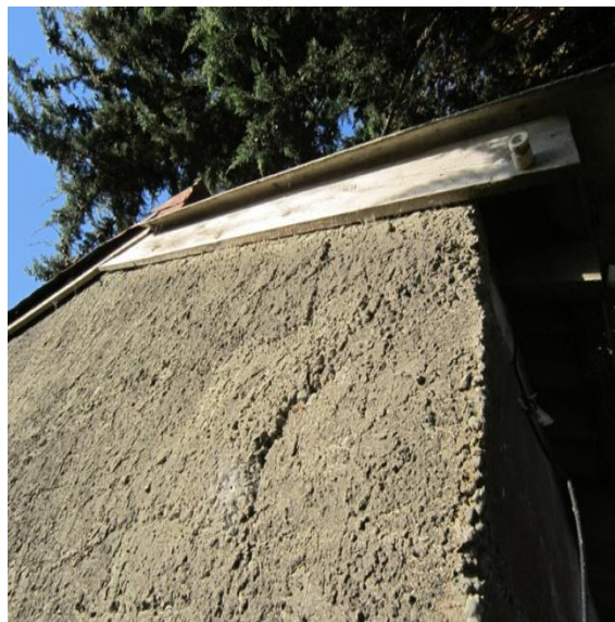
Photo 39: Large aggregate sizes in west concrete wall.
