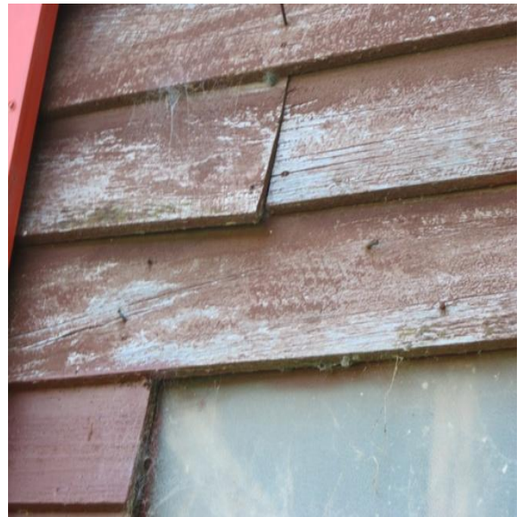
Photo 24: Bowed weatherboards on east timber wall.
