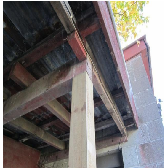
Photo 14: Timber column on east side of lean-to.
