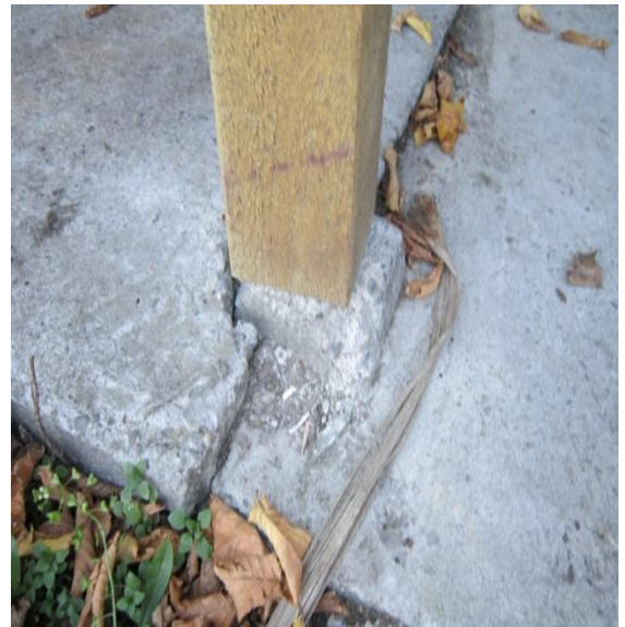
Photo 16: Base of timber column on east side appears to have no fixed shear connection to the concrete ground slab.
