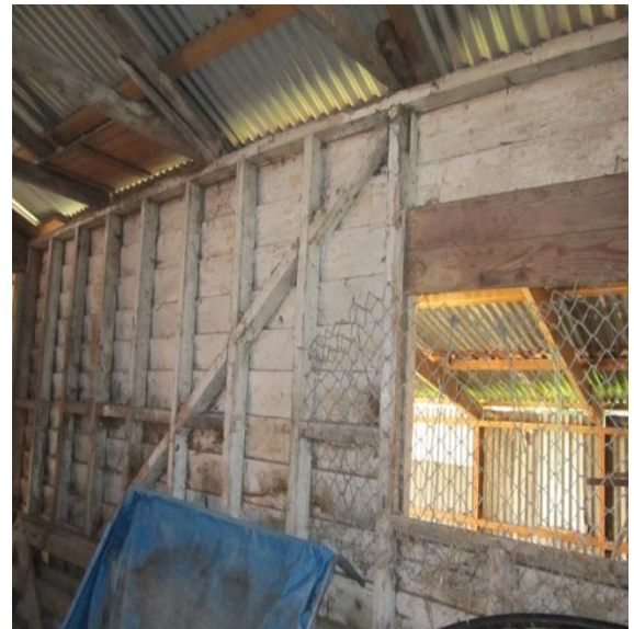
Photo 56: Diagonal timber wall brace on internal wall shown.
