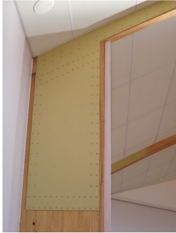
Close up of the glulam portal frame knee joint.
