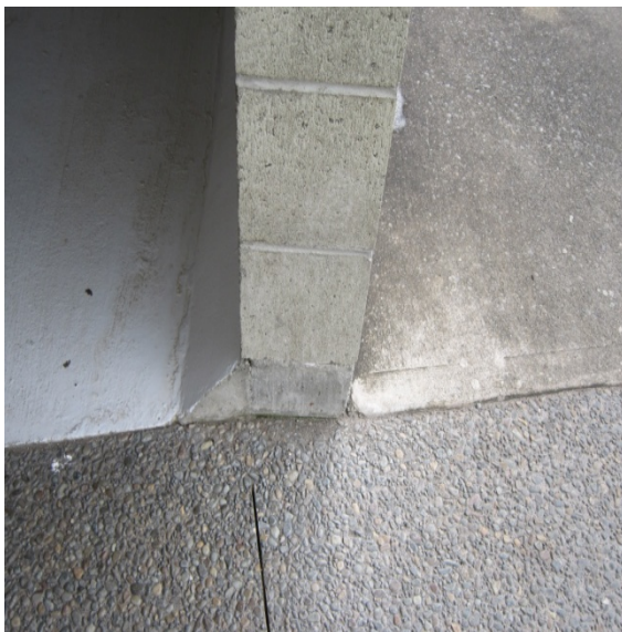
Photo 7: Footpath cast up to foundations with a concrete slab on grade cast within the structure
