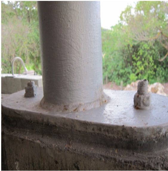
Photo 5: Base plate for roof support columns
