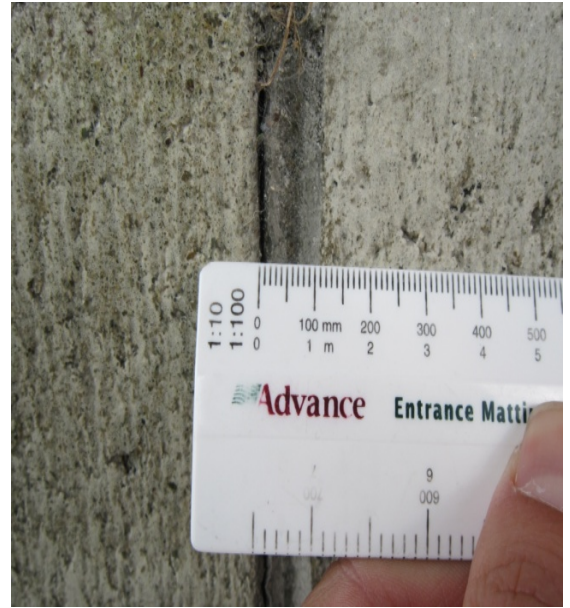
Photo 10: Cracking of approximately 1mm on north east corner
