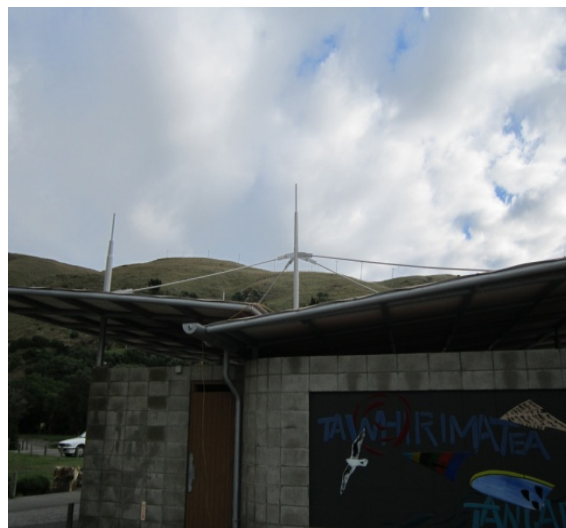
Photo 2: Structure consists of steel framed roof support by masonry shear walls via CHS columns
