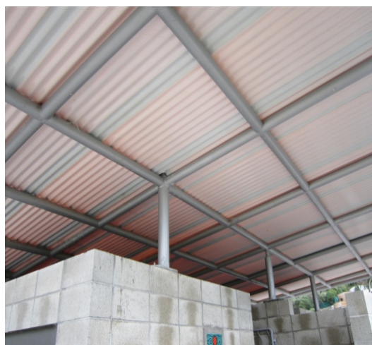
Photo 3: View along east support lines. Roof supports along west, centre and east lines with three supports per line, corner four supports also connected to central mast as shown in photo 3.
