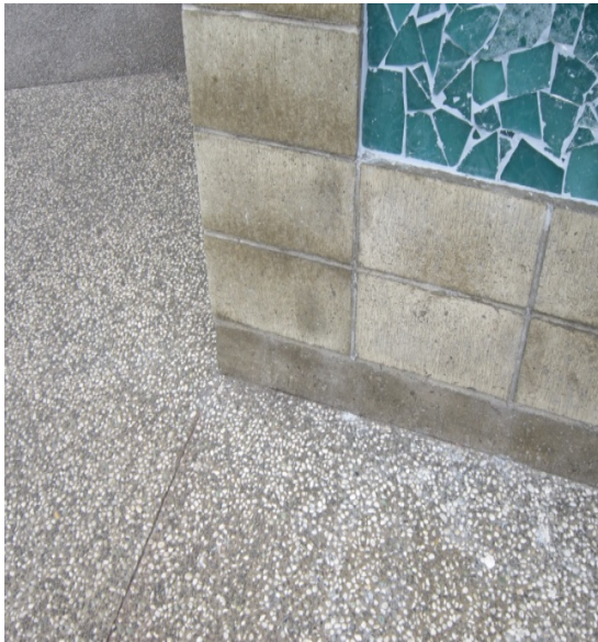
Photo 13: Corner of masonry structural walls
