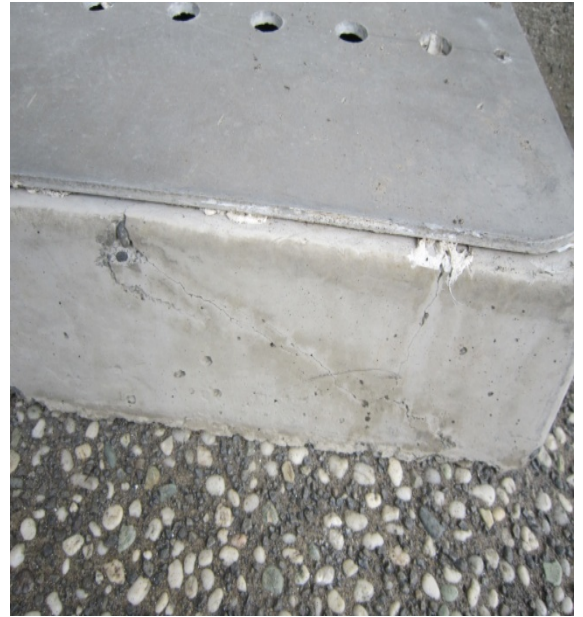
Photo 18: Hairline cracking through drainage pit.
