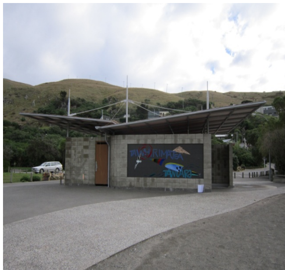
Photo 1: Taylors Mistake Bay toilets and changing rooms
