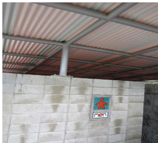
Photo 4: Support columns bolted to top of masonry walls via a base plate.
