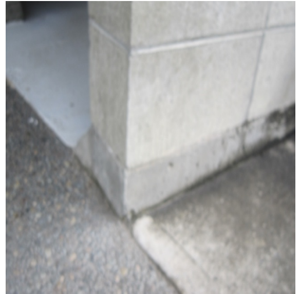
Photo 6: Concrete strip foundations supporting the masonry shear walls
