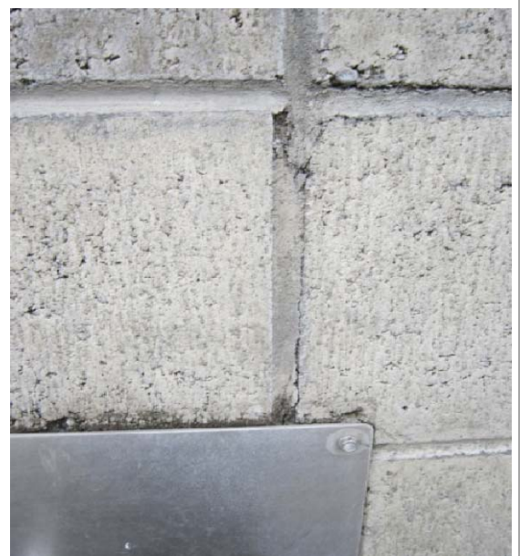
Photo 12: Separation of stacked masonry along mortar joint of approximately 0.4mm
