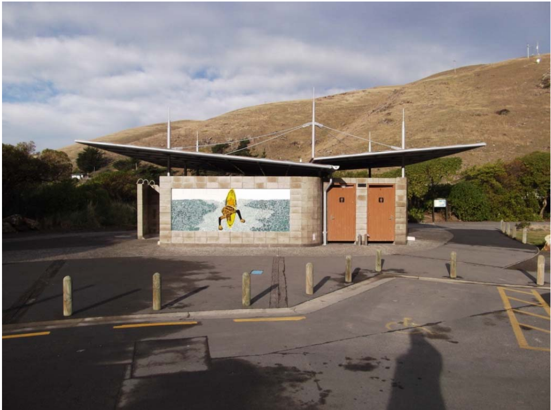
■ Figure 5 - Overview of the building (northwest wall).
