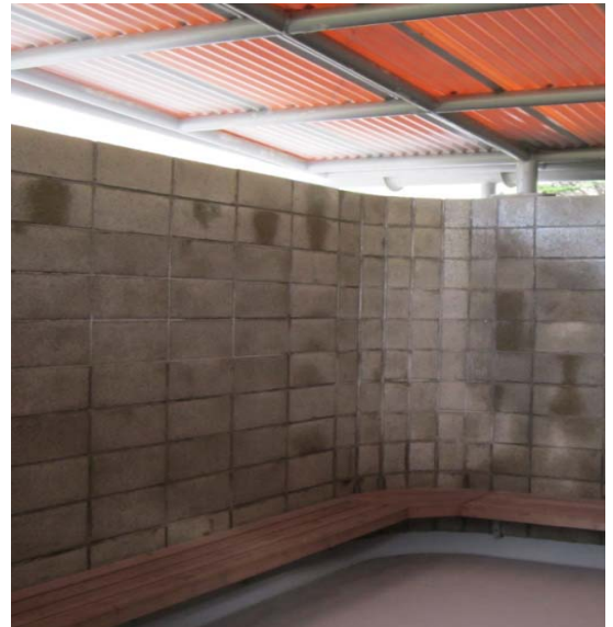
Photo 8: Typical corner detail with short blocks used to create a curve. Note blocks are stacked as opposed to staggered.
