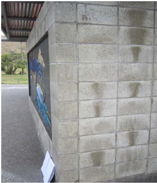
Photo 9: Separation of masonry along the mortar joint
