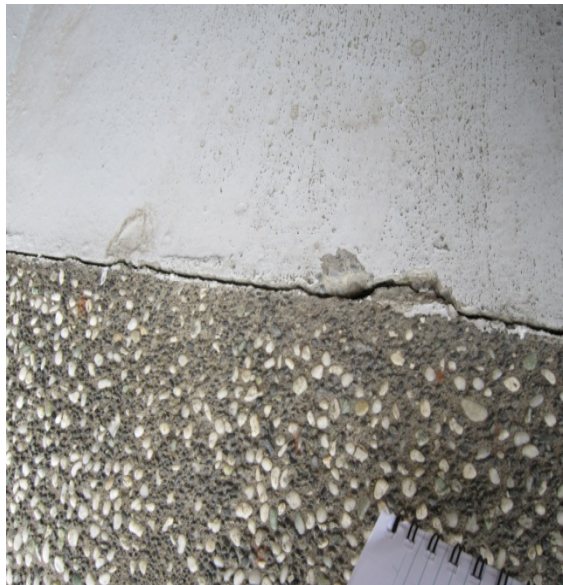
Photo 15: Separation of floor slabs from surrounding footpaths
