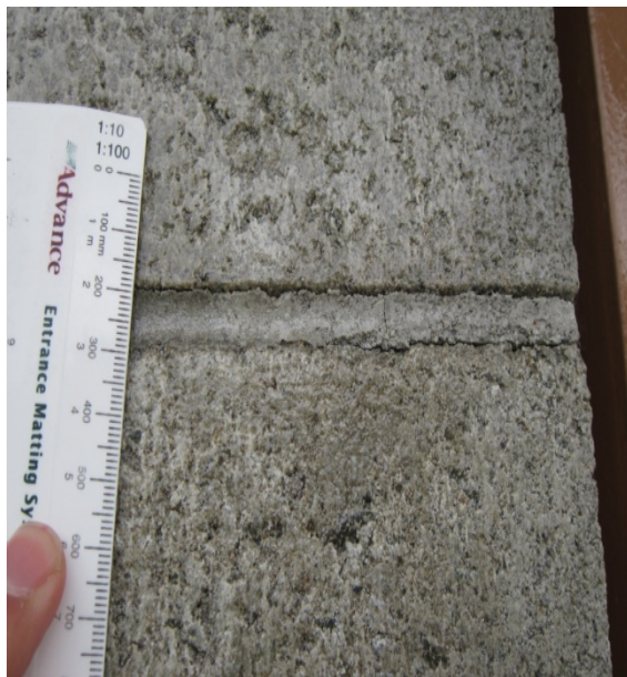
Photo 11: Separation of masonry along mortar joint approximately 0.3mm
