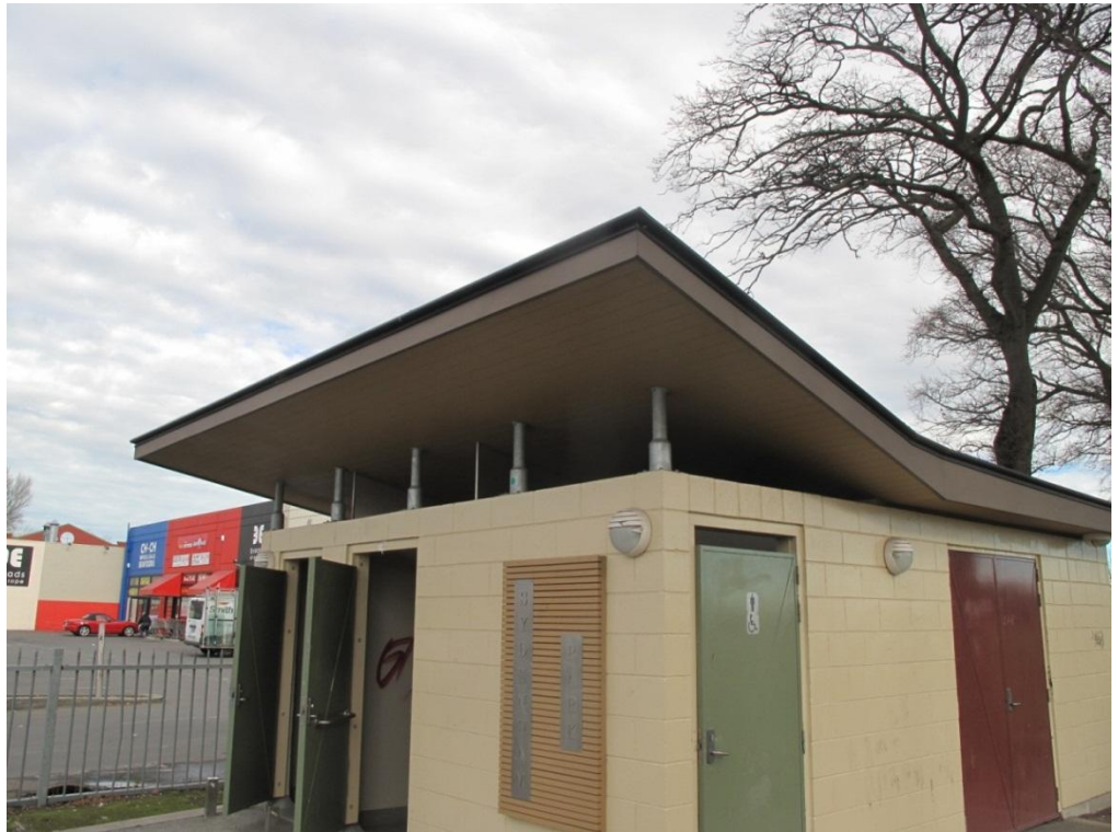
Photograph 7 Raised roof structure on the eastern side of the toilet block.
