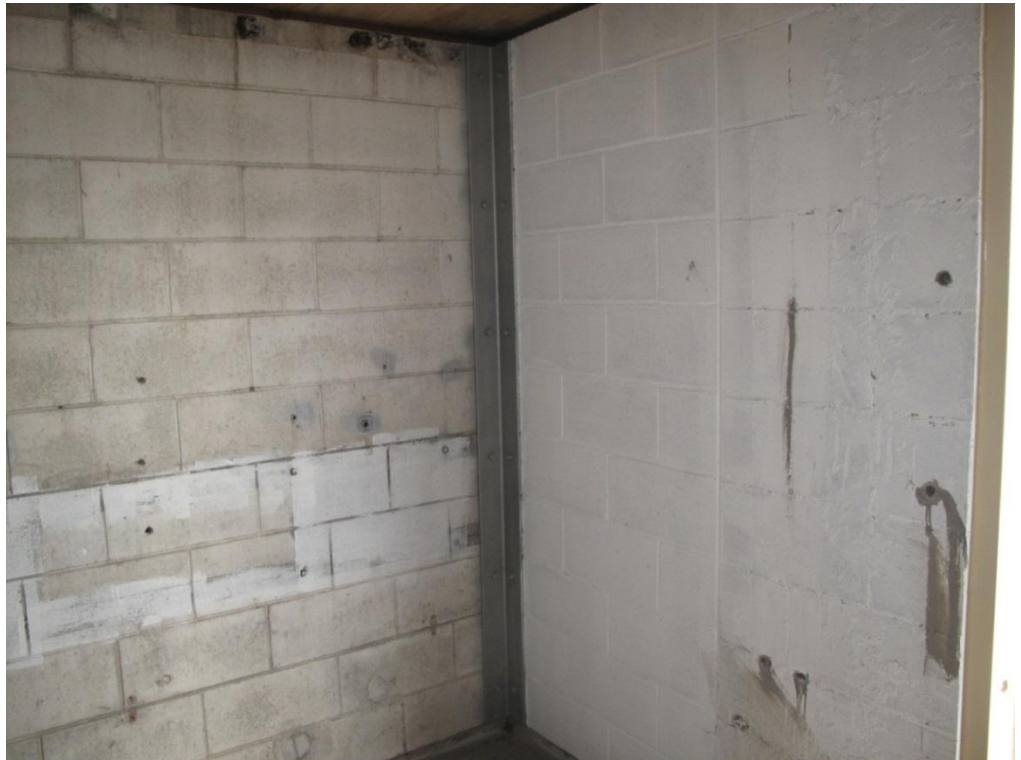
Photograph 5 Steel angle bolted to north west corner of the toilet block.
