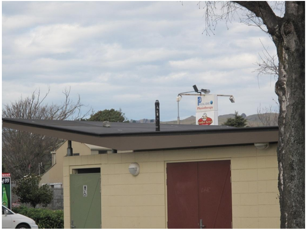
Photograph 9 Middle and western sections of the roof rest directly on the concrete block walls.
