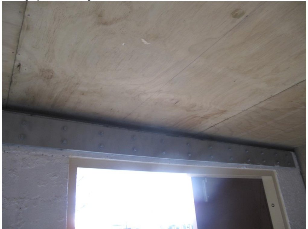
Photograph 6 Steel angle bolted to north west corner of the toilet block.
