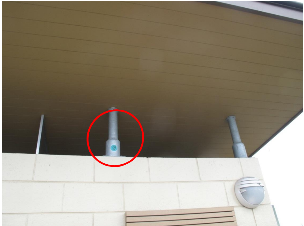
Photograph 8 Steel posts supporting roof beams on the eastern side of the structure.
