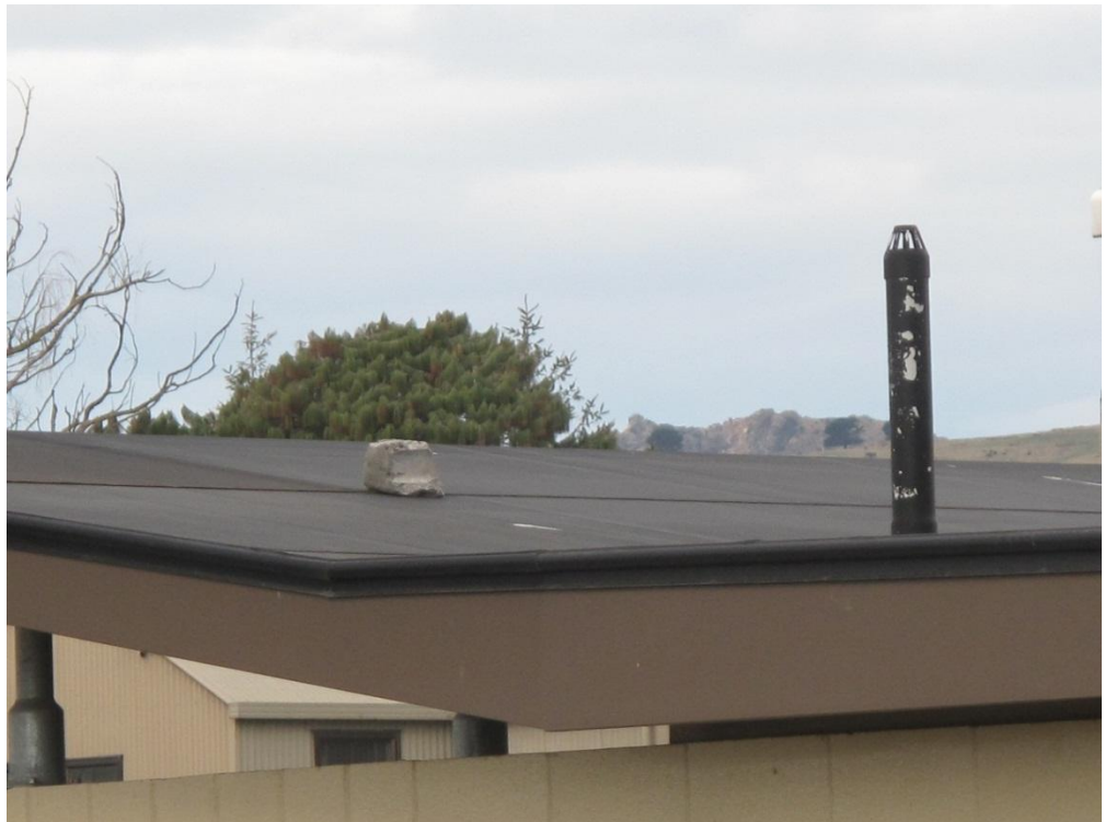
Photograph 10 The roof appears to be covered with asphalt sheets.
