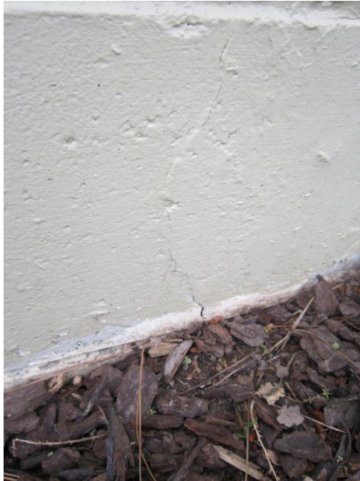
Photo 13: close up view from photo 11 showing 1mm cracks at foundation
