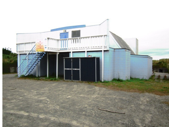
Western elevation of the Spencer Park Surf Club.
