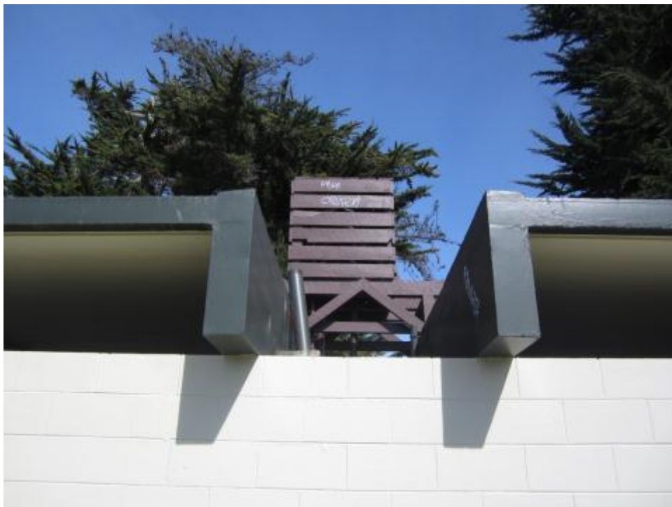
Photograph 6 Reinforced concrete legs supporting the reinforced concrete roof slab
