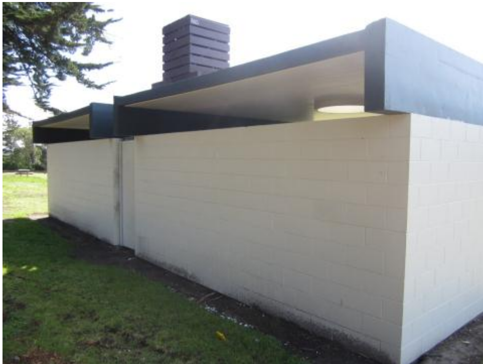
Photograph 2 View of concrete masonry wall and reinforced concrete roof slab
