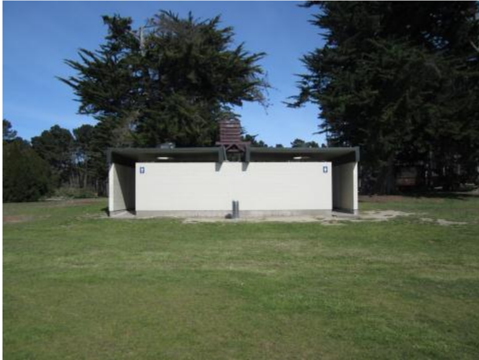
Photograph 3 View of the building from the north-east
