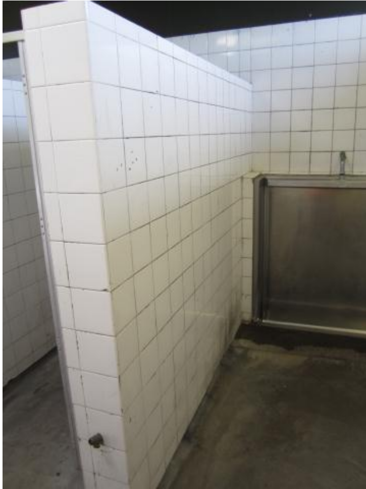
Photograph 5 Internal concrete masonry partition walls clad with ceramic tiles
