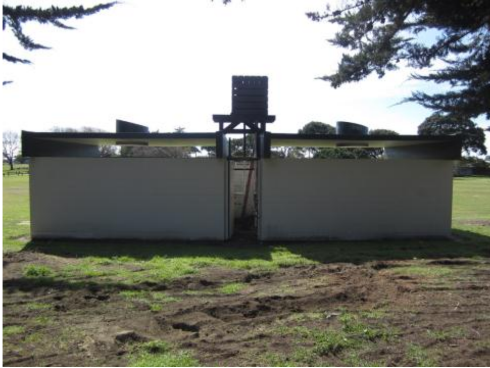
Photograph 1 View of the building from the south-west
