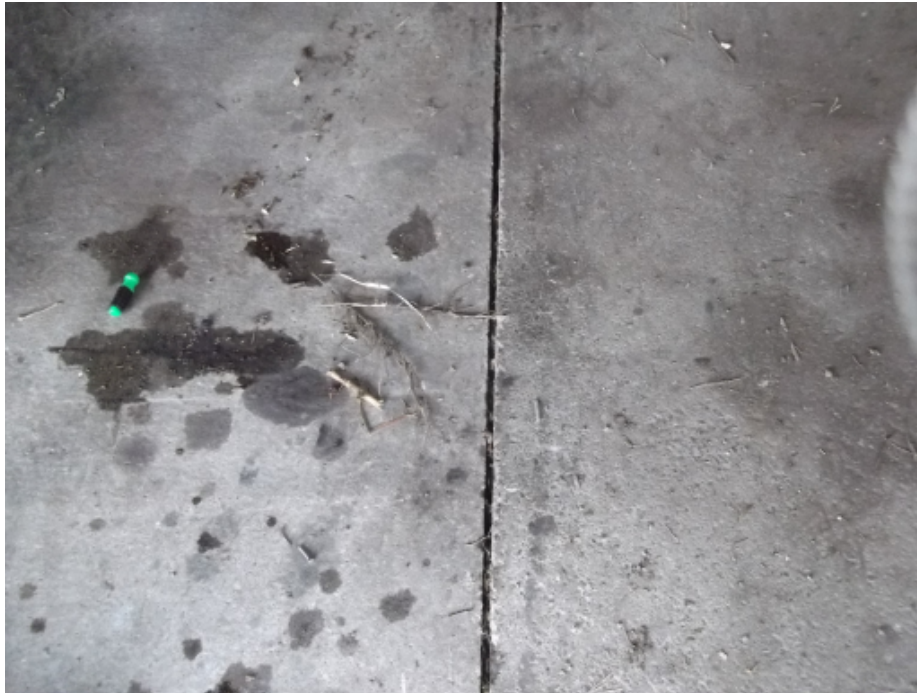
Photo 7: Widened construction joint
