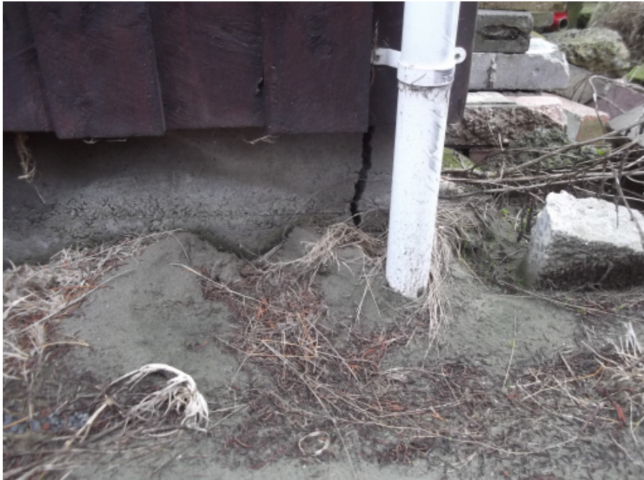
Photo 5: Cracking to foundation
