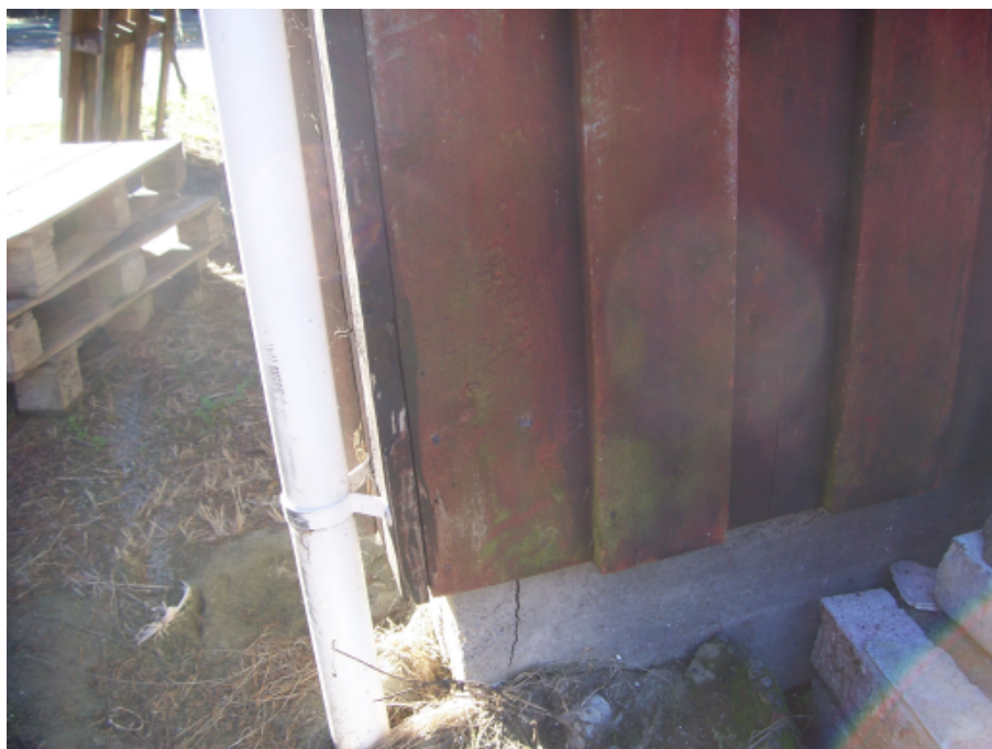
Photo 6: Cracking to foundation
