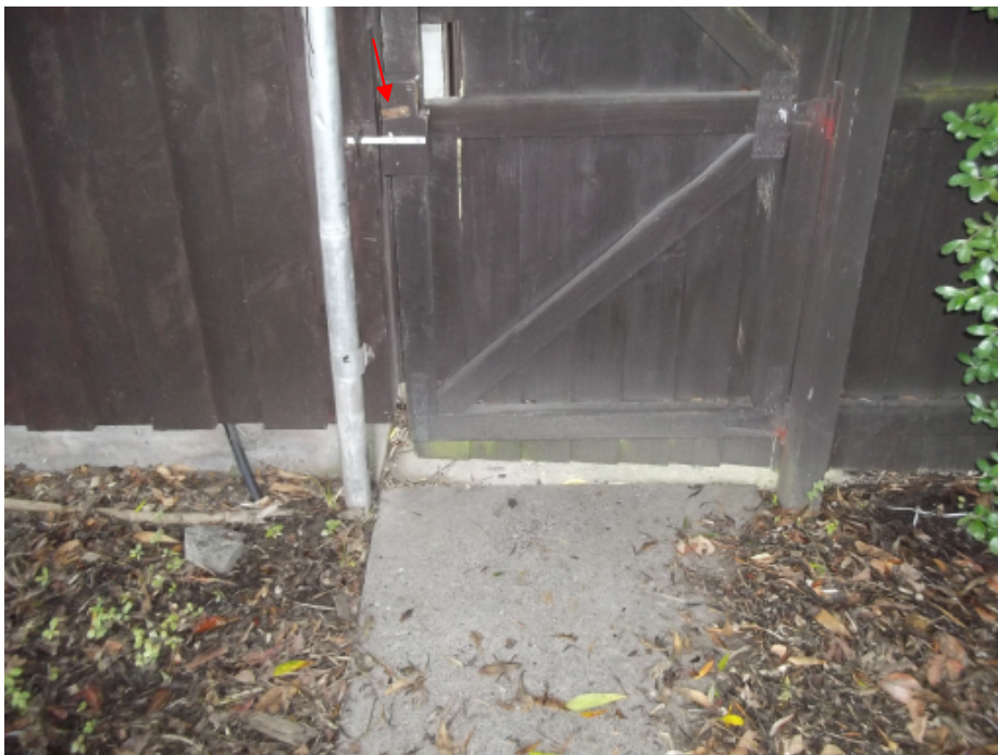
Photo 8: Ground movement indication
