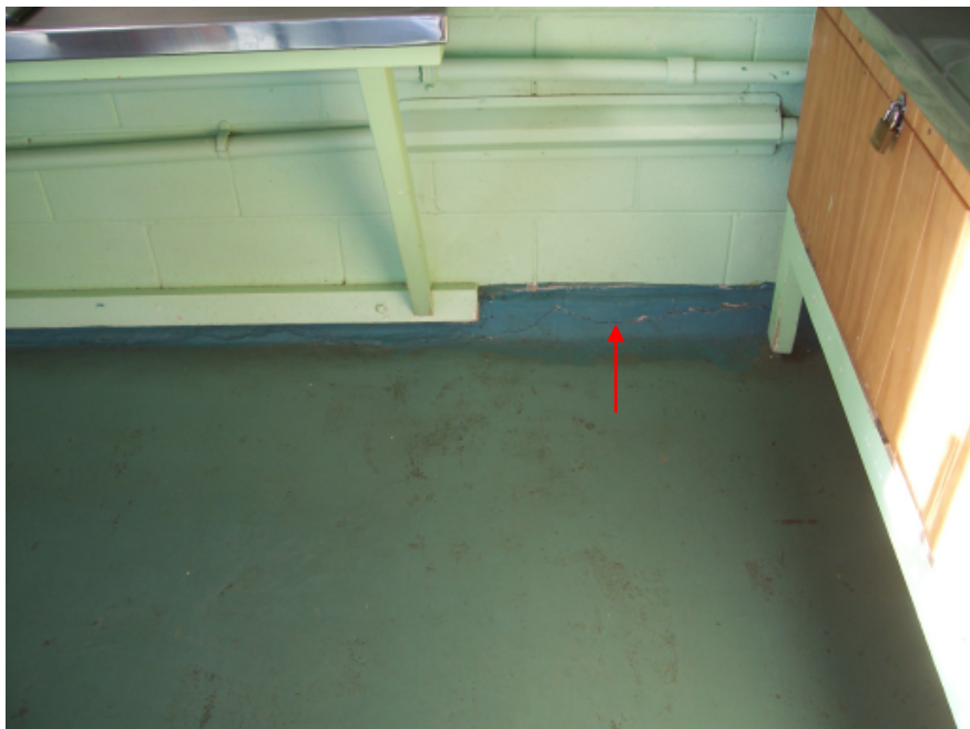
Photo 2: Typical cracking to thickened slab and separation between internal wall and thickened slab
