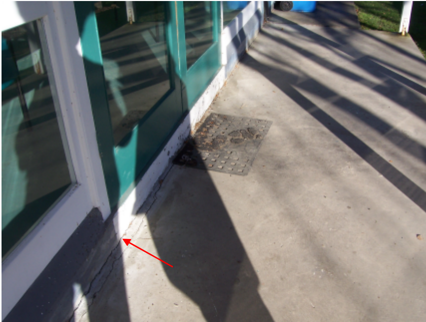
Photo 1: Typical Cracking and separation between slab edge thickening and external concrete apron
