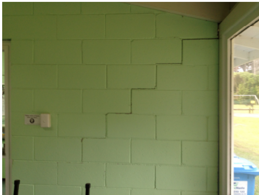
Photo 4: The widest cracking to masonry block
