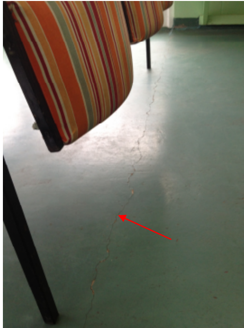
Photo 5: Typical cracking to concrete slab
