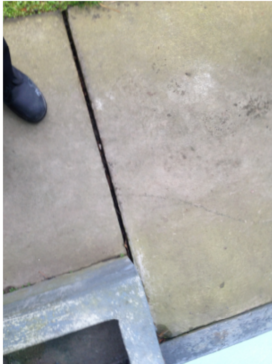
Photo 3: Widened construction joint of external concrete apron
