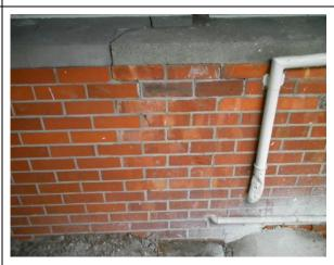
Step in floor slab between original slab and new slab.
