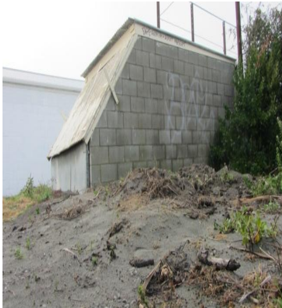
Photo 5: View showing evidence of liquefaction near the shed
