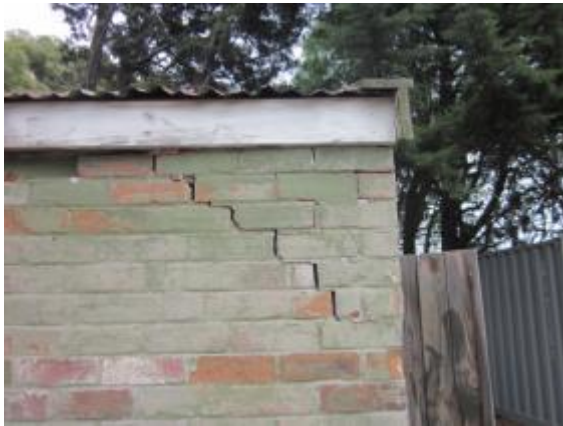
Photo 5: Major Cracking to Masonry in NW Corner
