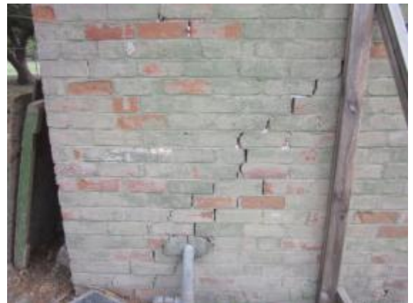
Photo 8: Major Cracking to Masonry in NE Corner
