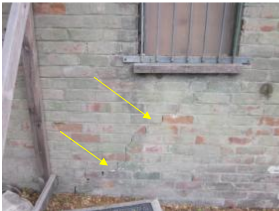
Photo 7: Step Cracking to Masonry on the North Face
