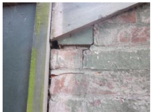
Photo 10: Minor Cracking around top Brick in the SE Corner
