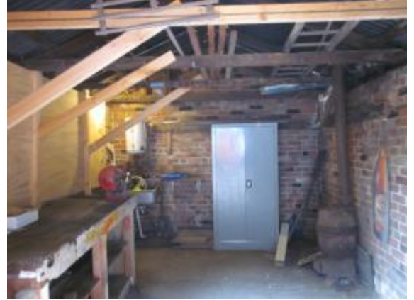
Photo 2: Internal View of Tool Shed - Temporary Proping Installed along North Face
