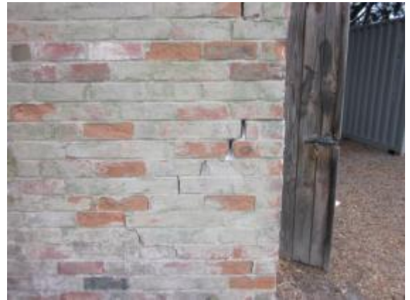
Photo 6: Major Cracking to Masonry in NW Corner
