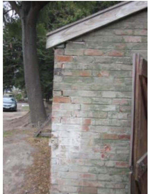
Photo 12: Cracking to Masonry in NW Corner
