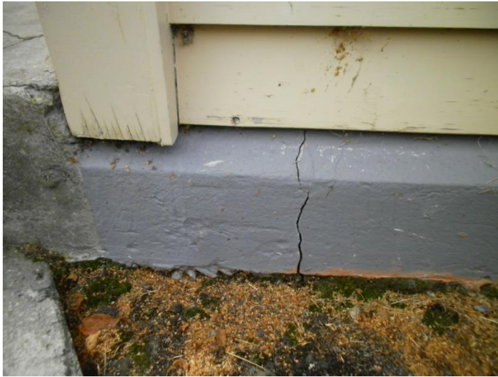
Crack in concrete perimeter foundation
