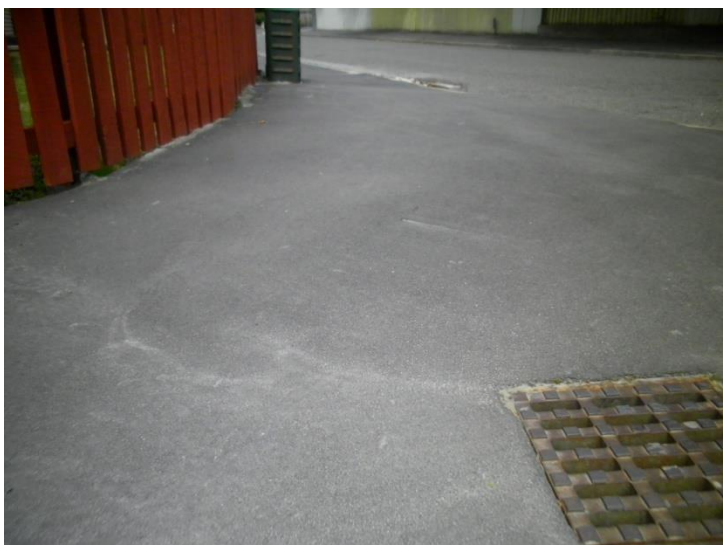
Sizable liquefaction boil below asphalt
