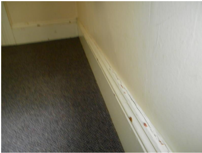
Lining damage at floor level
