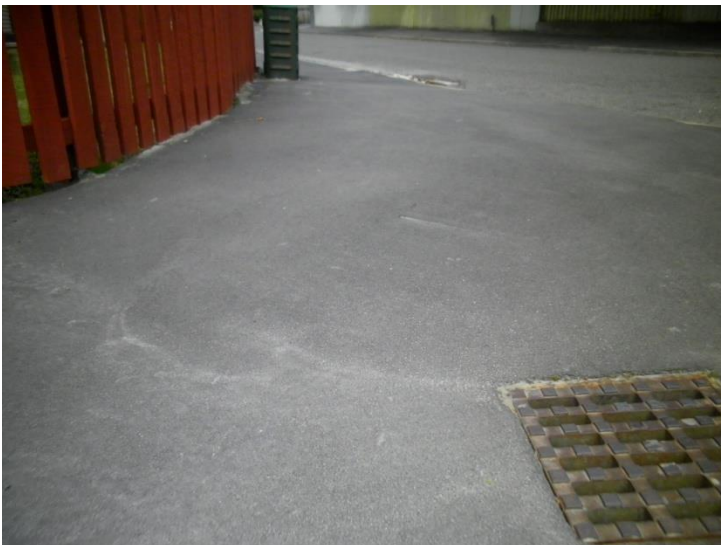
Sizable liquefaction boil below asphalt
