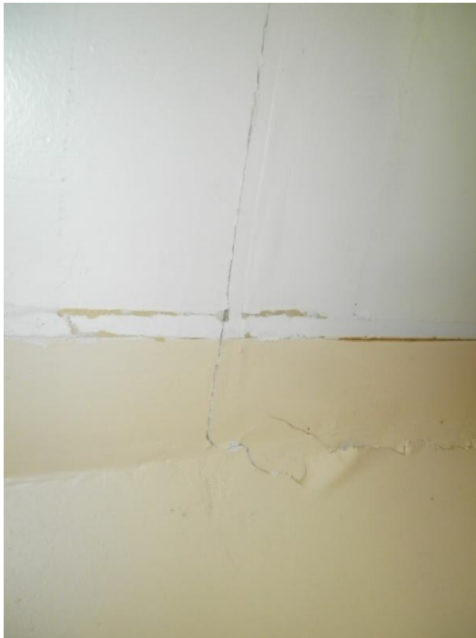
Lining damage at ceiling wall intersection
