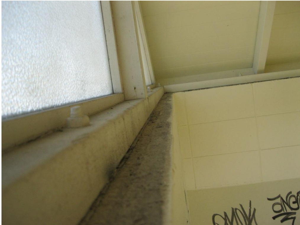
Photograph 5 Timber wall plate fixed to fully grouted concrete masonry wall with 12mm diameter bolts.
