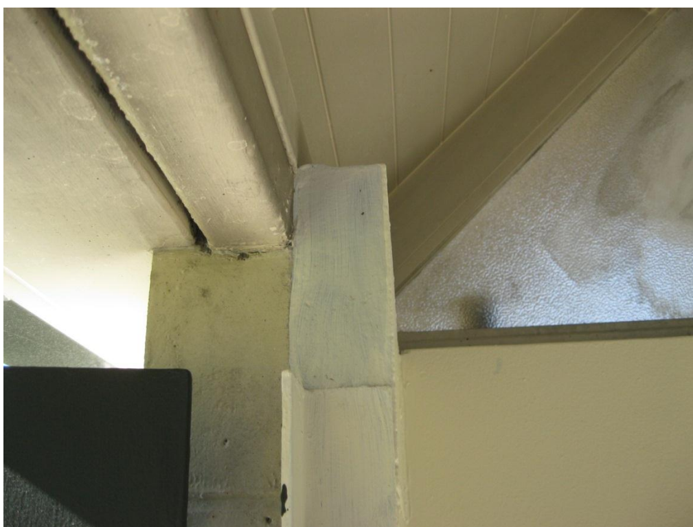
Photograph 3 Roof structure showing timber sarking, rafters and purlins.
