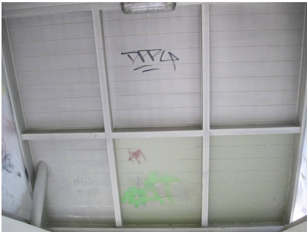
Photograph 3 Roof structure showing timber sarking, rafters and purlins.
