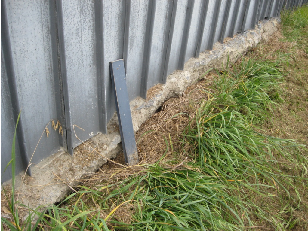
Photograph 7 Settlement of the retained ground to the north of the building.
