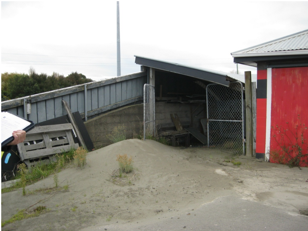
Photograph 2 Sand and silt from liquefaction piled outside the building and adjacent covered yard with concrete retaining wall.
