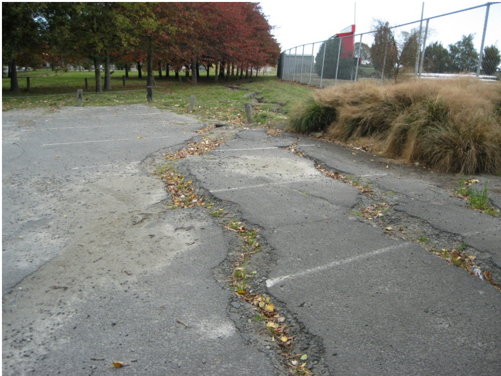
Photograph 8 Ground cracks near the river to the south of the garage.
