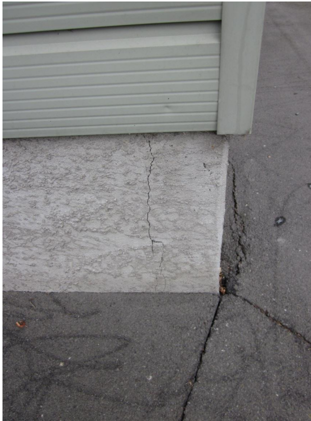
Photograph 5 Cracking to strip footing in the south-east corner of the building.
