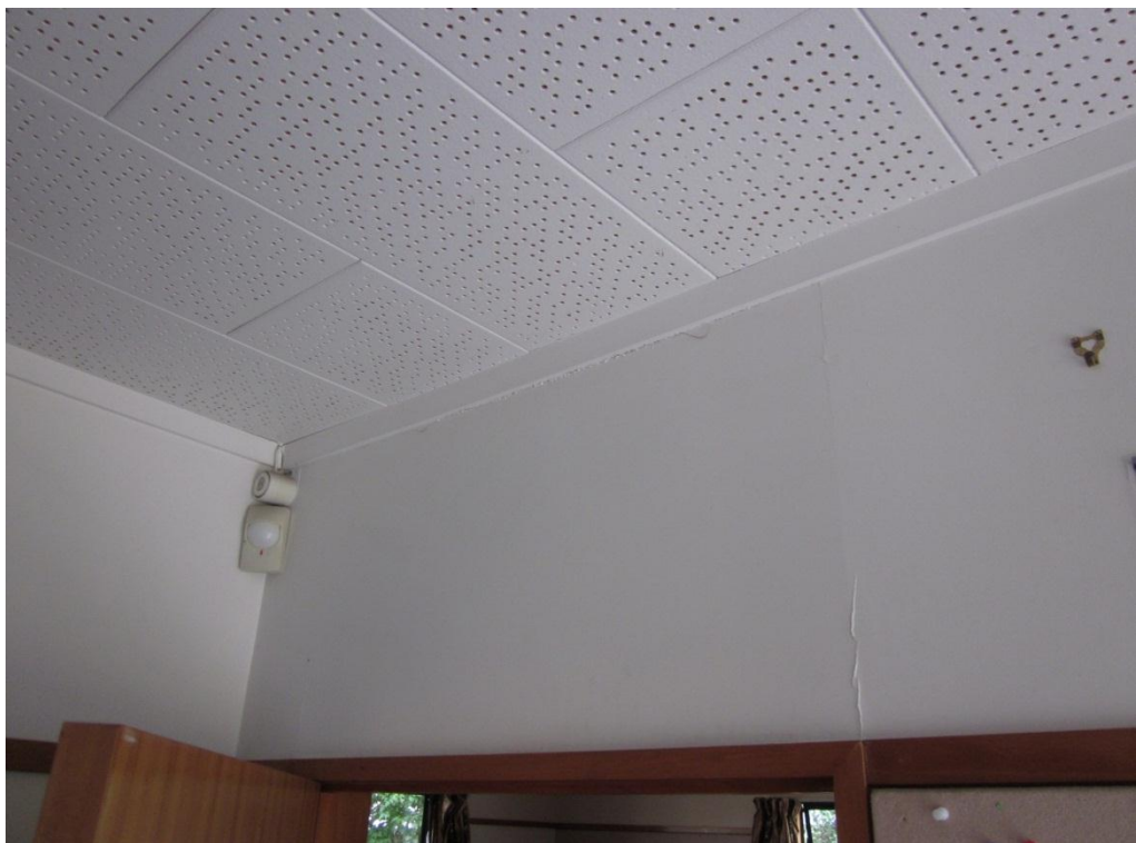
Photograph 8 Damage to GIB lining above doors.
