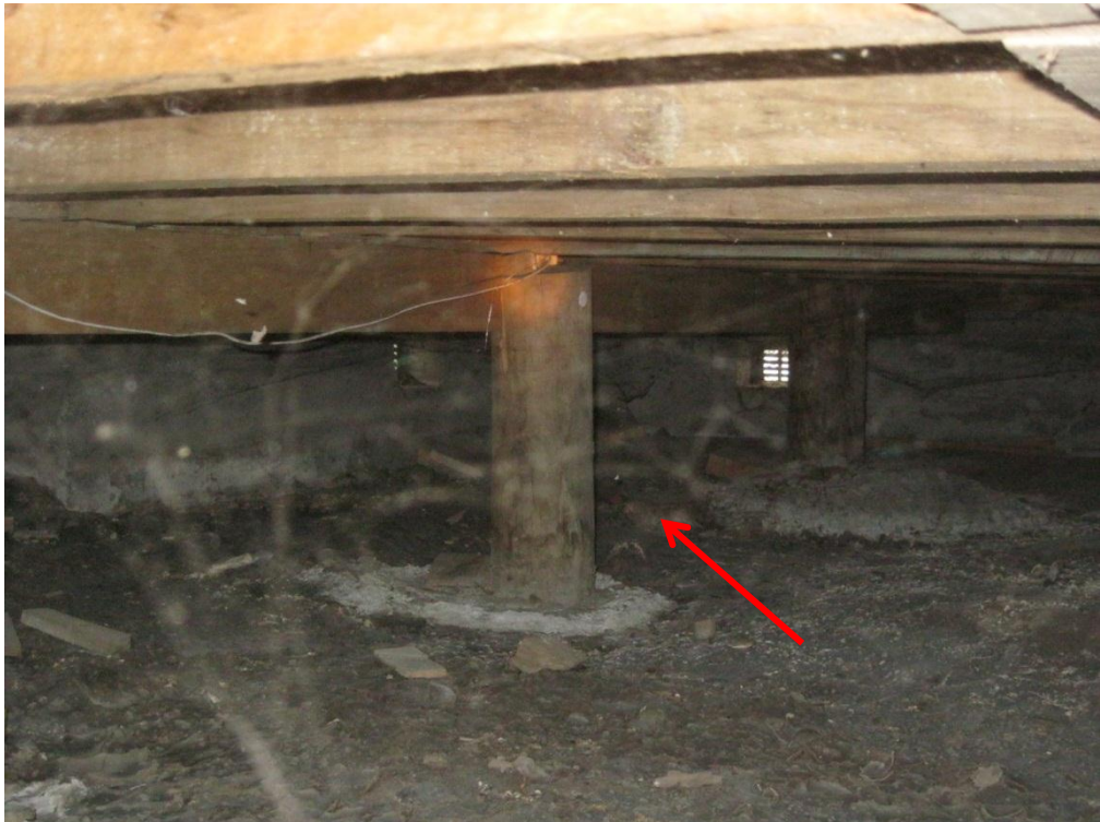
Photograph 11 Foundation piles at the south-west of the building where building has settled most. Evidence of significant liquefaction was observed at location of arrow.
