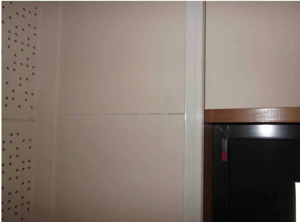
Photograph 7 Damage to GIB lining above doors.
