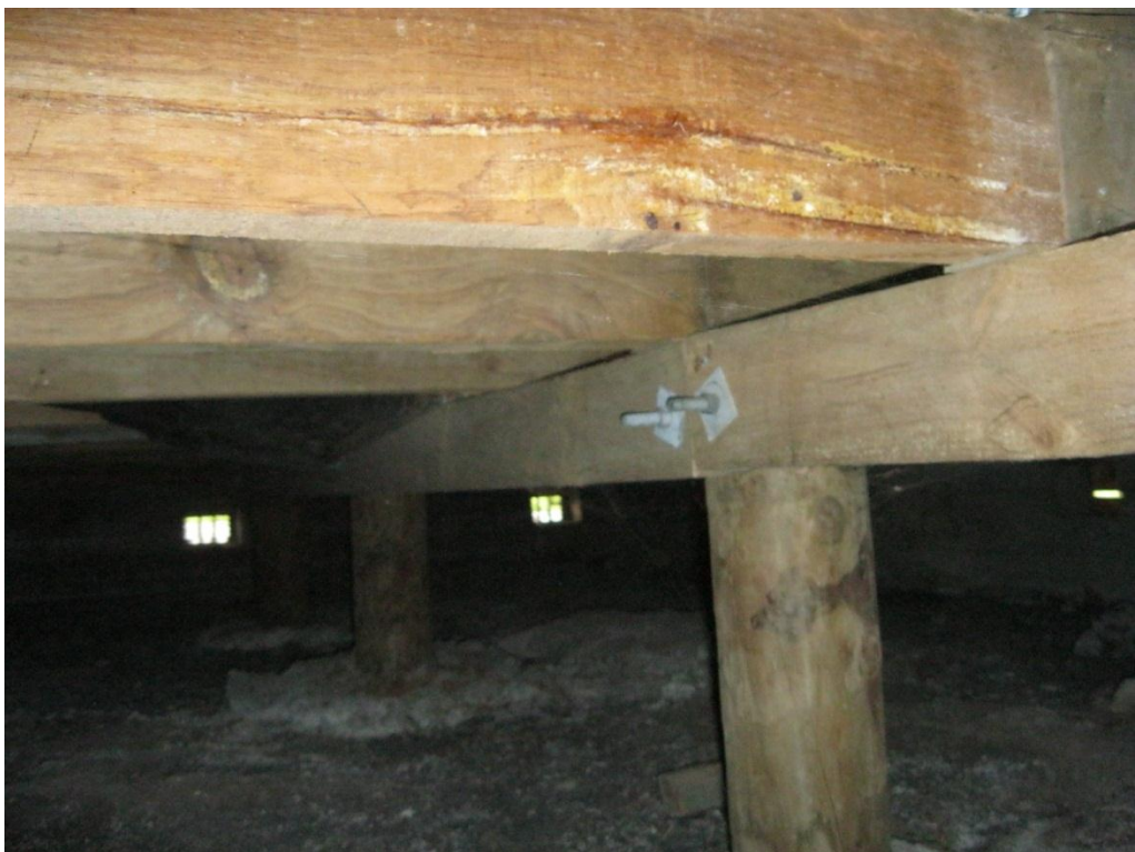
Photograph 10 Timber piles and bearers near the west of the building viewed from sub-floor space
