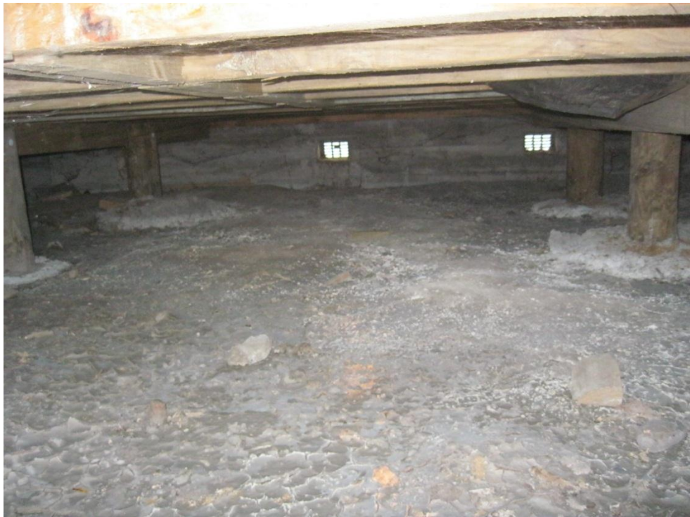
Photograph 12 Evidence of liquefaction of ground under the building.
