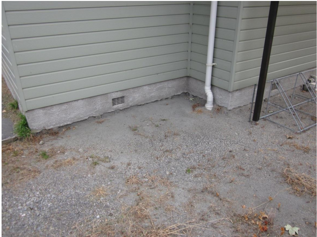
Photograph 3 Area where pavement was destroyed and settlement of surrounding ground occurred as a result of liquefaction.
