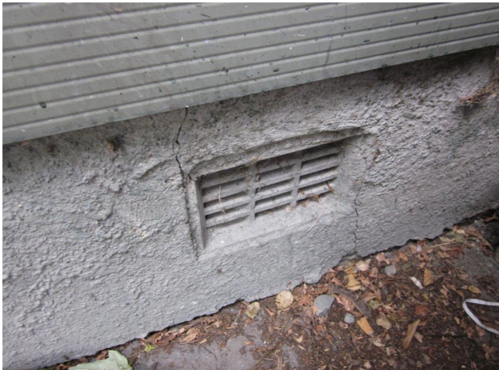
Photograph 6 Cracking to the strip footing to the north of the building.
