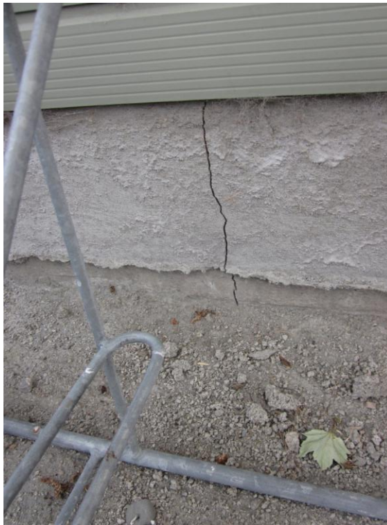
Photograph 4 Vertical cracking to perimeter footing in the south-west of the building.
