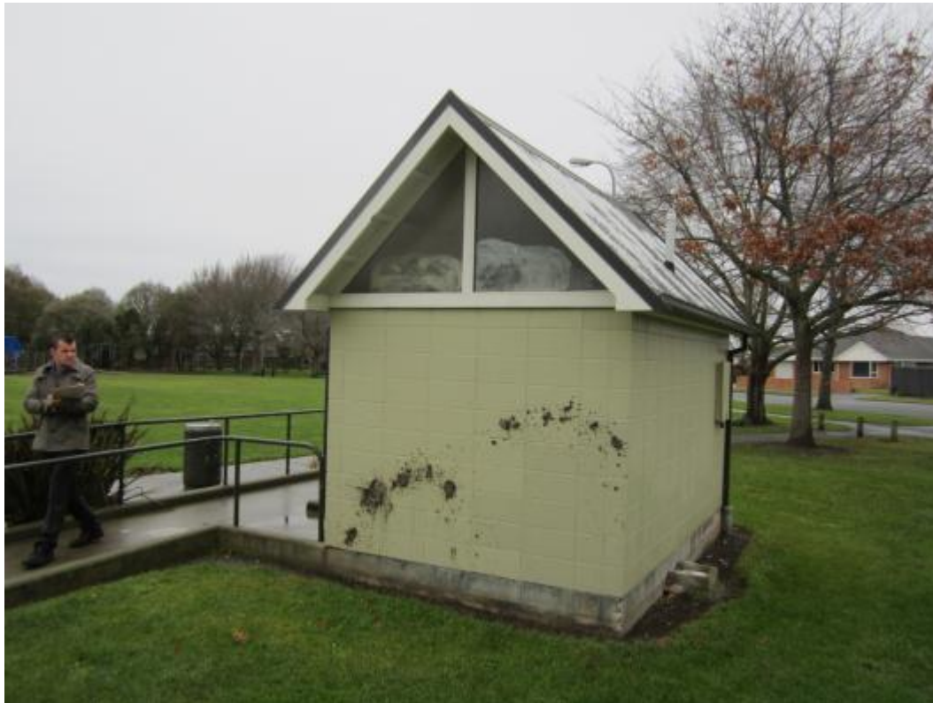
Photograph 3 View of duo-pitched timber roof structure
