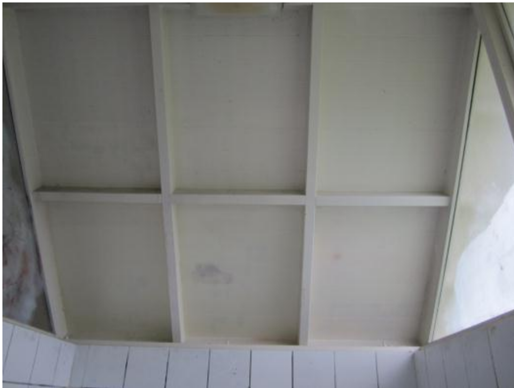
Photograph 4 View of timber sarking in roof structure
