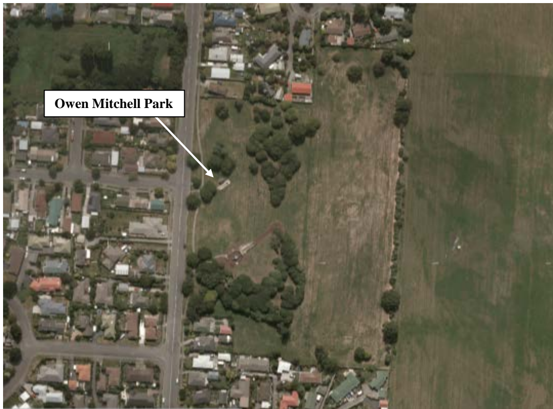
Figure 6.1 Post February 2011 Earthquake Aerial Photography 2
