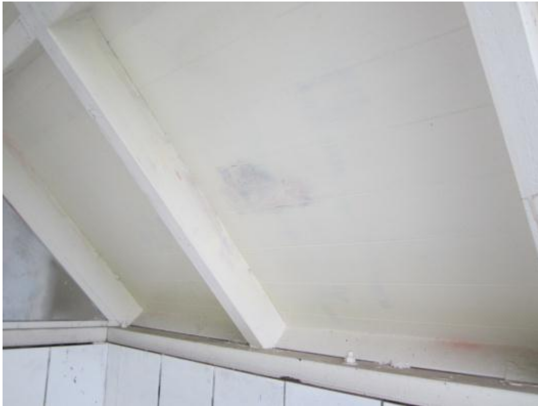
Photograph 5 Connection between timber roof framing and concrete masonry walls
