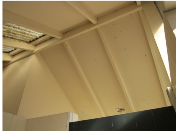
Internal view of the timber framed roof consisting of a ridge beam and rafters.
