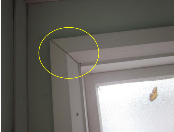
Photo 21: Mitre Joints on the Window Architrave in the toilet Area have Opened up
