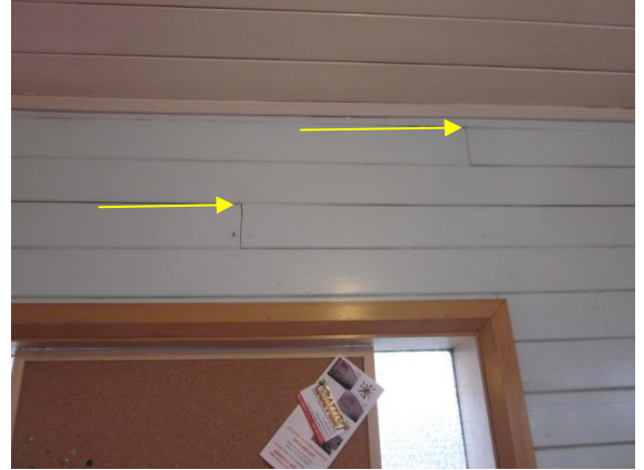
Photo 18: Hairline Cracks along Tongue & Groove Joints
