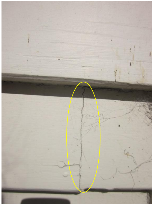
Photo 3: Hairline Cracking at Weatherboard Joints (typical)
