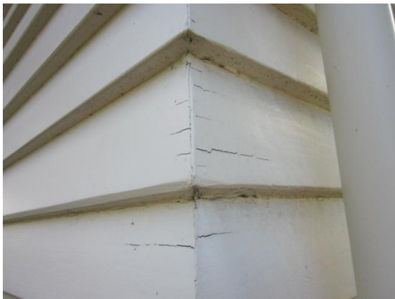
Photo 11: Existing Damage in the South East corner Exacerbated by EQ (SW Corner Similar)
