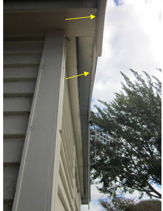
Photo 6: Hairline Cracking along Soffit Lining and Fascia Board Joint
