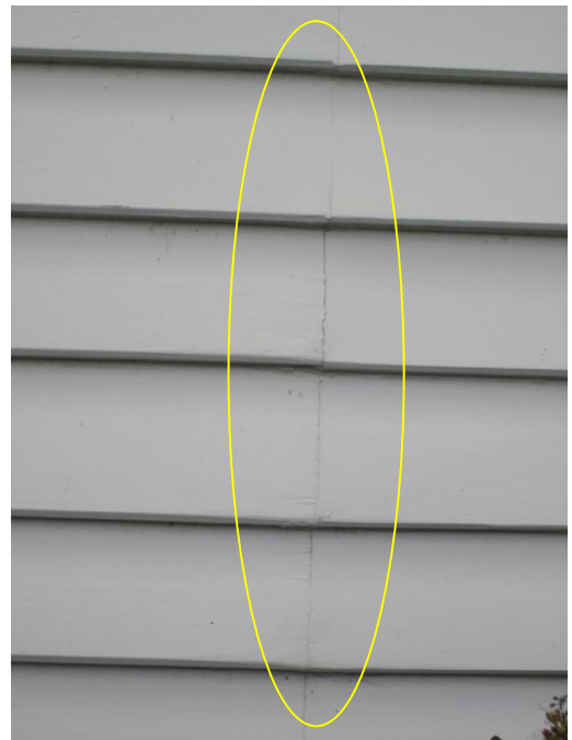
Photo 16: Hairline Cracks along Weatherboard Joints on the West Wall (typical)
