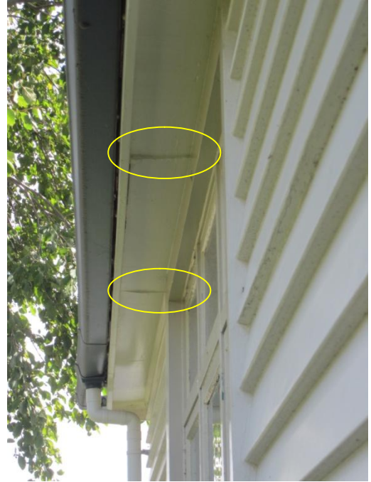
Photo 14: Hairline Cracking along Soffit Lining Joints on the South Wall
