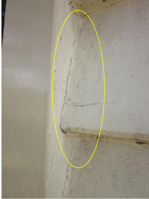
Photo 9: Hairline Cracking along the Window Architrave and the Weatherboard Joints
