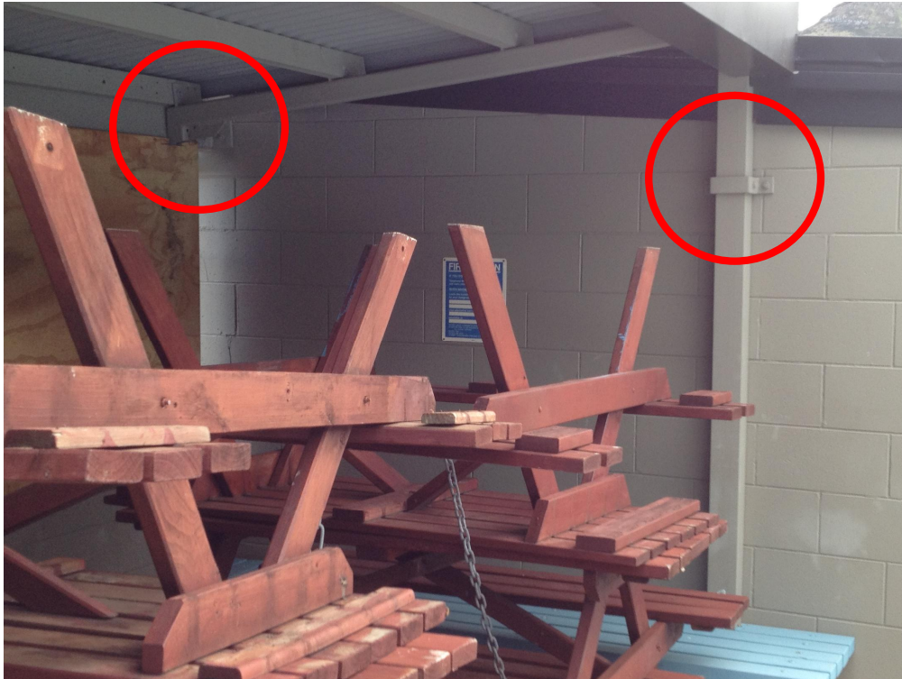
Photo 3: Connections to adjacent Ladies' Change Room eastern masonry wall.
