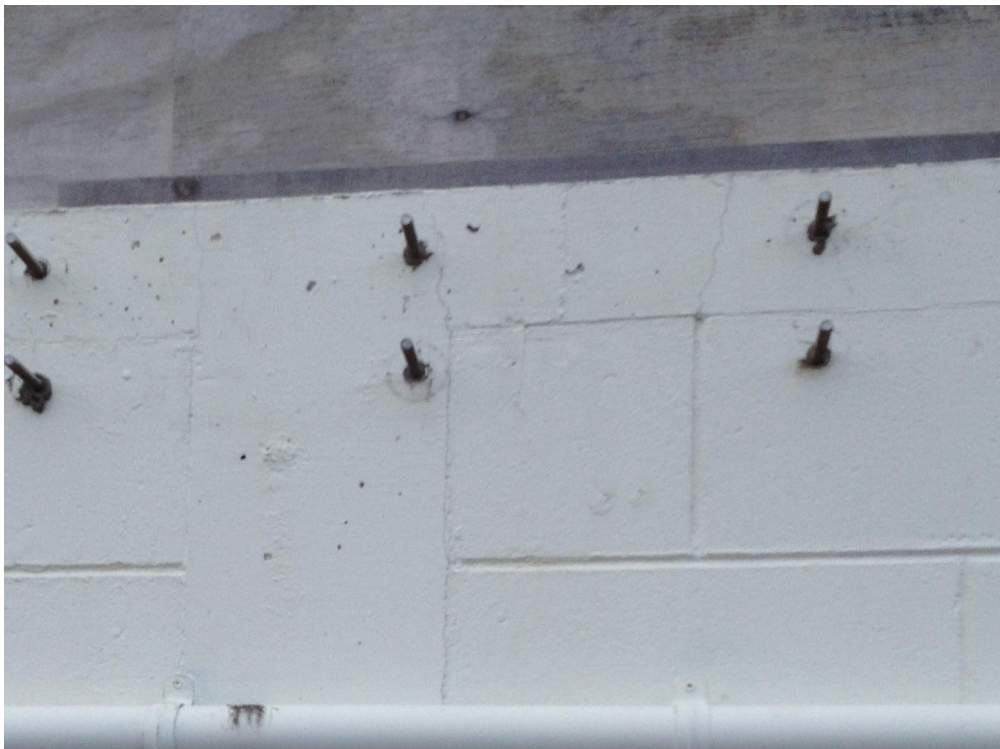
Photo 6: Concrete bond beam on top of the partial-height masonry block wall (view from south).
