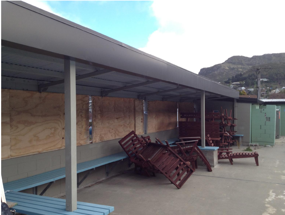
Photo 1: External view of Lean-to Shelter (view from north-east). Temporary plywood cladding has been installed to replace the broken glazing.
