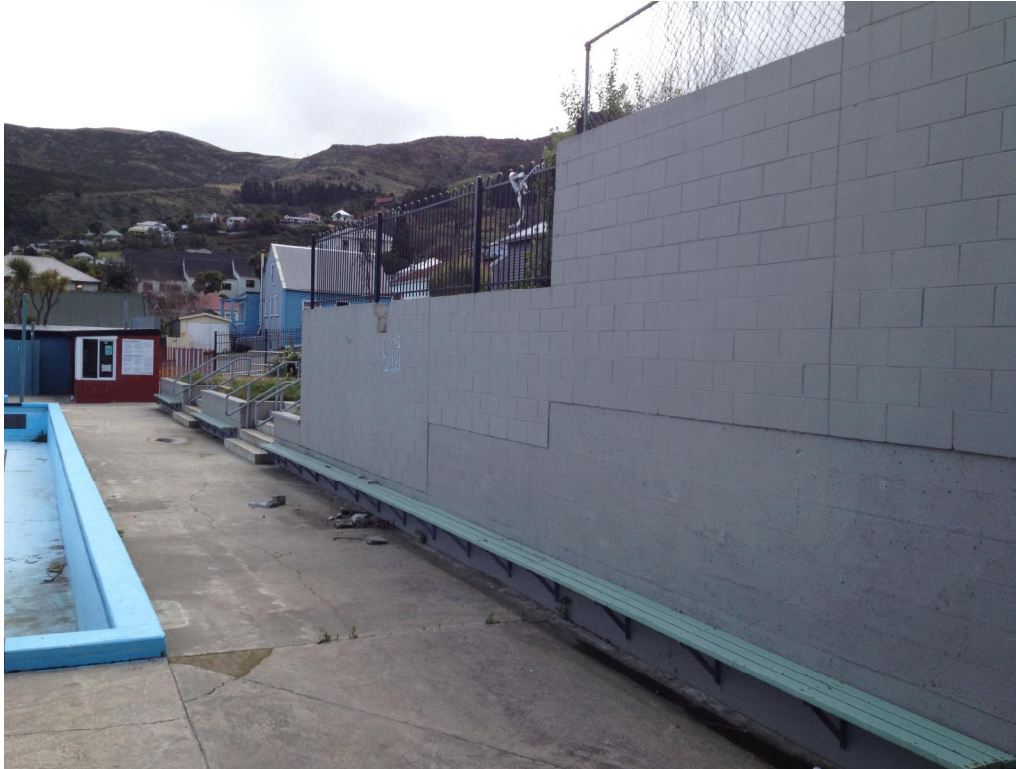
Photo 13: Concrete retaining wall and concrete masonry block fence to the north of the pool (view from south-east).
