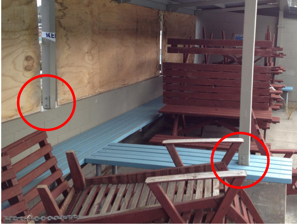
Photo 5: U-bracket connections between columns and concrete plinth (on the right) and concrete masonry wall (on the left).
