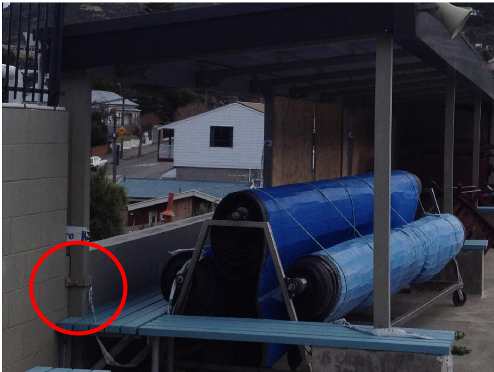
Photo 4: Connection to concrete masonry wall extending to the east.
