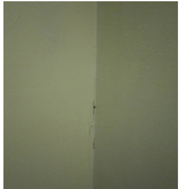
Photo 8: Typical separation of linings in corners
