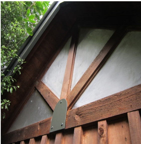
Photo 3: Close up of timber truss
