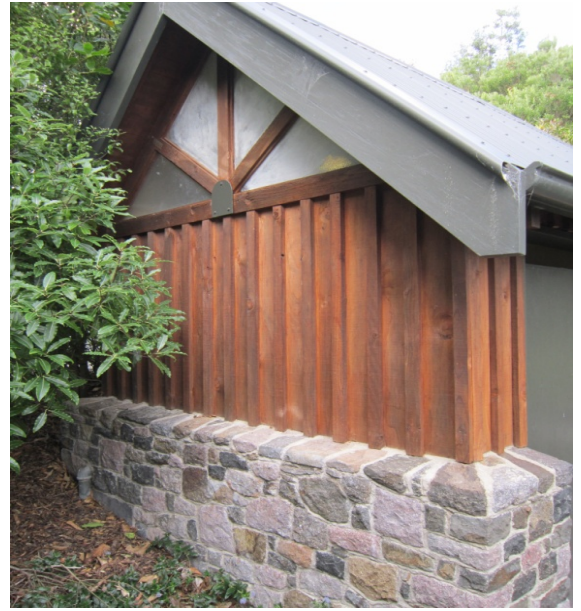
Photo 2: North side of the building showing construction – Steel cladding, timber roof trusses, light timber framed walls and stone masonry
