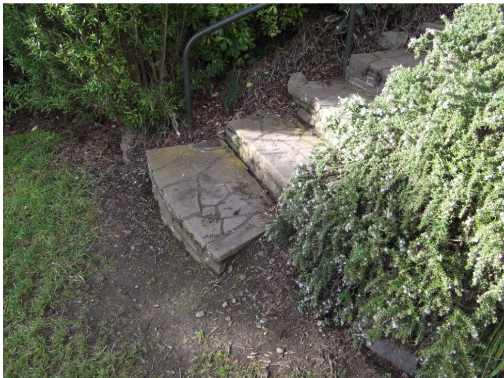
■ Figure 6 – 10 mm crack in between steps approximately 15m west of the building.
