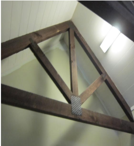
Photo 5: Trusses connected using nail plates which do not appear to have suffered damage
