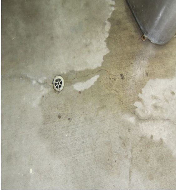
Photo 9: Cracking propagating through floor slab from drainage penetration hairline ~ 0.4mm cracks
