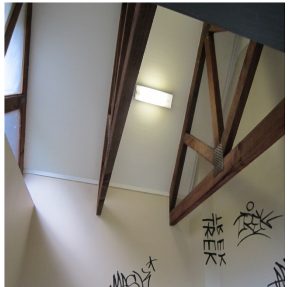
Photo 4: Timber trusses spaced at approx 800mm crs.
