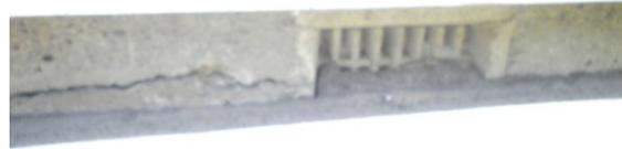
Vertical crack at cladding junction between original structure and later addition.
