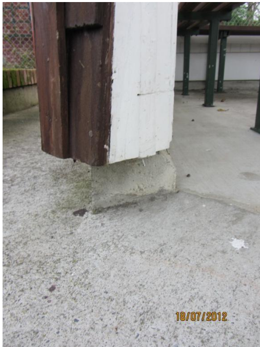
Photo 7: Concrete strip footing
