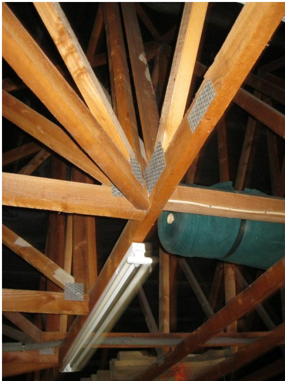
Photograph 6 Internal roof trusses connection.
