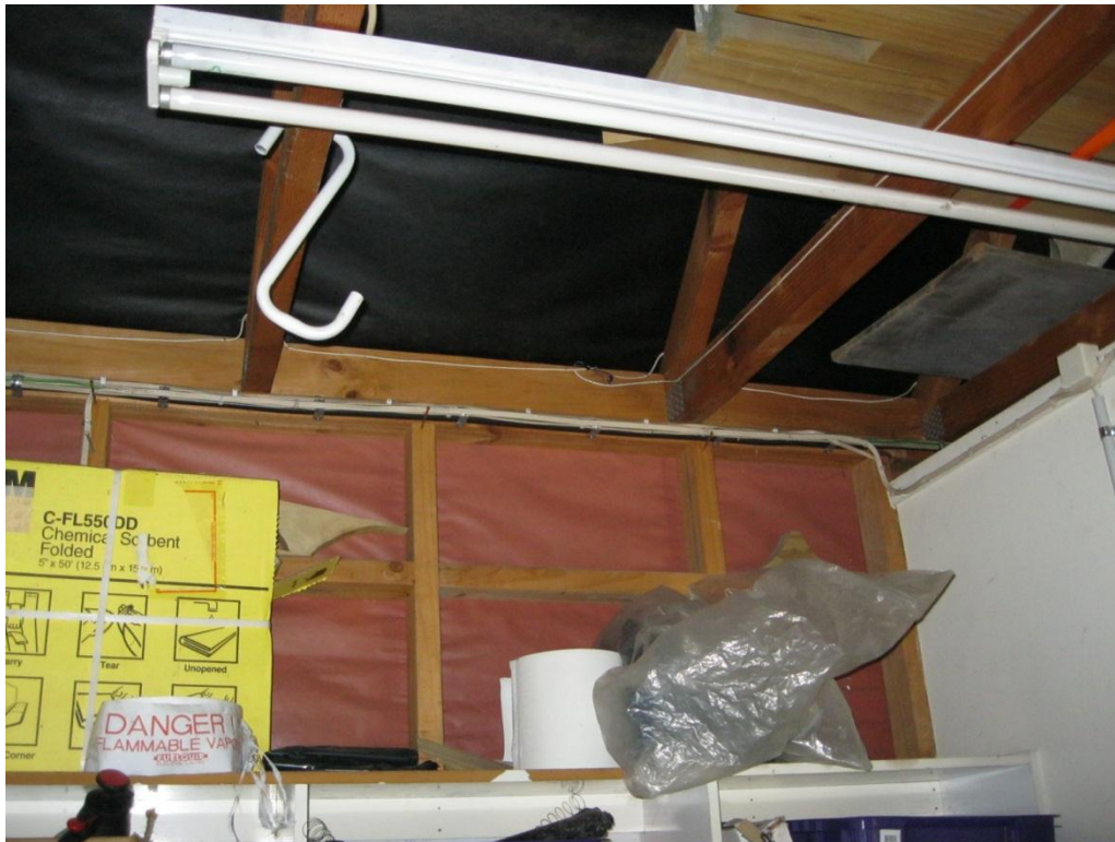
Photograph 7 Connection between roof trusses and timber wall.
