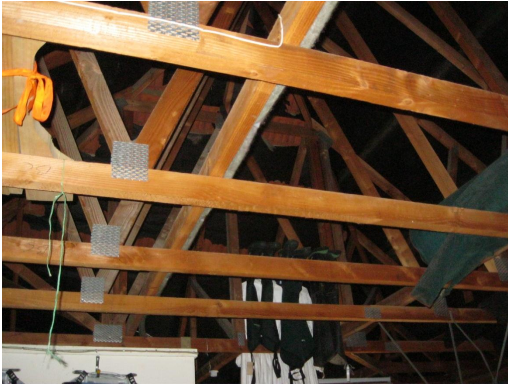
Photograph 5 Roof truss nail plate connections.
