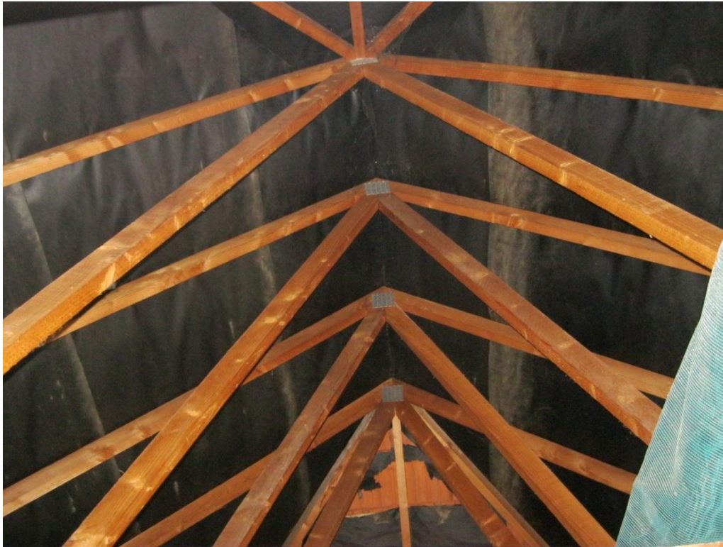
Photograph 3 Internal roof trusses.
