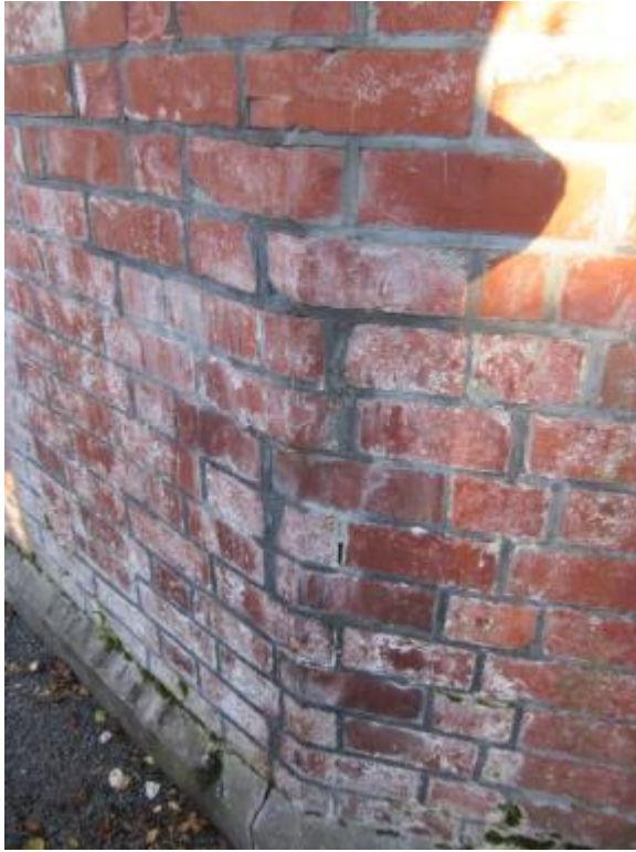
Photo 9. Repointed Unreinforced Brick Masonry Joints.
