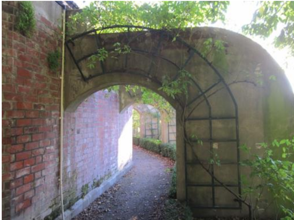
Photo 6. Unreinforced Brick Arch Buttress.
