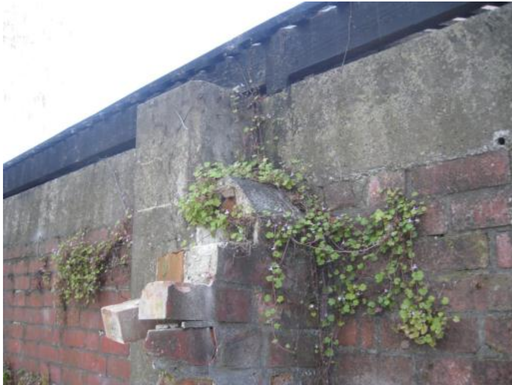
Photo 11. Brick arch previously connecting the boundary wall to structure.
