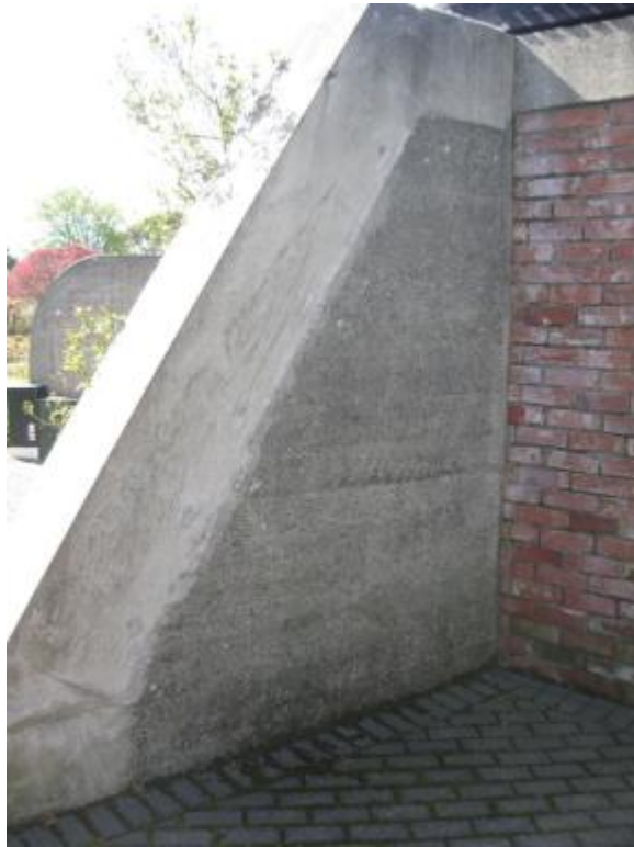
Photo 5. Reinforced concrete buttress..
