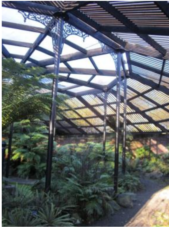
Photo 3. Posts supporting pergola roof structure.
