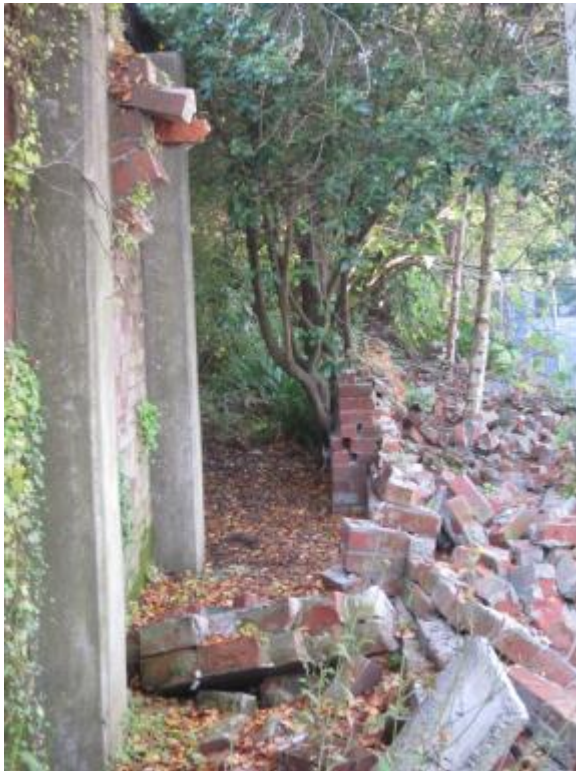
Photo 10. Collapsed Boundary Unreinforced Brick Masonry Wall adjacent to structure.
