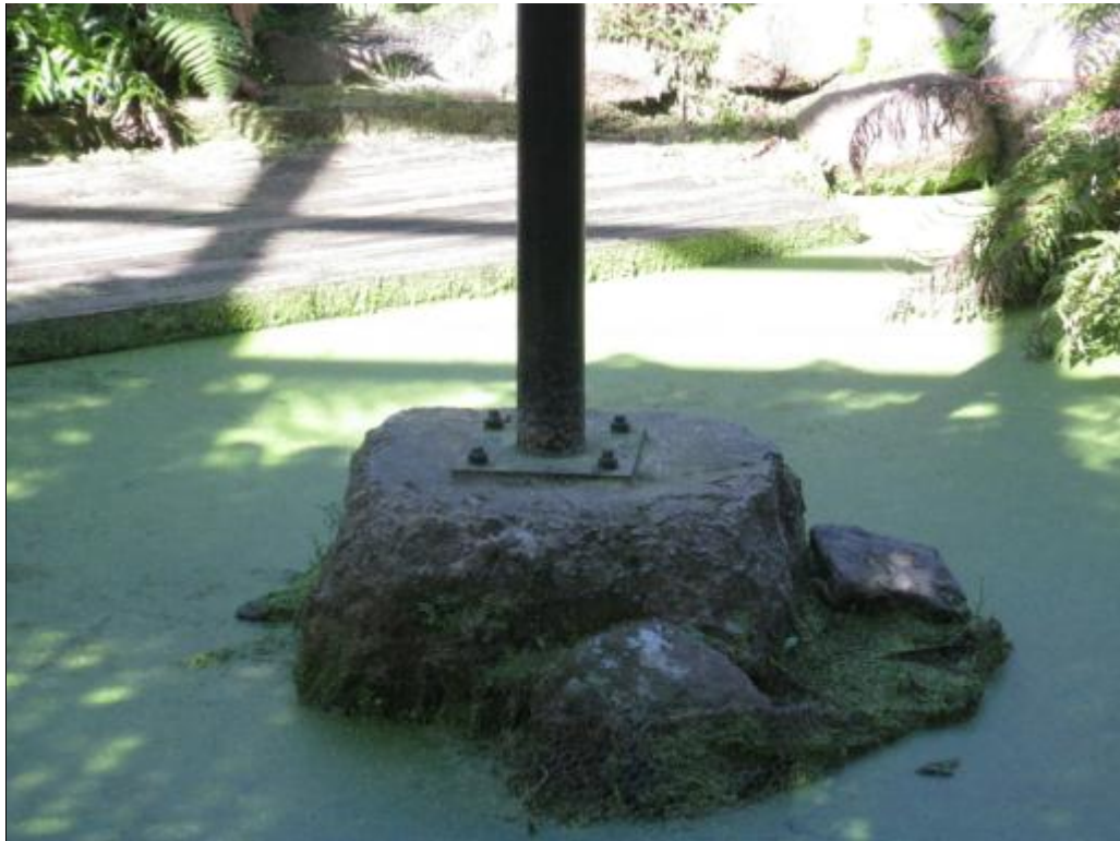
Photo 8. Pad Foundation for Post.
