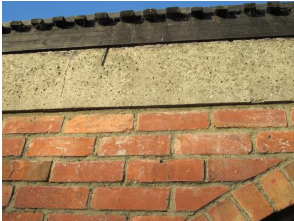
Photo 7. Reinforced Concrete Ring Beam.
