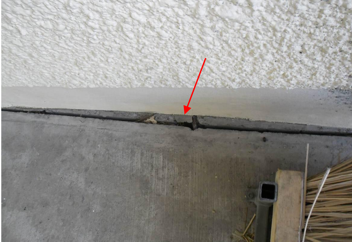
Photo 7: Settlement and separation at east entrance with exposed rebar
