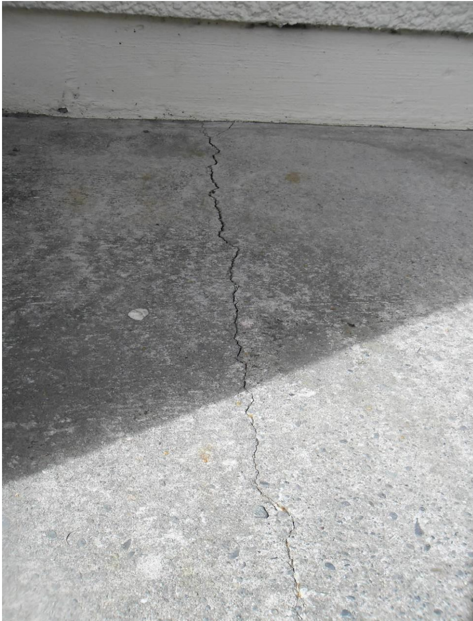
Photo 3: Typical cracking to concrete footpath at outside of the building
