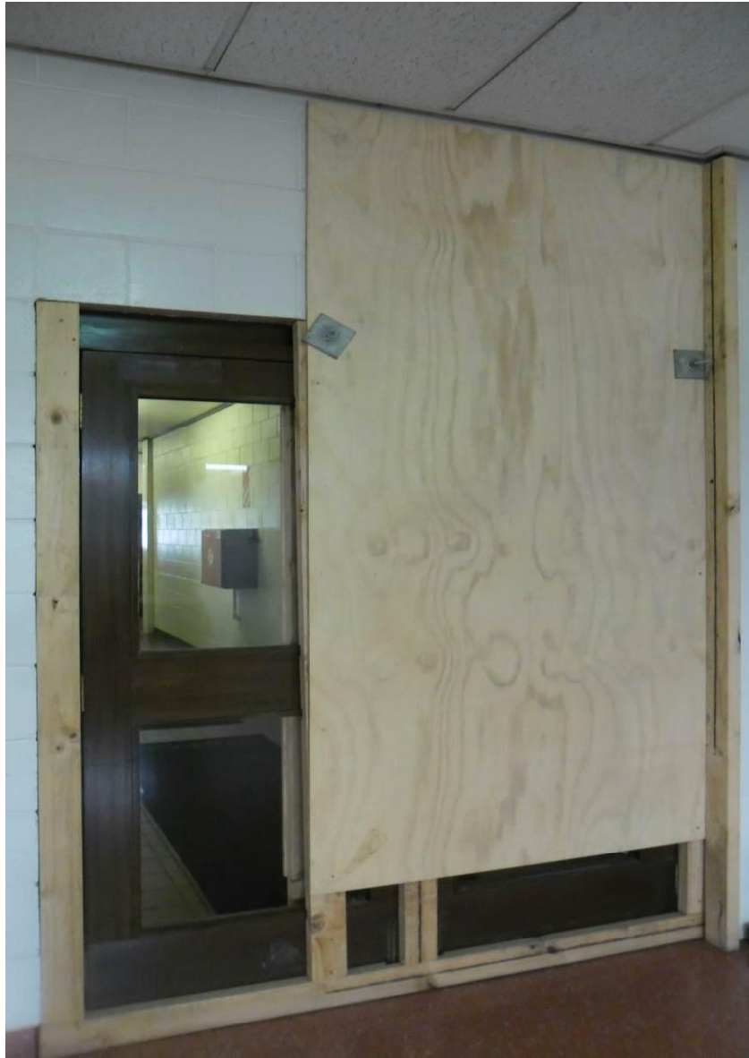
Photo 10: Plywood propping at lunch room
