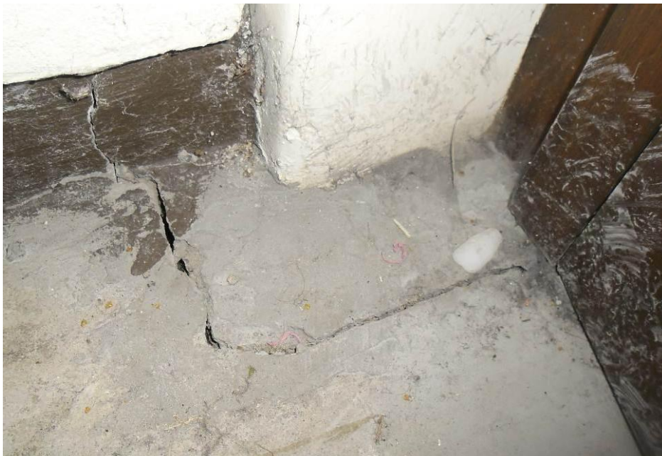
Photo 12: Evidence of foundation settlement below the concrete column
