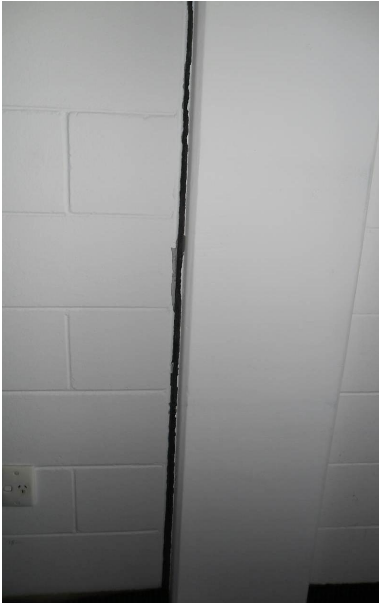
Photo 13: Separation between masonry and column at Client Service office
