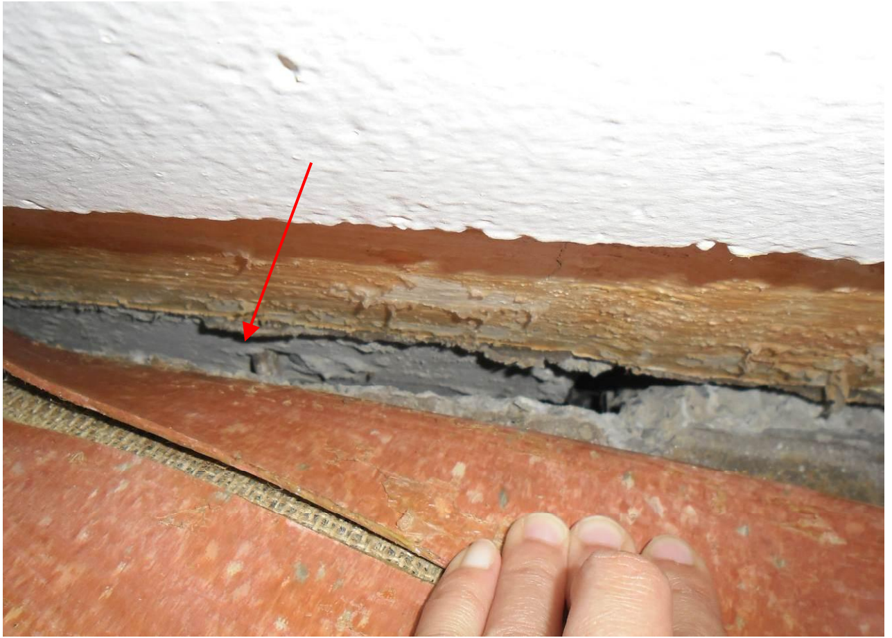
Photo 9: Cracking to concrete slab with exposed reinforcement at Client Service office
