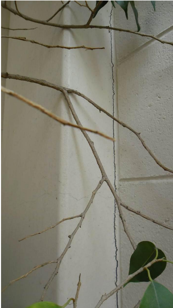
Photo 17: Typical separation between masonry blocks and concrete column
