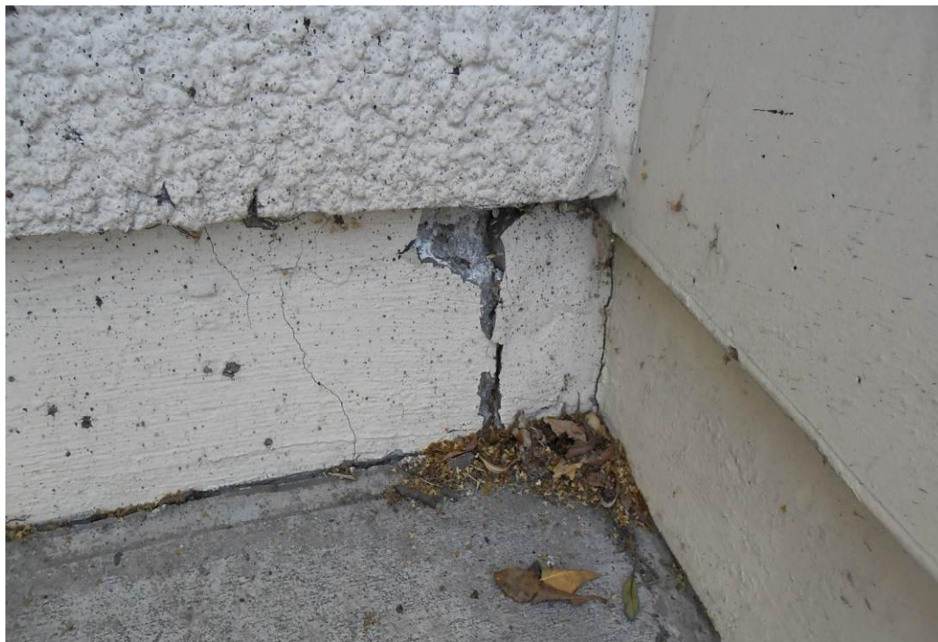
Photo 2: Typical cracking and spalling to concrete foundation walls
