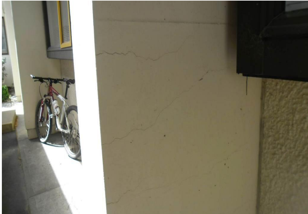
Photo 1: Typical crack to perimeter concrete column
