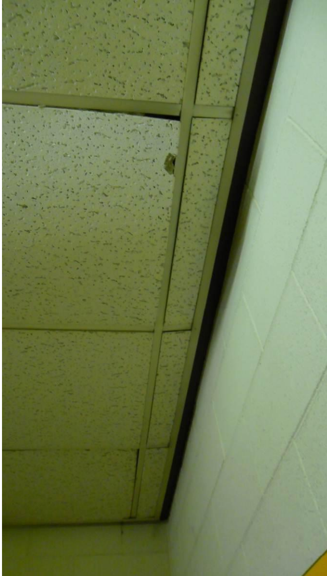
Photo 15: Typical damage to suspended ceiling tile and framing
