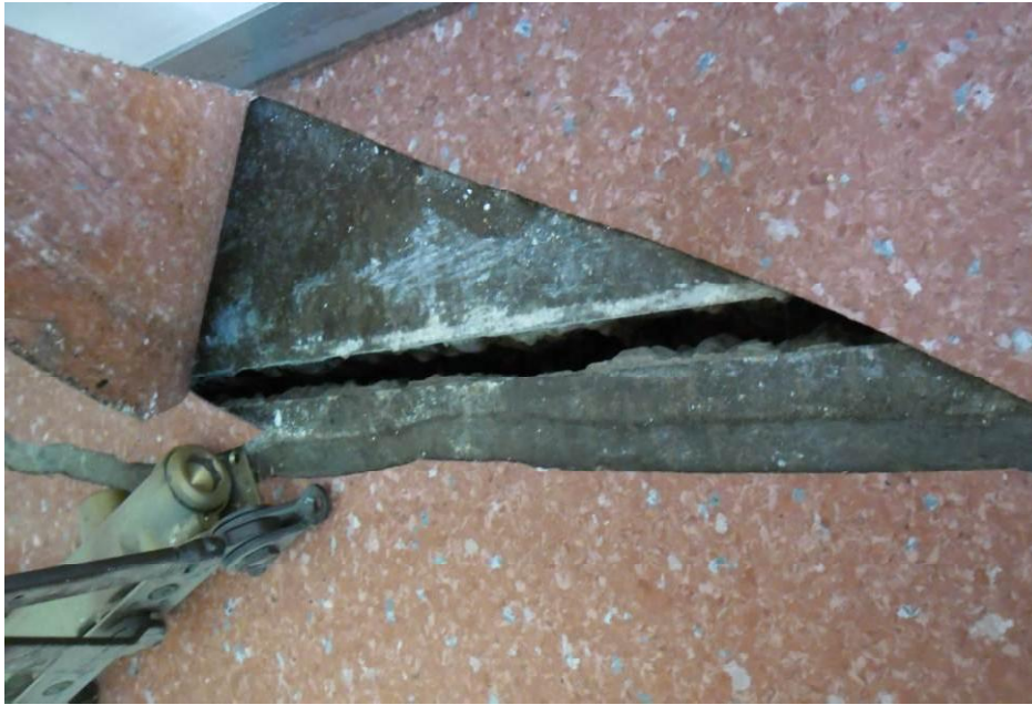
Photo 11: Cracking to concrete slab at the east wall of Lunch Room
