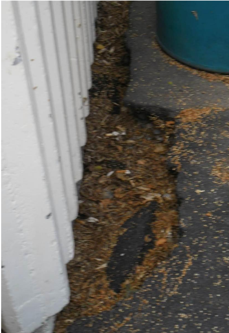
Photo 6: Evidence of ground movement at the southern face of the building
