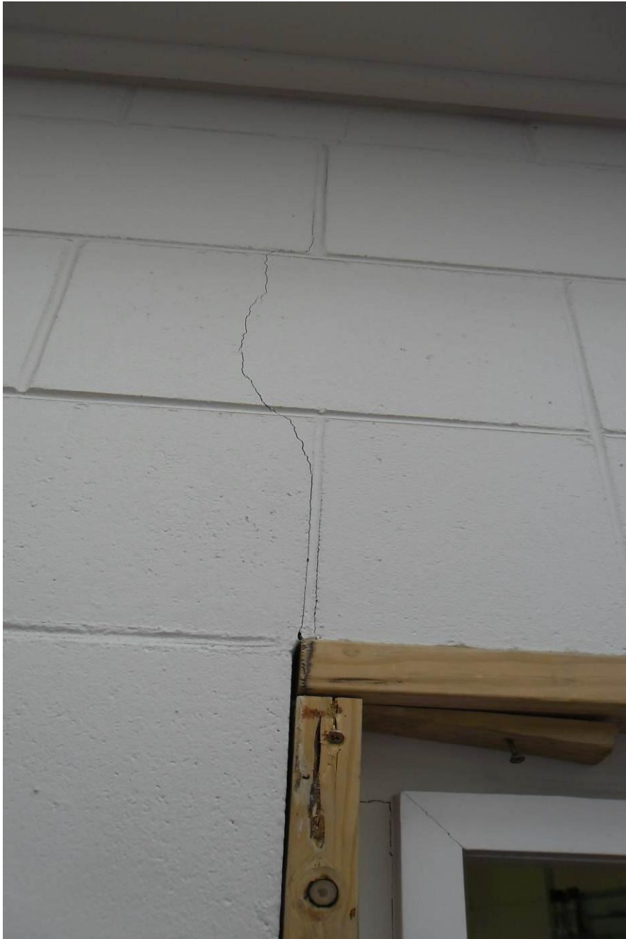
Photo 8: Typical cracking to masonry blocks
