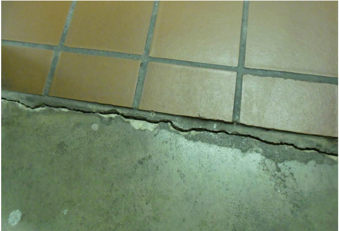
Photo 14: Cracking to concrete slab along the Locker Room Hallway
