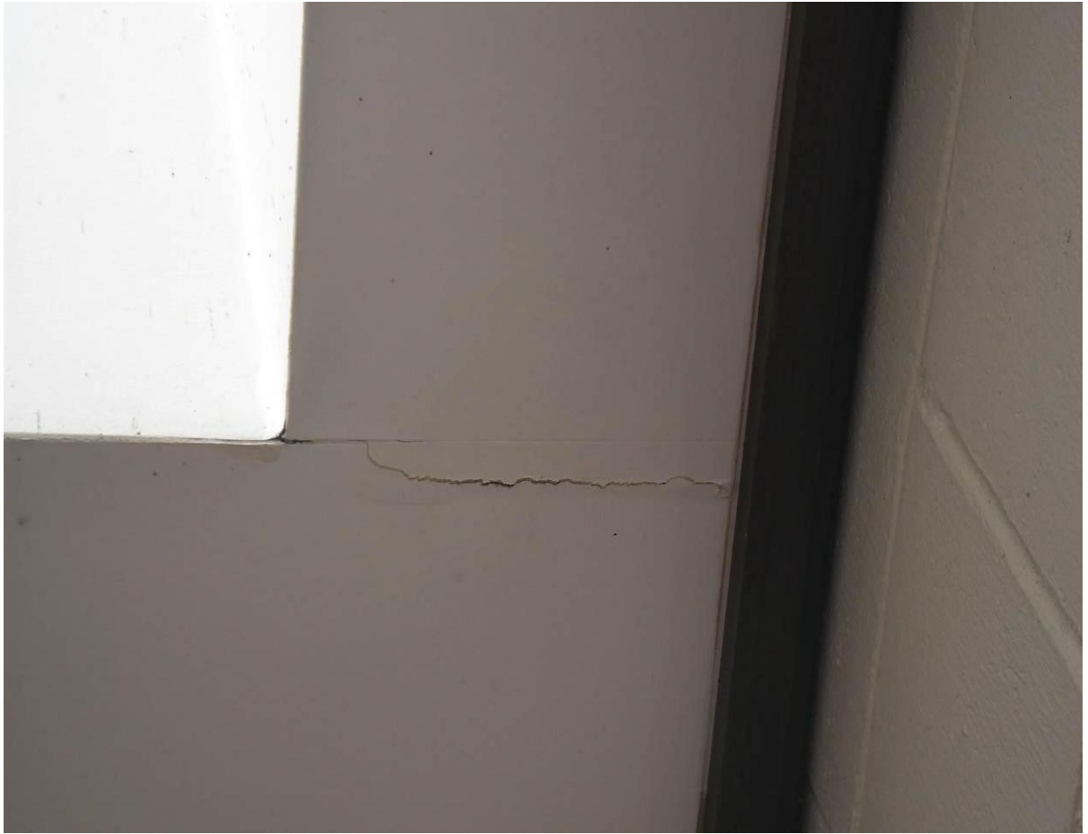
Photo 16: Typical cracking to gypsum plasterboard in the ceiling
