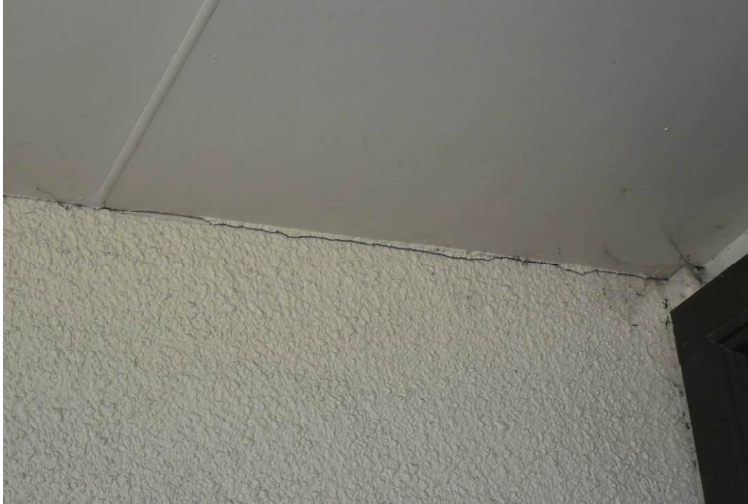
Photo 5: Separation between ceiling and masonry wall at the southern face of the building
