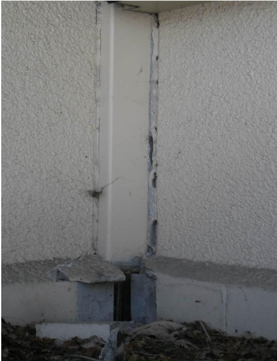
Photo 4: Significant separation at south face of the building
