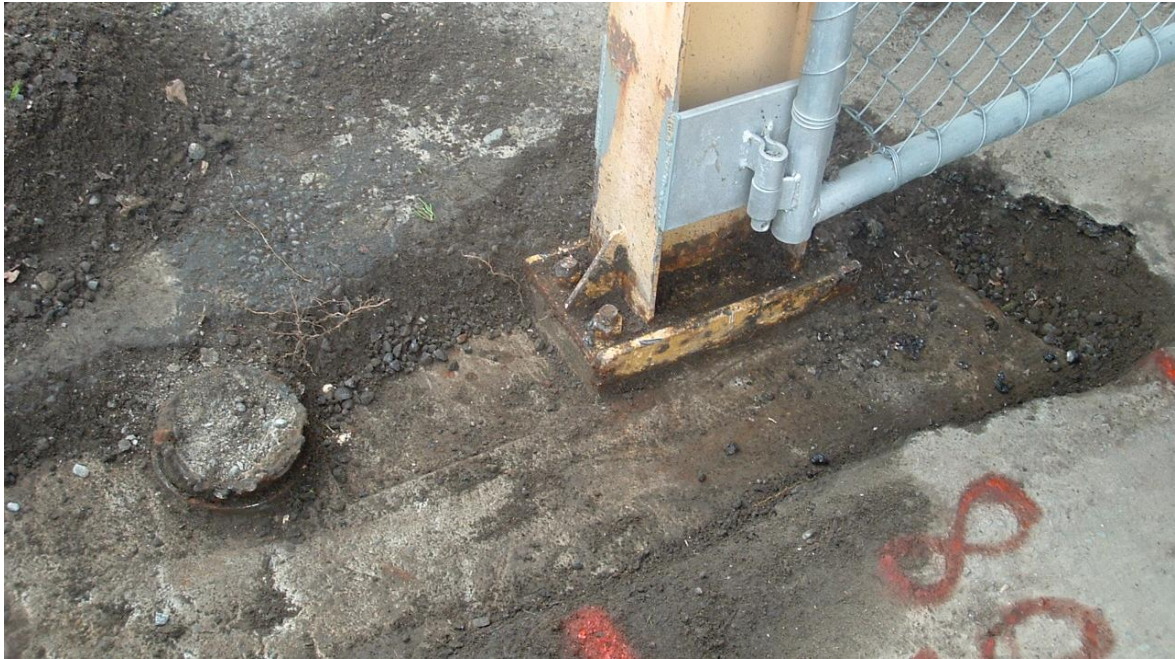
Photo 5: Typical western portal frame column foundation.
