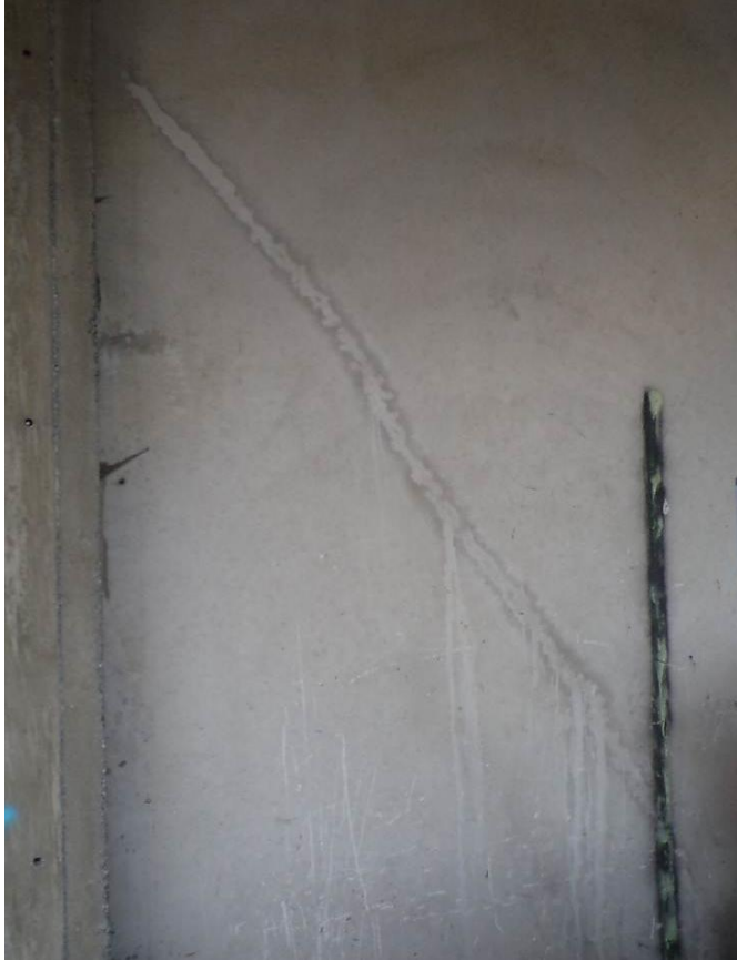
Photo 7: East precast tilt panel wall damage
