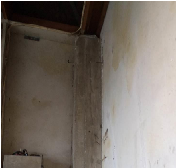
Photo 6: Internal concrete column and precast tilt panel.
