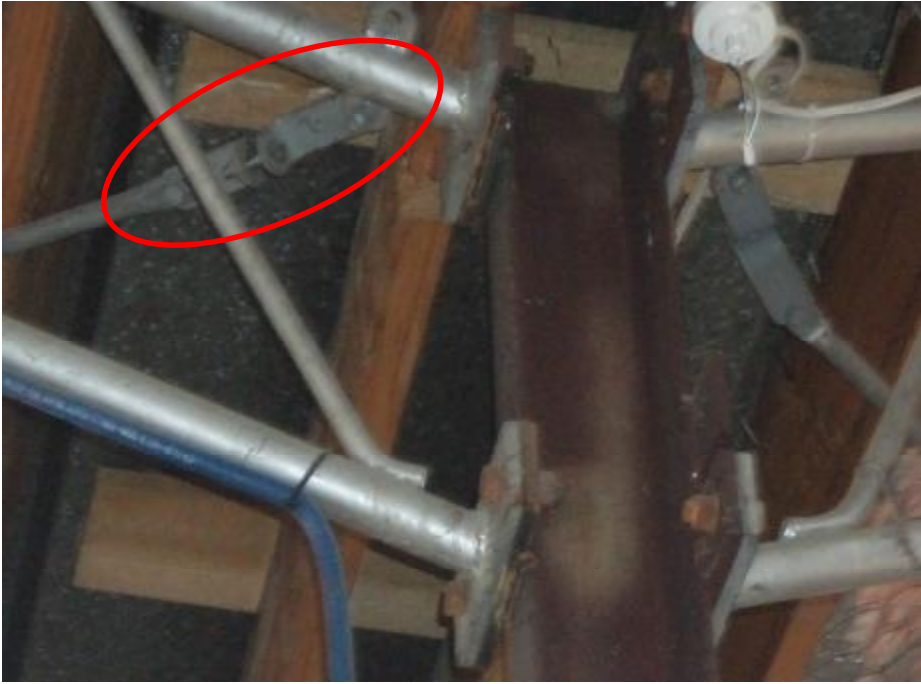
Photo 6: Roof bracing connection
