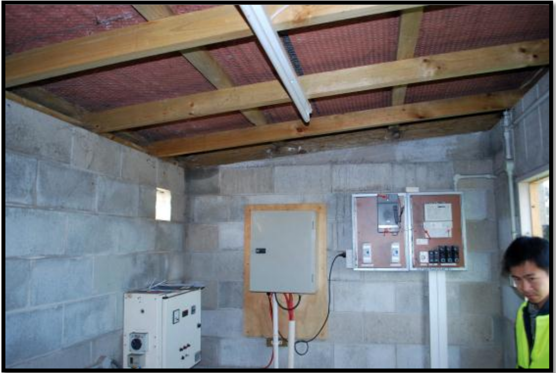
Photograph 7 Timber roof structure.
