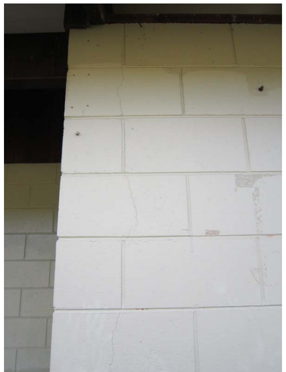
Photo 24: Cracking through masonry elements and mortar joints on the south side.
