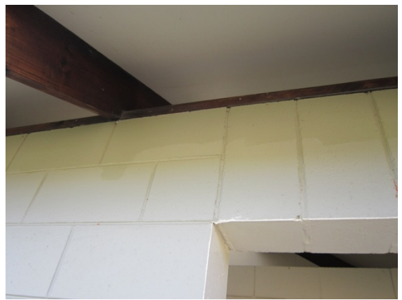
Photo 26: Timber roof rafter and timber edge beam on top of masonry wall over entrance to women's toilets
