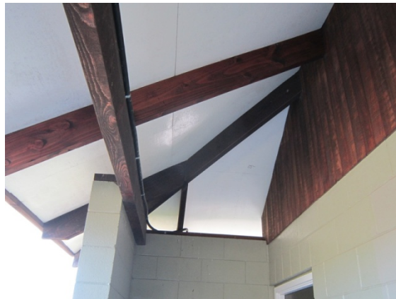
Photo 7: Timber roof rafter layout on the southwest corner.
