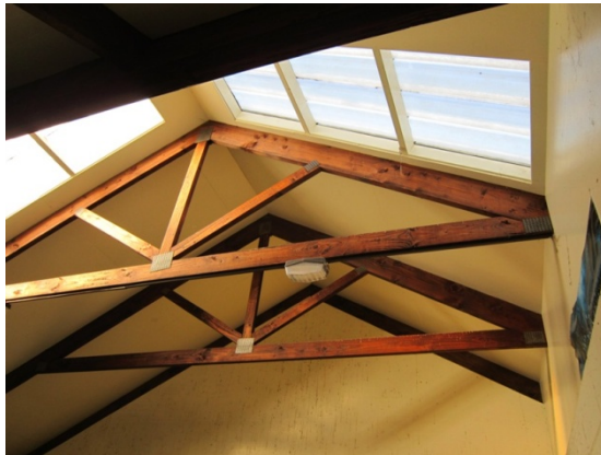
Photo 17: Timber roof trusses in the changing room.
