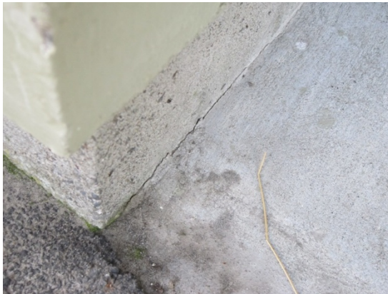
Photo 9: Crack between concrete strip footing and concrete ground slab.
