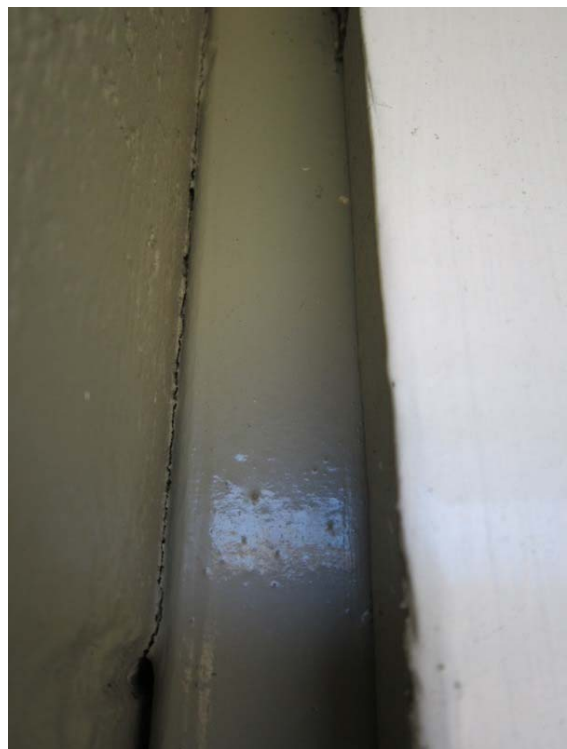
Photo 23: Gaps opening up between timber elements in the doorframe and the masonry wall on the south side
