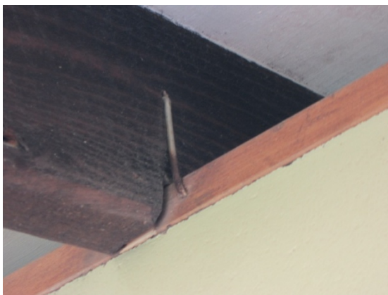
Photo 11: Connection between timber roof rafter and timber edge beam on top of masonry wall.
