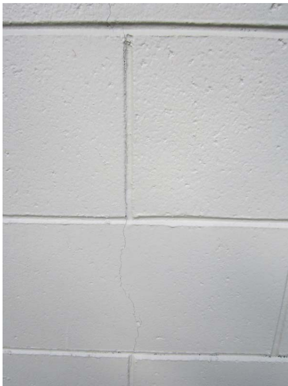
Photo 43: Crack through masonry elements and mortar joints on the west wall.
