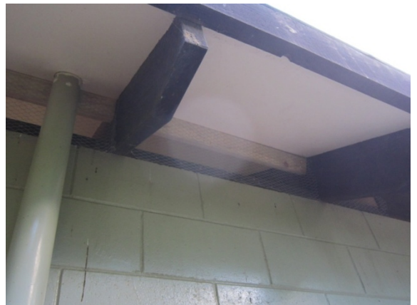
Photo 40: Timber roof rafters and timber edge beam above the north wall.
