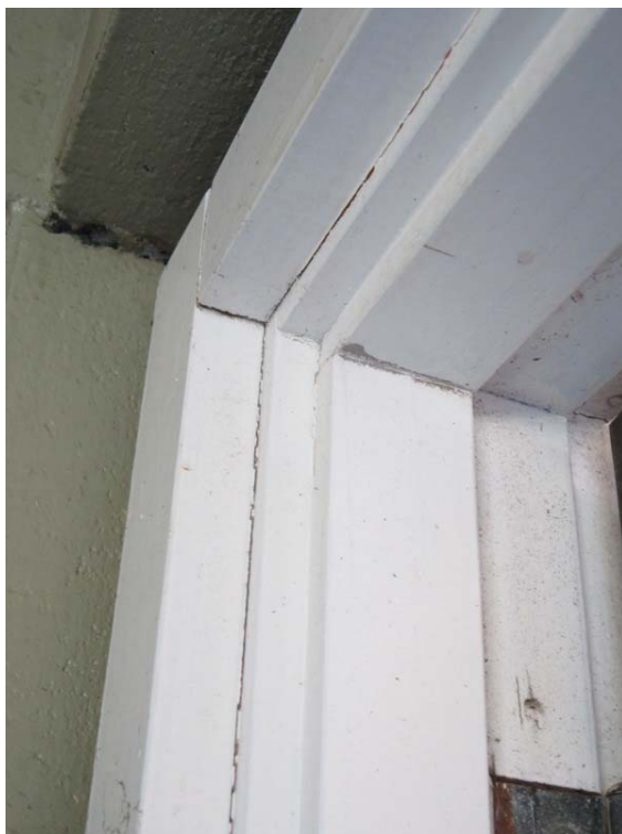
Photo 15: Gaps opening up between timber elements on the changing room doorframe.
