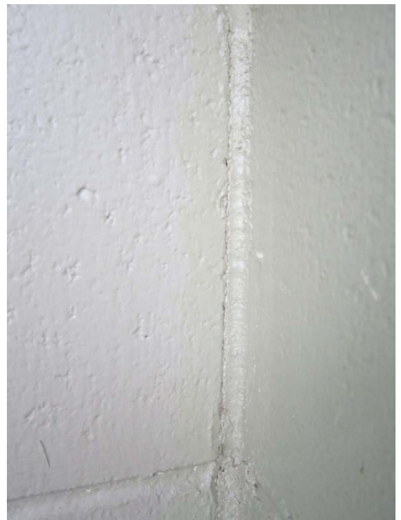
Photo 20: Crack in mortar joint at intersection of perpendicular walls on the south side.
