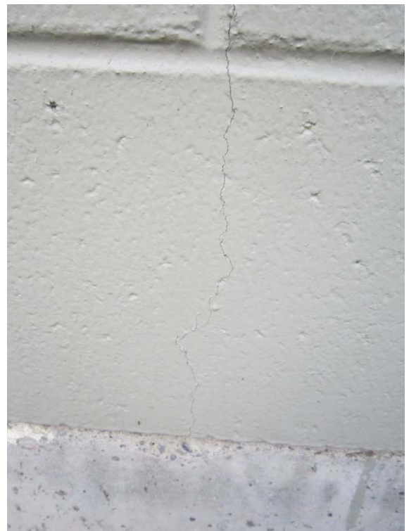
Photo 44: Crack through masonry elements and mortar joints on the west wall.
