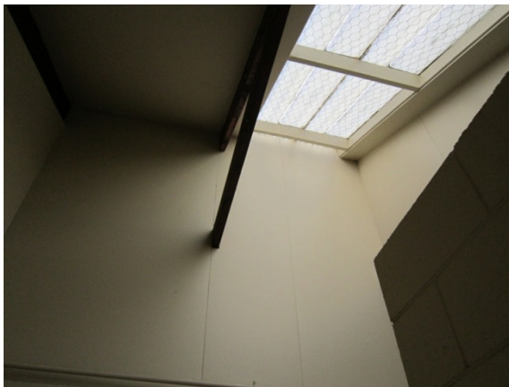
Photo 31: Roof layout inside the women's toilets, with plasterboard cladding on the walls above the masonry blocks.
