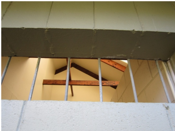
Photo 35: View through ventilation gap in east wall showing roof rafters in the men's toilets.
