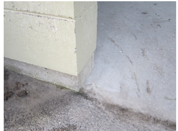
Photo 8: Concrete strip footing directly under the masonry wall on the south side.
