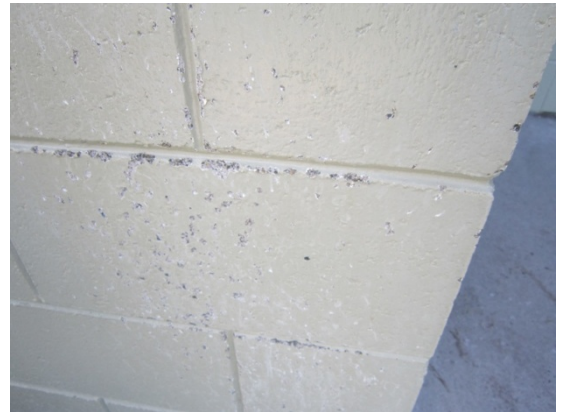
Photo 10: Paint removal on south wall.
