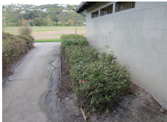
Photo 39: Cracking in footpath on the east side of the building.
