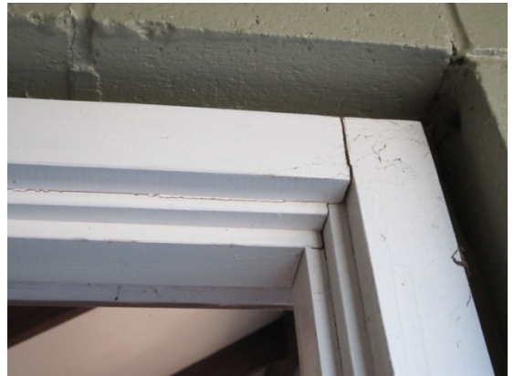
Photo 14: Gaps opening up between timber elements on the changing room doorframe.
