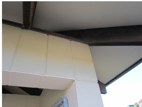
Photo 27: Timber roof rafter and timber edge beam on top of masonry wall over entrance to women's toilets
