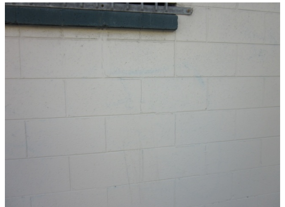
Photo 8: Blockwork cracking on the eastern facade.
