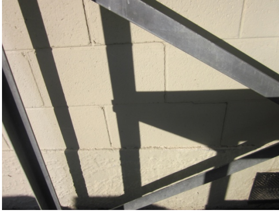
Photo 9: Blockwork cracking on the western facade.
