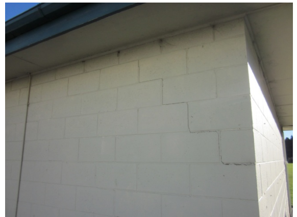
Photo 4: Blockwork cracking on the eastern facade.
