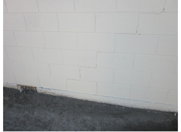
Photo 6: Blockwork cracking on the eastern facade.
