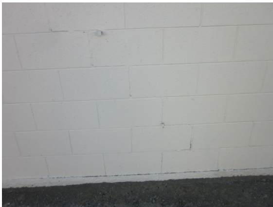
Photo 7: Blockwork cracking on the eastern facade.
