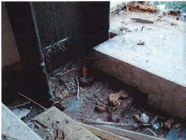
South-east gymnasium portal column: No bolt fixing into masonry wall. Base plate welded to bar cast into the wall.
