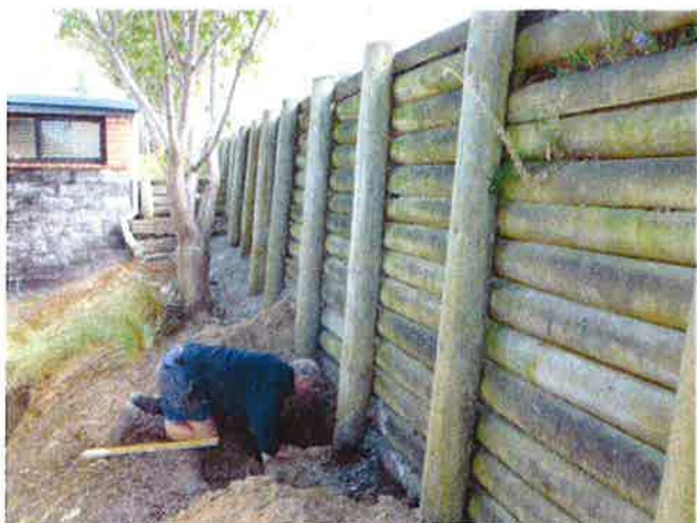
Timber poles embedded 1.85m into ground.
