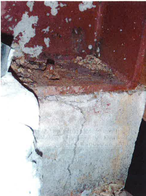
Portal column in squash courts area: No nut to threaded rod cast into masonry wall. Base plate tack welded to threaded rod instead.
