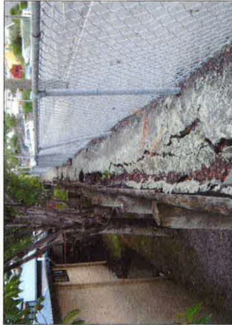
Photo 4: Cracks and subsidence above northern retaining wall
