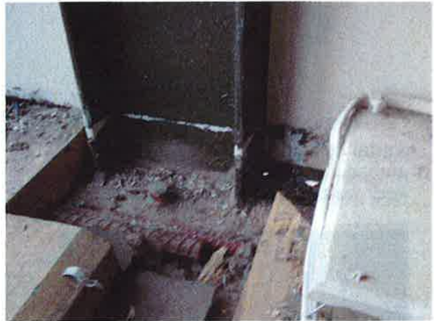
South-west gymnasium portal column: One M10 or M12 bolt fixing portal base plate to masonry wall. Base plate also welded to a bar, welded to another bar, and welded to a vertical bar cast into the wall.
