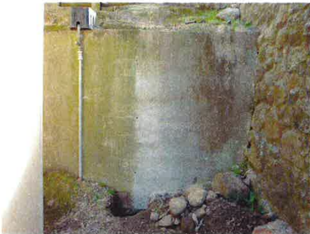
Concrete retaining wall on north side. Drilling indicates the wall is 250mm-300mm thick and reinforced.
