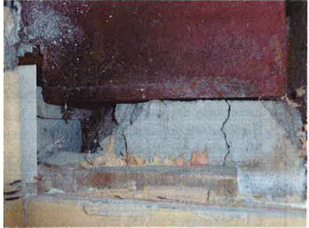
Cracking and spalling to masonry at connection with steel portal frame – south-east corner of squash courts
