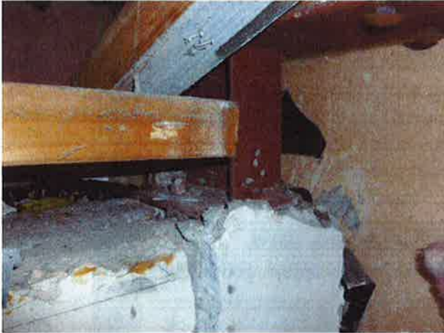
Dislodgement of masonry block at connection with steel portal frame – north-east corner of squash courts.
