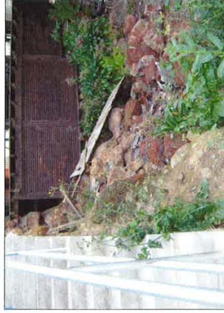
Photo 5: Failed basalt block wall on the east side
