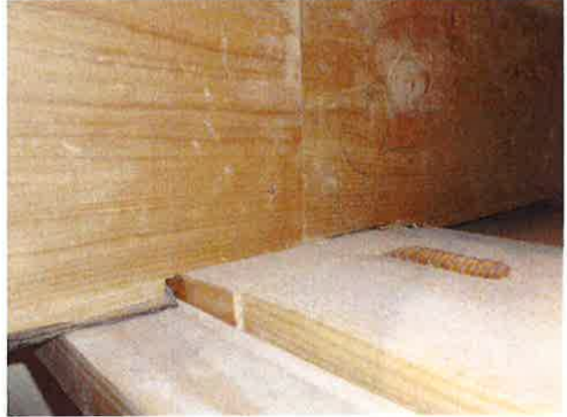
Joists fixed to top plate with 2 skew nails. Top plate fixed to masonry wall below with bent D12 bar at 600mm centres.
