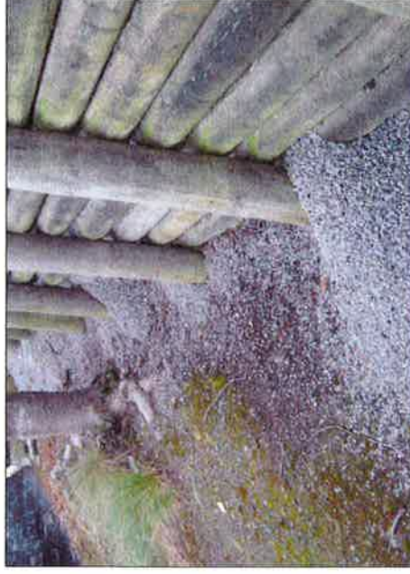
Photo 3: Talus cones of granular fill at base of upper level of northern retaining wall
