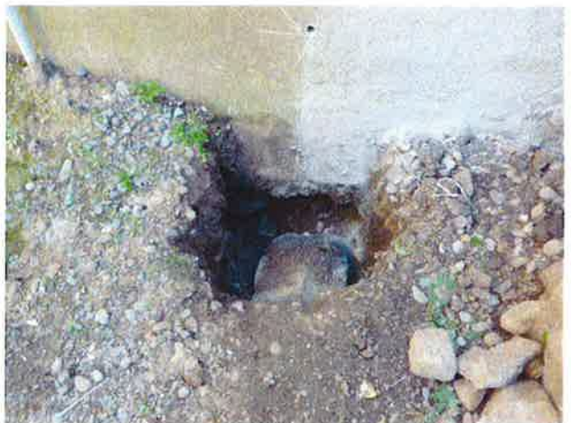
Excavation of the retaining wall footing revealed no toe footing. Drilling suggested there was no heel extending behind the wall either.
