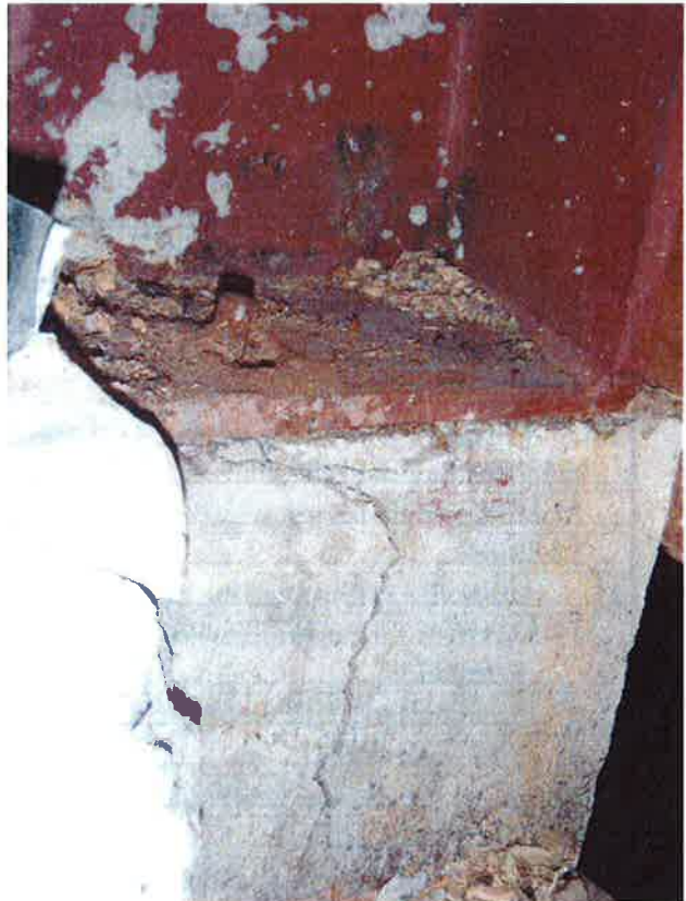
Cracking to masonry at connection with steel portal frame – squash court area
