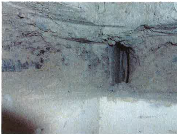
South-west corner of squash courts area: No reinforcement tying external wall into return wall.
