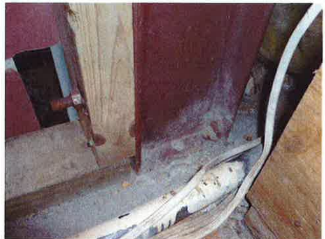
Portal column north-west column of gymnasium: No bolt fixing base plate to masonry wall below.
