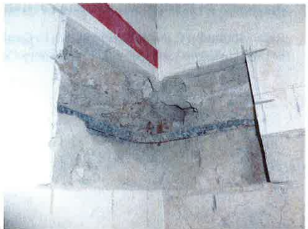
North wall of squash courts area: Return bar around corner not bent around vertical reinforcement.
