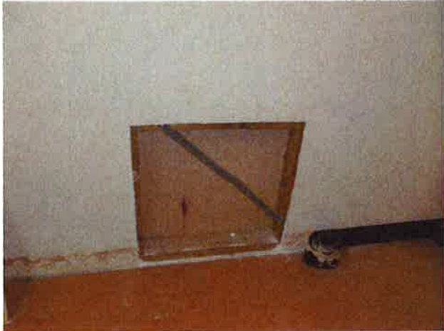
Diagonal steel brace present where detailed on original drawings.
