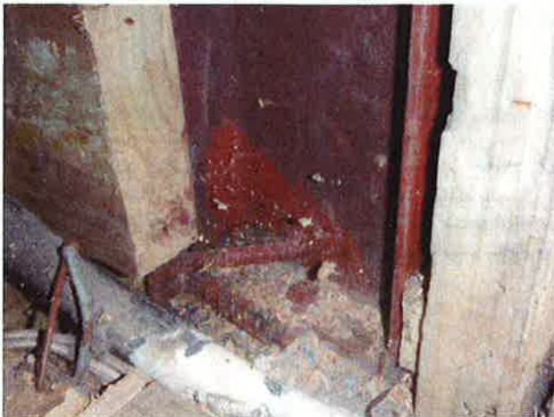
Portal column in squash courts area: Appears to be no bolt fixing into masonry wall below. Base plate welded to reinforcing bar cast into masonry wall instead.
