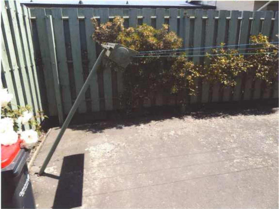
Figure 7 Rotation of the pole of the clothesline (west of unit No 2 Block A facing west)
