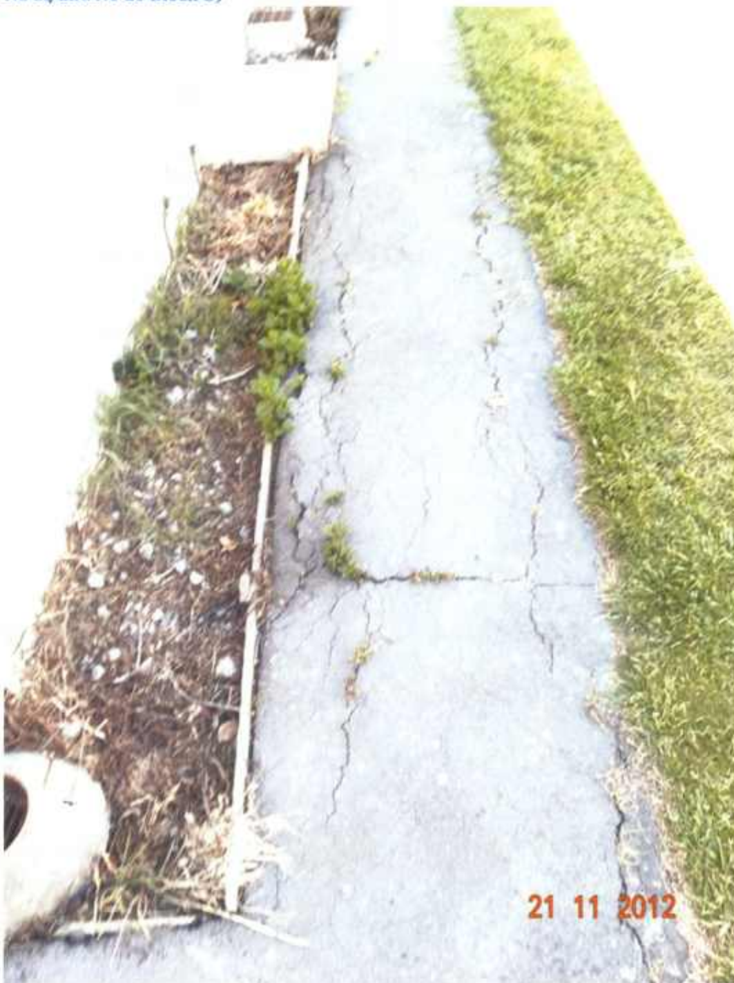
Figure 52 Several cracks along the footpath, most of these cracks are considered to be existing before the earth quake event and caused by long term consolidation settlement (between unit No 24 and No 26 Block G)
