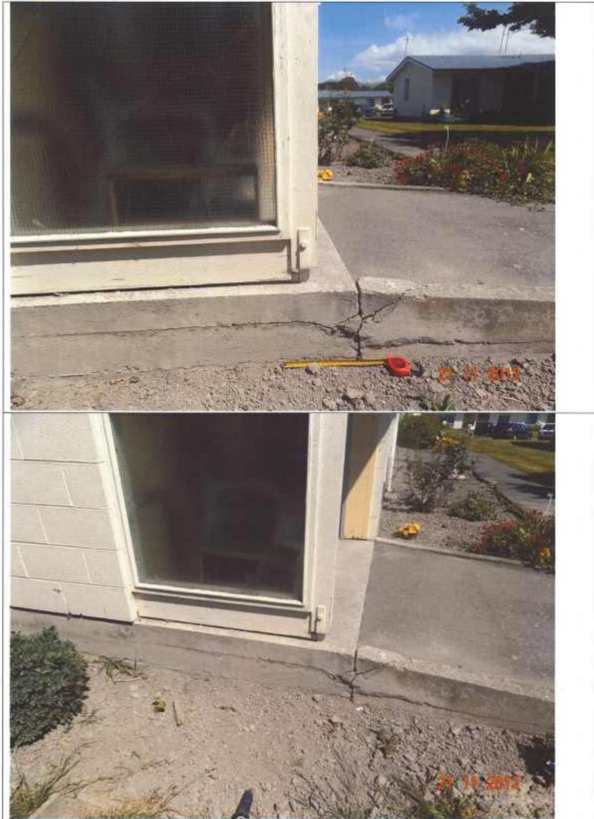
Figure 36 Crack between foundation slab and doorway, window cracked (eastside of unit No 14, block D facing south)
