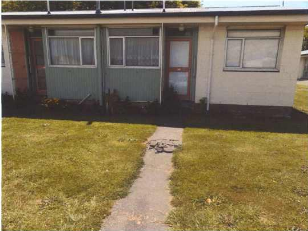
Figure 2 Major crack in pavement footpath at sand bulge (footpath towards unit No 1 (south side of block A, facing north))
