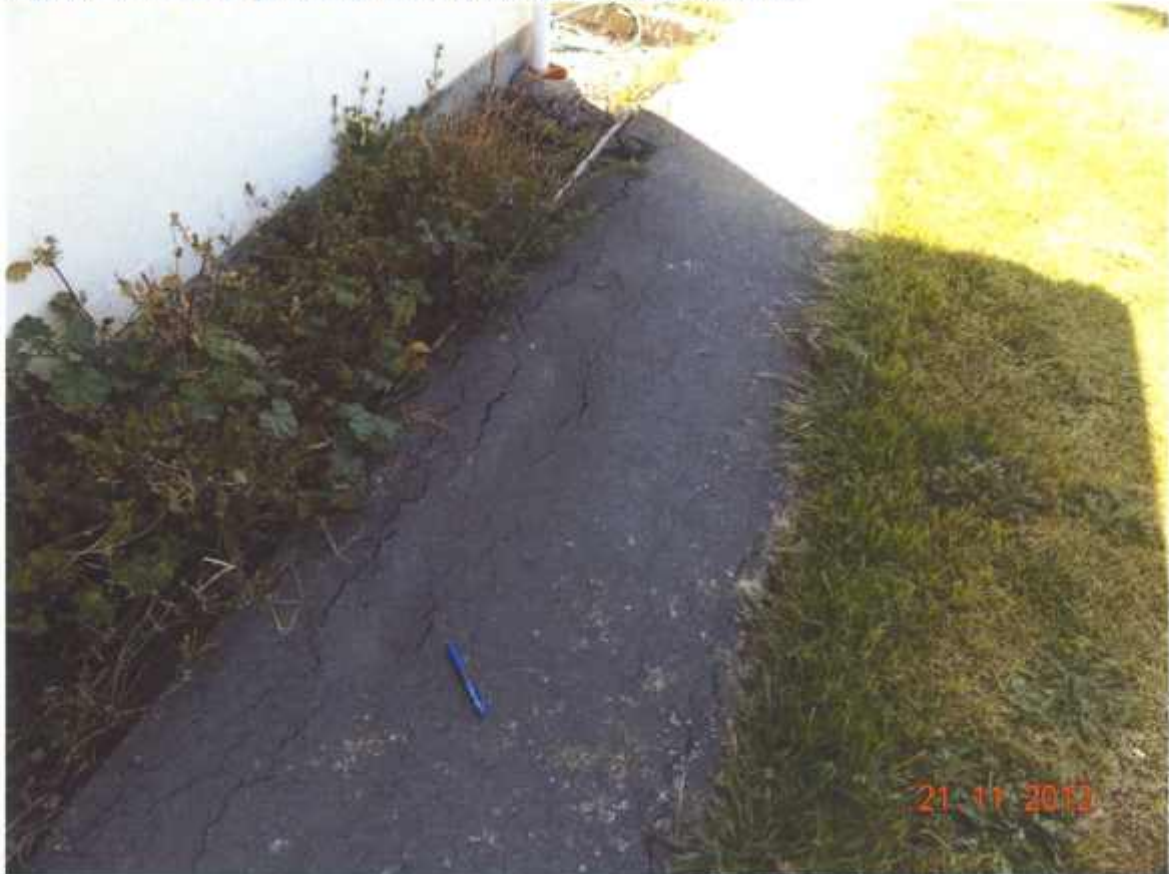
Figure 60 Cracks in pavement (next to No 29 and No 30 block H)
