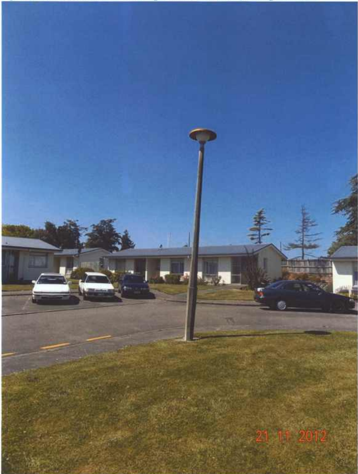
Figure 59 Visible rotation of the street light towards east (unit 30 facing north east)
