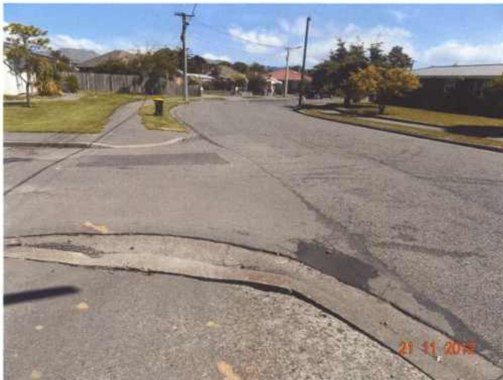
Figure 11 Cracks of drive way and repair (Block B, unit No 3 facing south)
