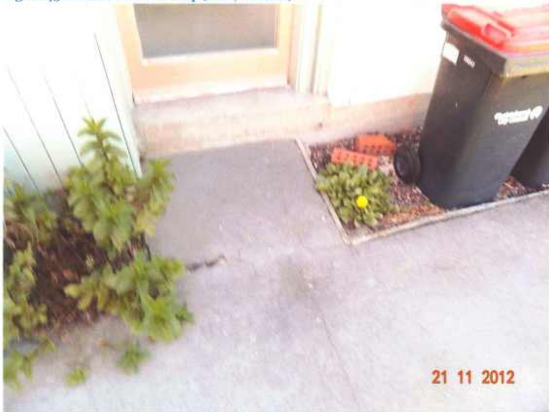
Figure 45 Cracks in the doorstep (No 17 Block E)
