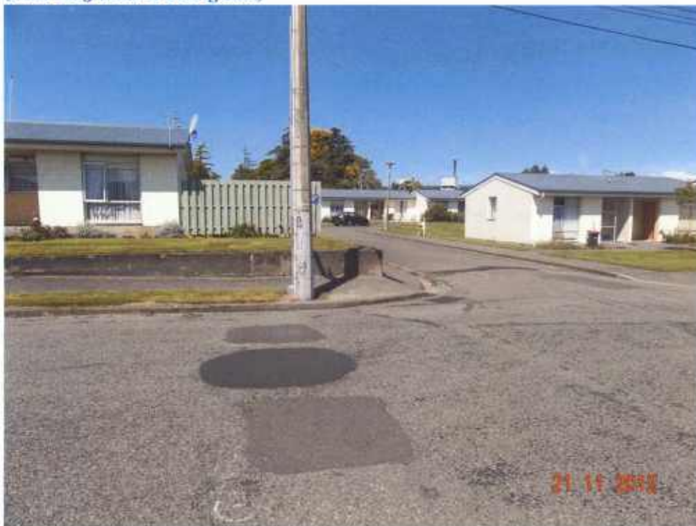
Figure 14 Bend on the end of drive way facing east, various repair work of asphalt cracks (Unit No 3 block B facing east)
