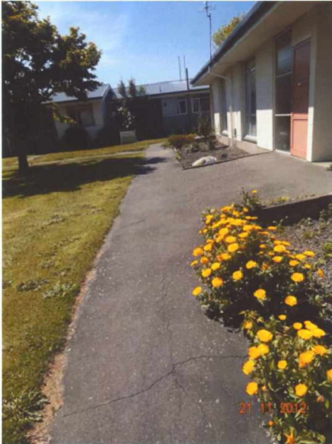
Figure 37 Minor cracks on footpath (west face of units No 14 and No 15 Block D facing north)
