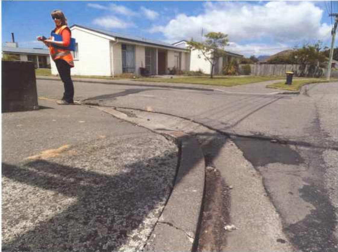
Figure 13 Bend on the end of the drive way, repairs of cracks visible general depression of the pavement visible (Unit No 3 of Block B facing north)
