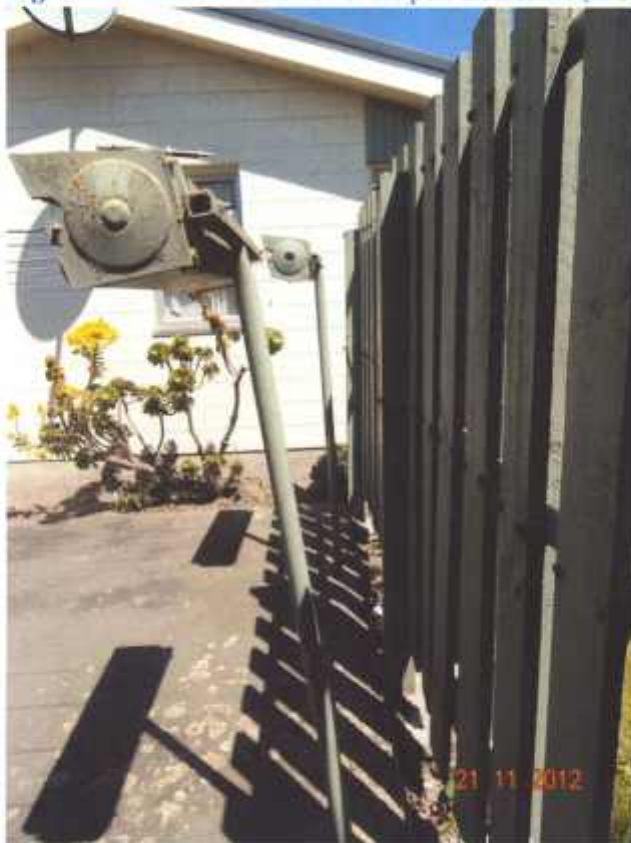
Figure 26 Distinctive rotation of the pole clothesline (in between unit No 13 and No 14, block C and D)
