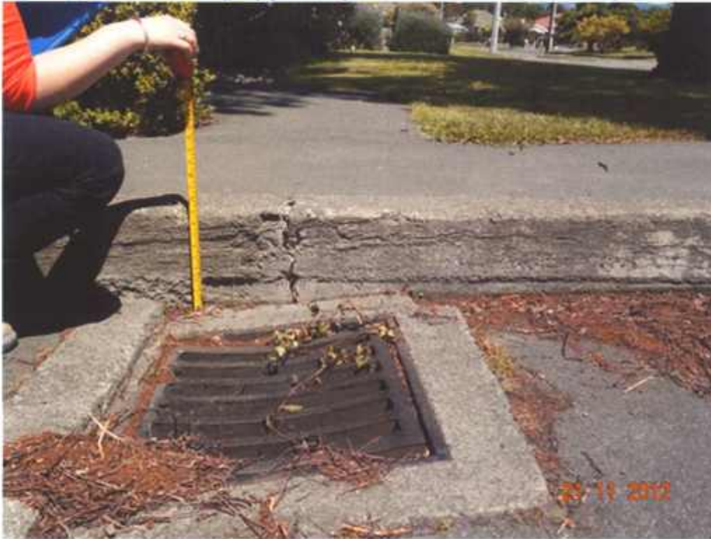
Figure 34 Rotation of the gully pot (detail at car park north of unit No 7, Block B/C)
