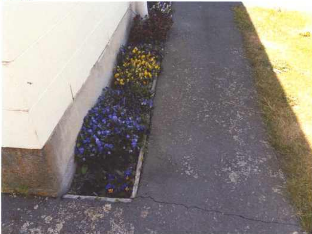
Figure 19 Cross cracks around the corner of the pavement of footpath (unit No 5 and No 6 of Block B)
