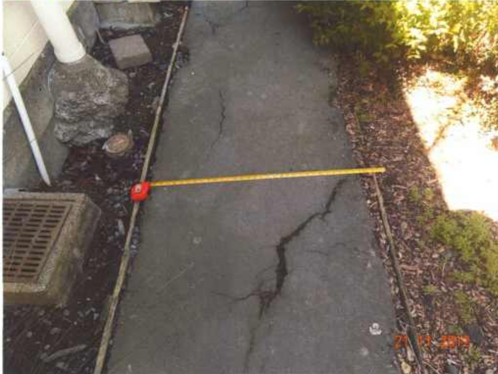
Figure 55 Recent crack along the footpath (unit No 24 – No 26, block G)
