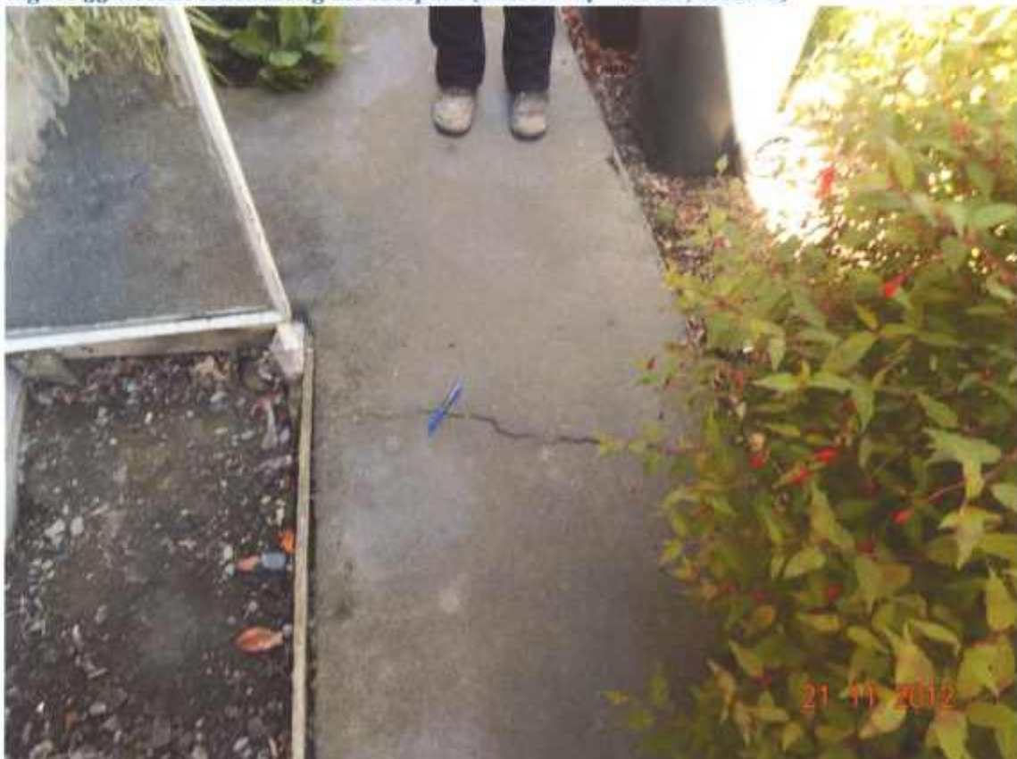
Figure 55 Recent crack along the footpath (unit No 24 – No 26, block G)
