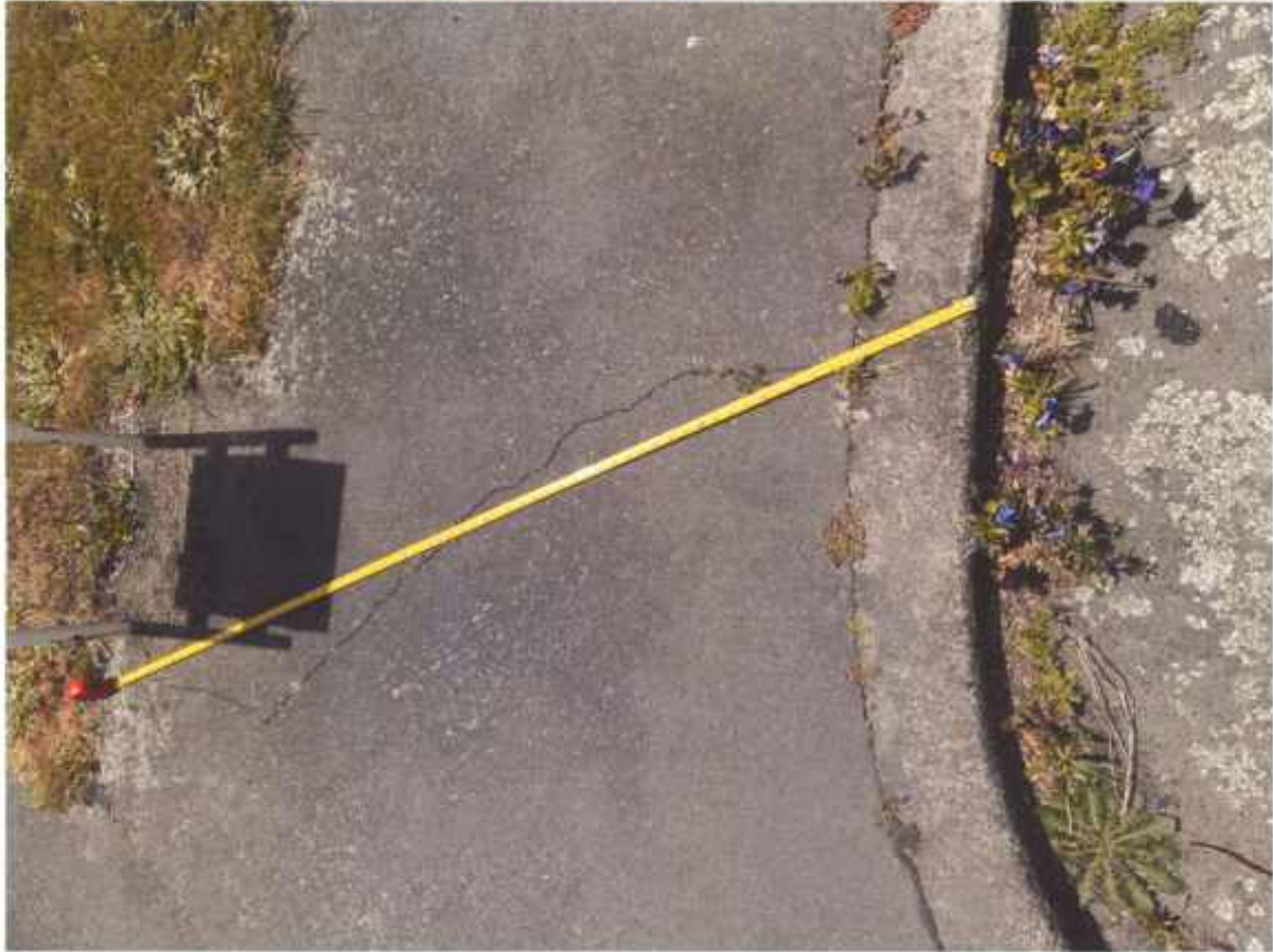
Figure 10 Crack of the pavement (unit No2 Block A, facing south-west)
