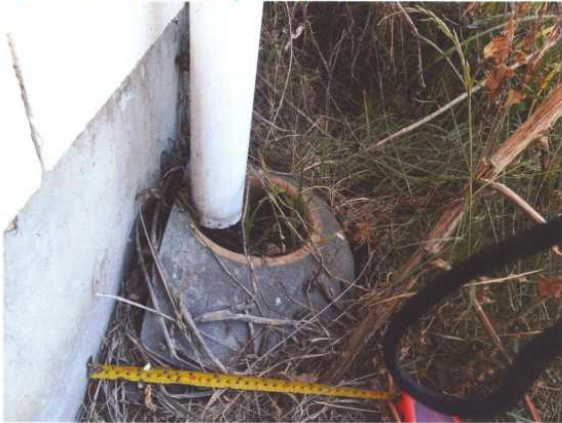
Figure 22 Defect of a waste water trap (unit No 4 block B)
