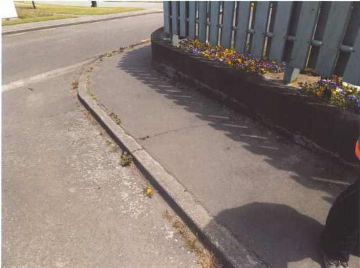
Figure 10 Crack of the pavement (unit No2 Block A, facing south-west)
