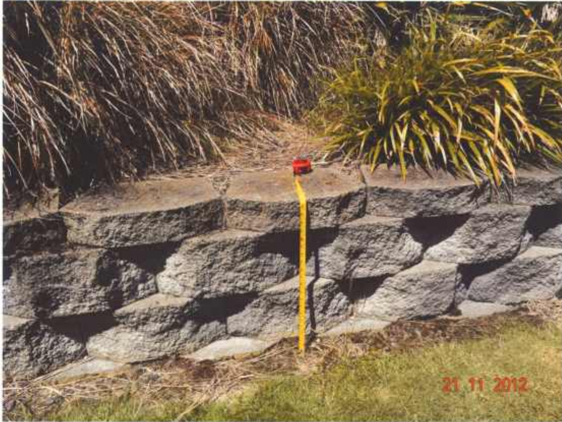
Figure 24 Block retaining wall, no defects observed (opposite unit No 13, Block C)
