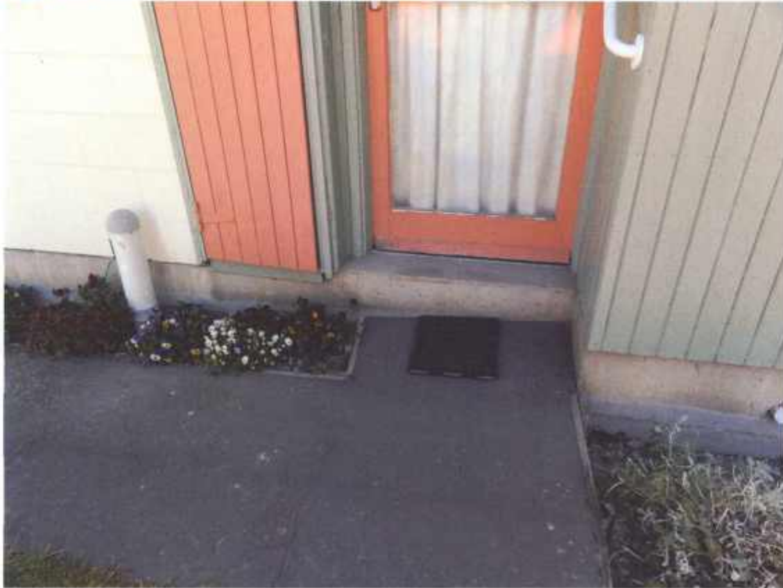
Figure 20 Differential settlement (total \pm 10 cm) of doorstep unit No 5 Block B
