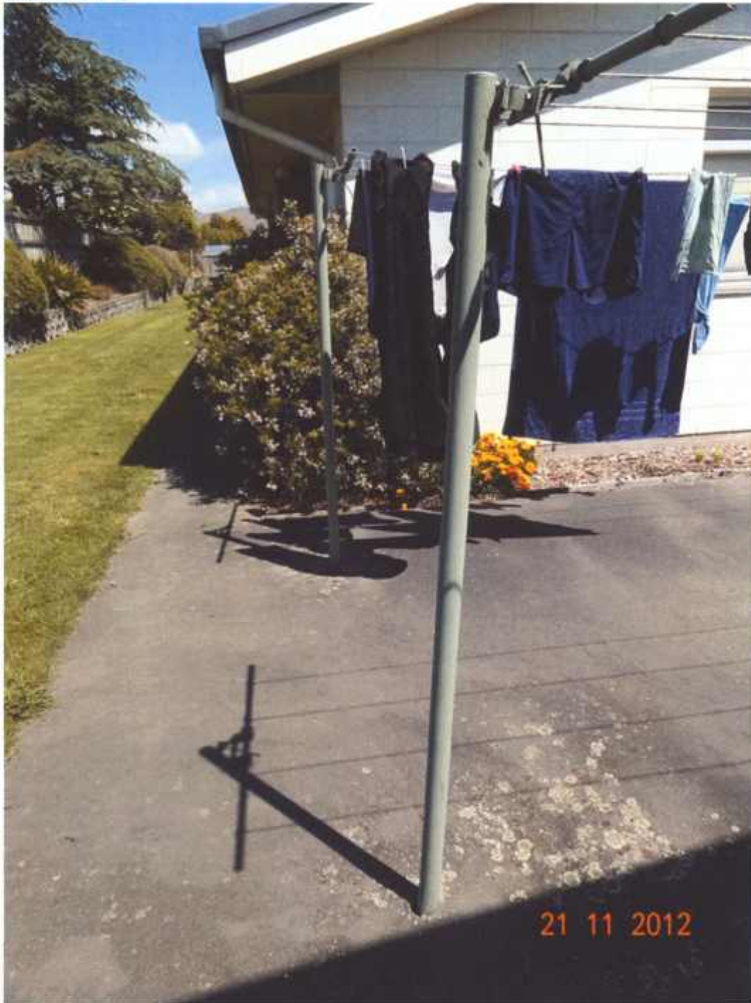
Figure 47 Distinctive rotation of the pole of the clothesline (between unit No 16 and no 17 block D and E)
