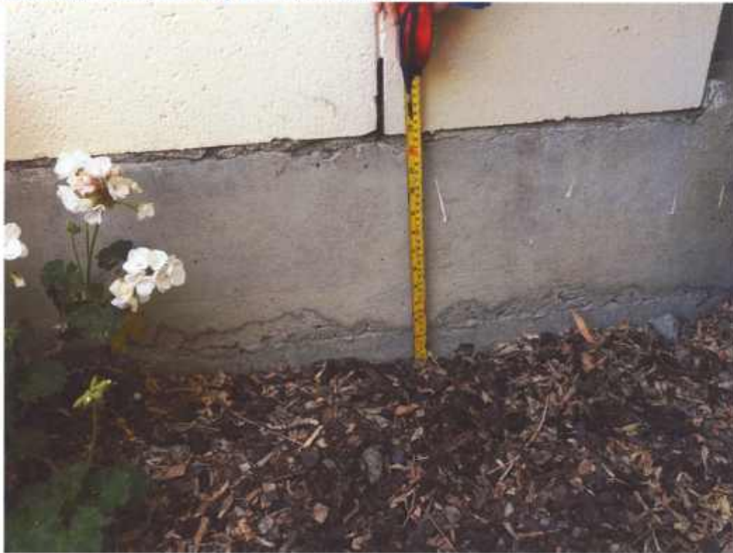
Figure 19 Cross cracks around the corner of the pavement of footpath (unit No 5 and No 6 of Block B)
