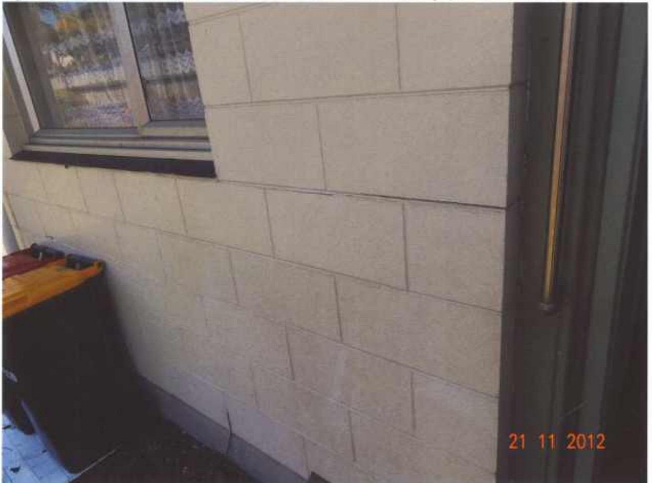
Figure 40 Horizontal cracks in in the mortar of the concrete masonry (No 16 of block D)
