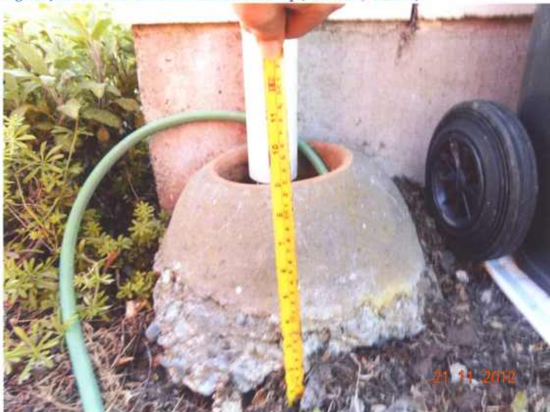
Figure 46 Settlement under the waste water trap (near no 17 block E)
