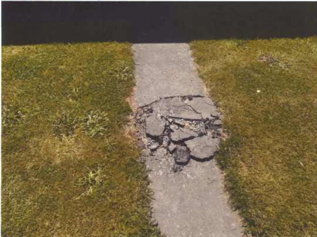
Figure 3 Close-up of sand bulge and cracks in the pavement (footpath towards unit No 1 southside of block A, facing north)
