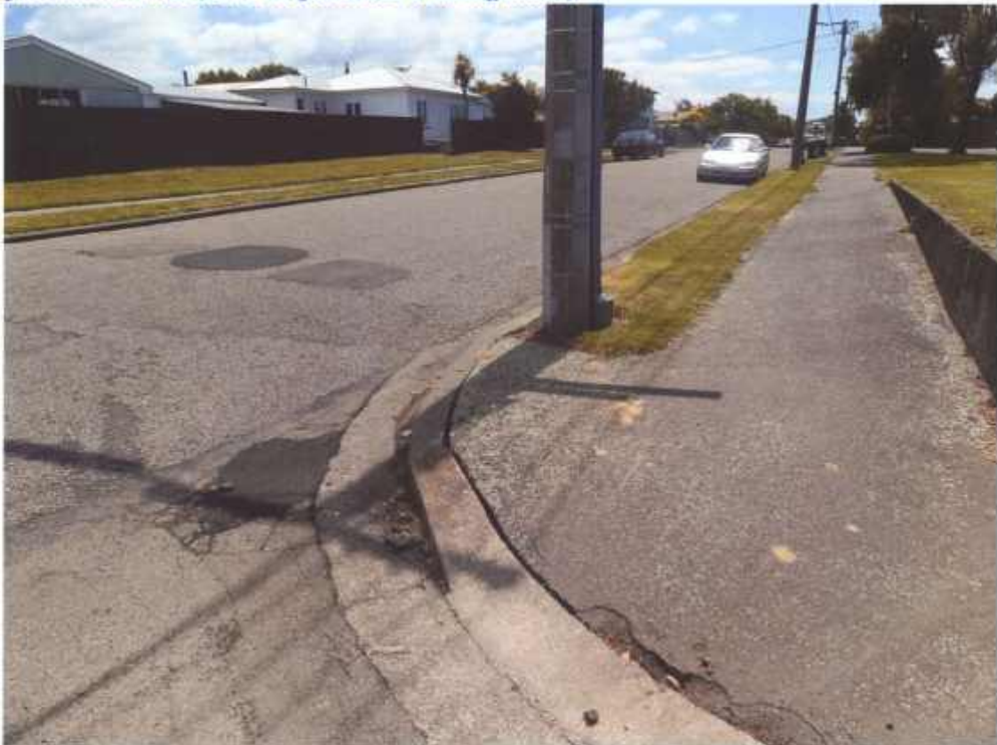
Figure 13 Bend on the end of the drive way, repairs of cracks visible general depression of the pavement visible (Unit No 3 of Block B facing north)
