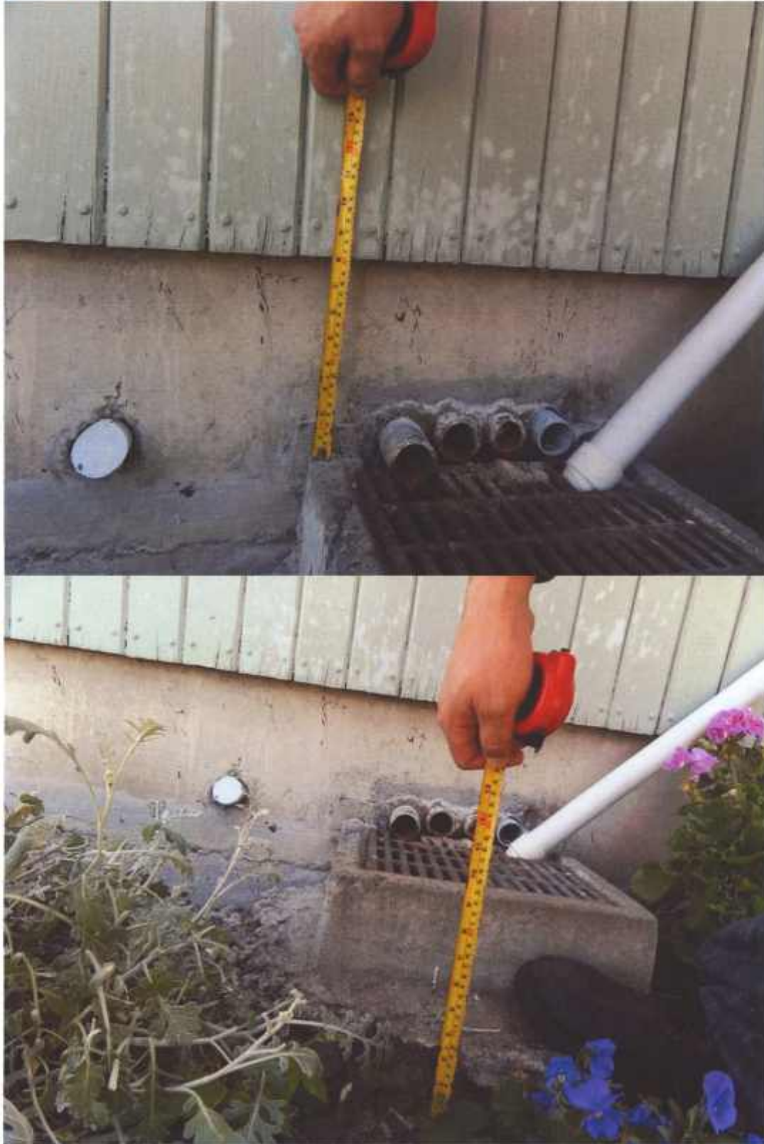
Figure 21 Close-up of gully pot; vertical displacement and depression under gully pot (unit No 4 block B)
