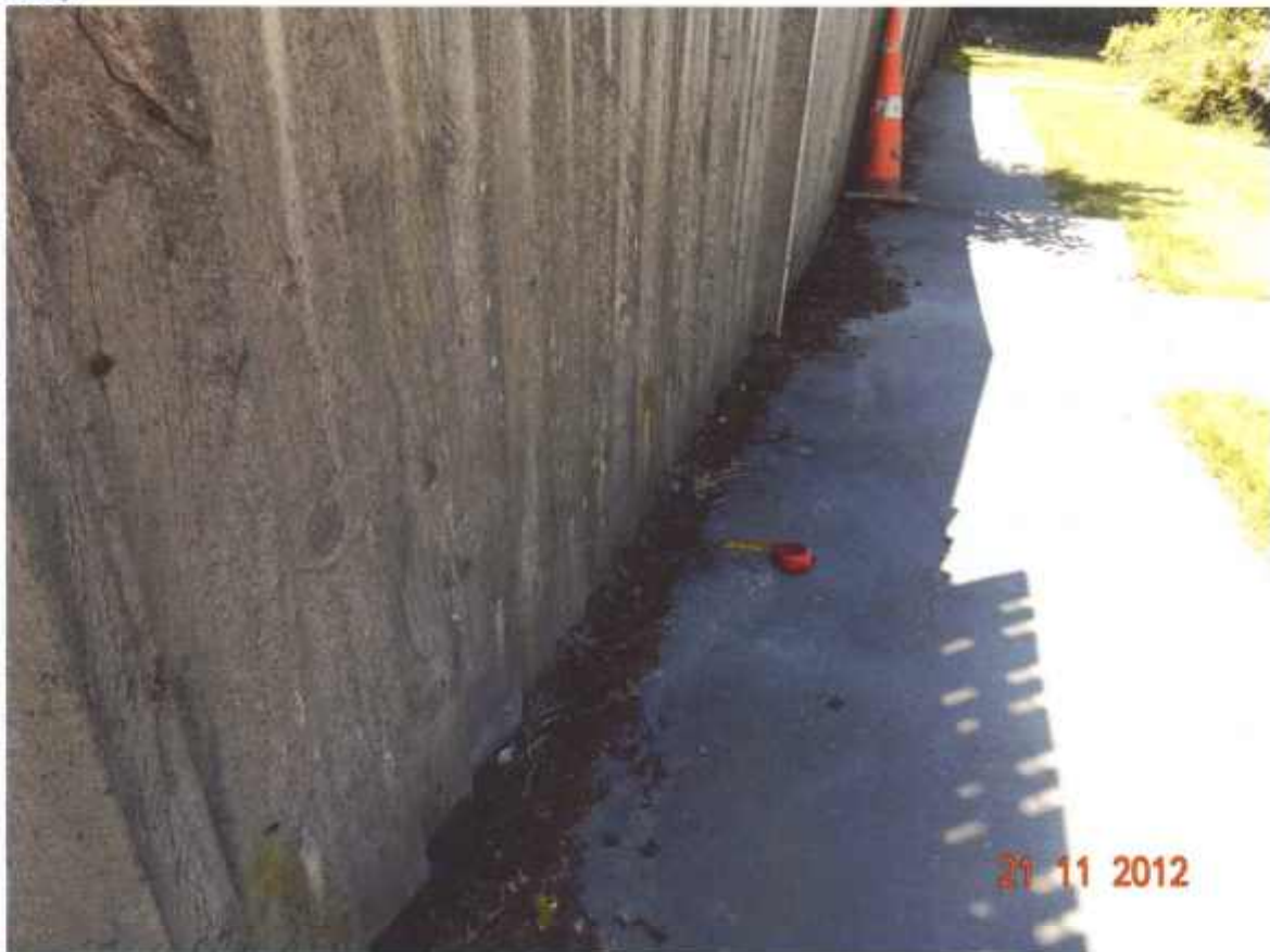
Figure 28 Pavement of the footpath pushed up, possibly due to a sand well. There is a safety cone placed next to the footpath to indicate this defect (north of unit No 10 Block C, facing east).
