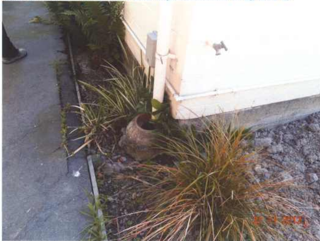
Figure 56 Settlement under waste water trap (corner of unit No 24, Block H)
