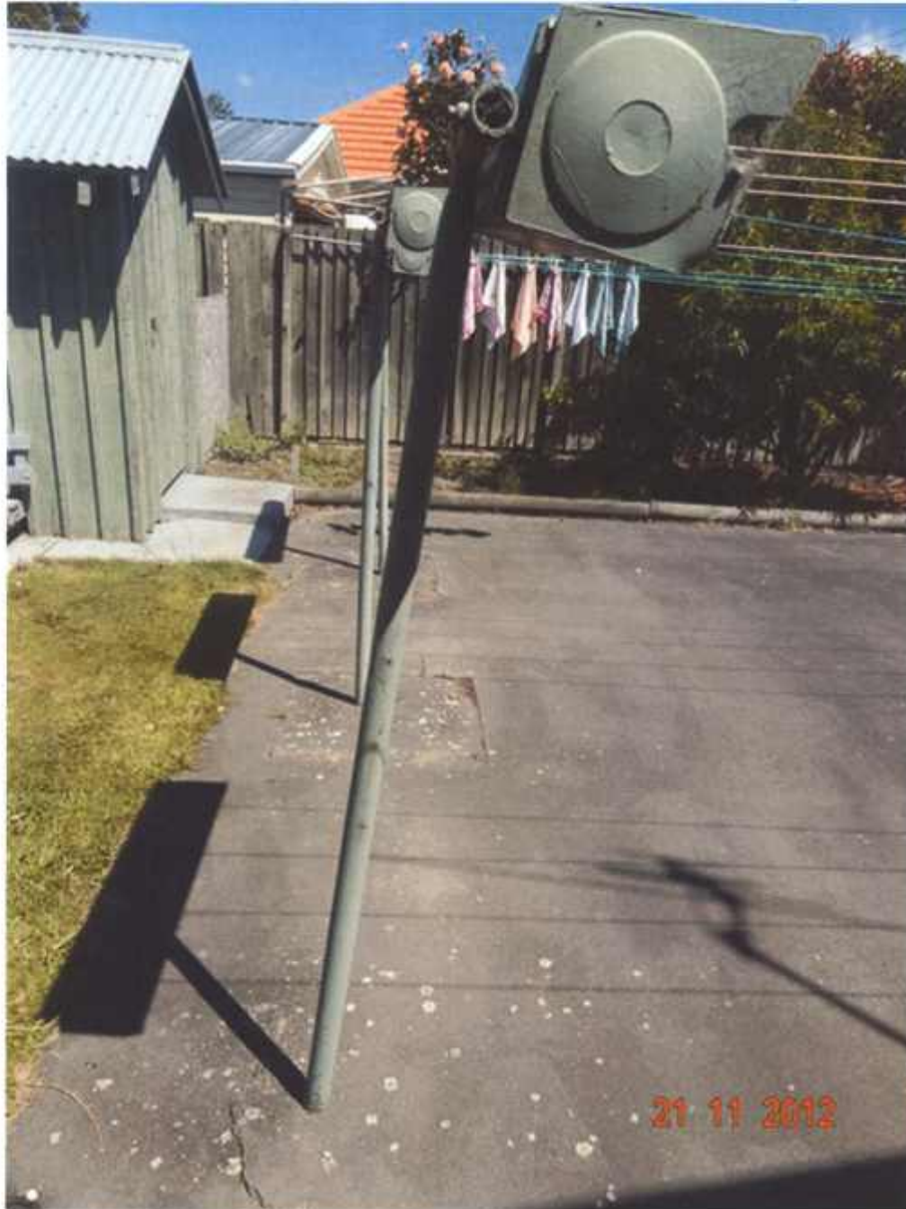
Figure 49 Rotation of the pole of the clothesline (No 23 of block F facing south)
