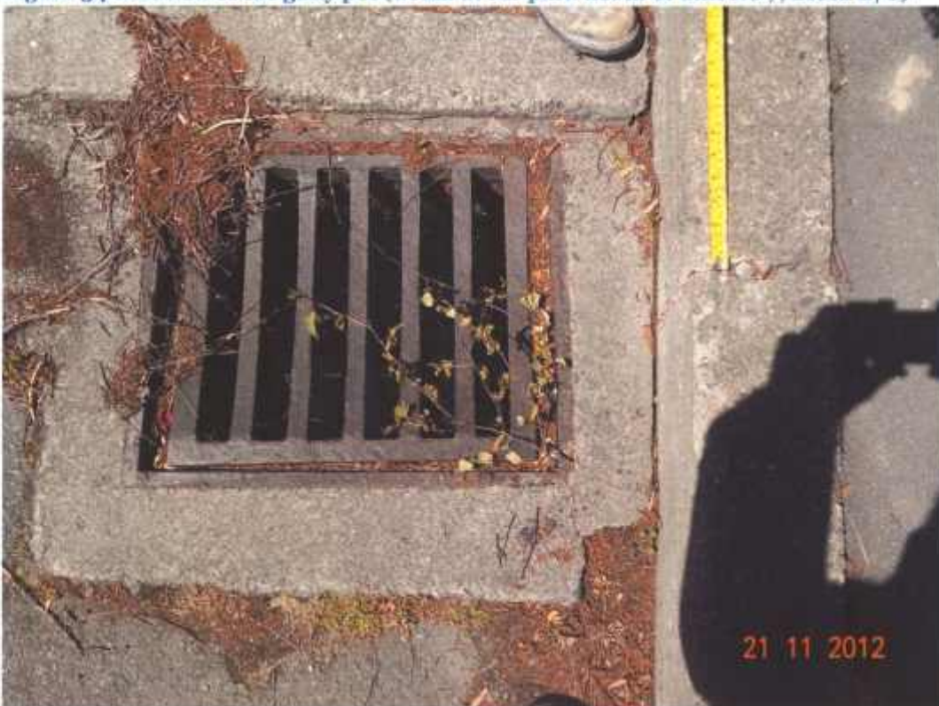
Figure 34 Rotation of the gully pot (detail at car park north of unit No 7, Block B/C)
