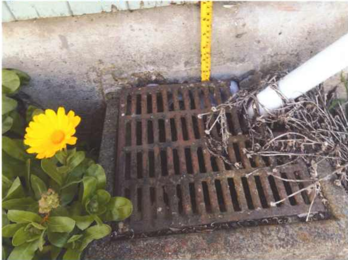
Figure 8 Settlement of the gully pot (unit No 2 Block A)
