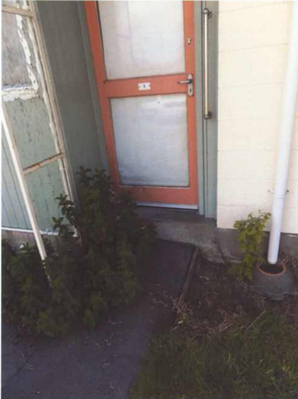
Figure 4 Doorstep settlement; settlement under waste water trap (unit No 1 Block A)
