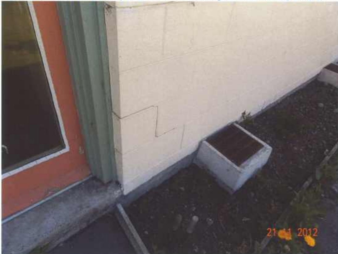
Figure 51 Cracks in the masonry wall, next to the doorstep of (unit No No 23 Block F)
