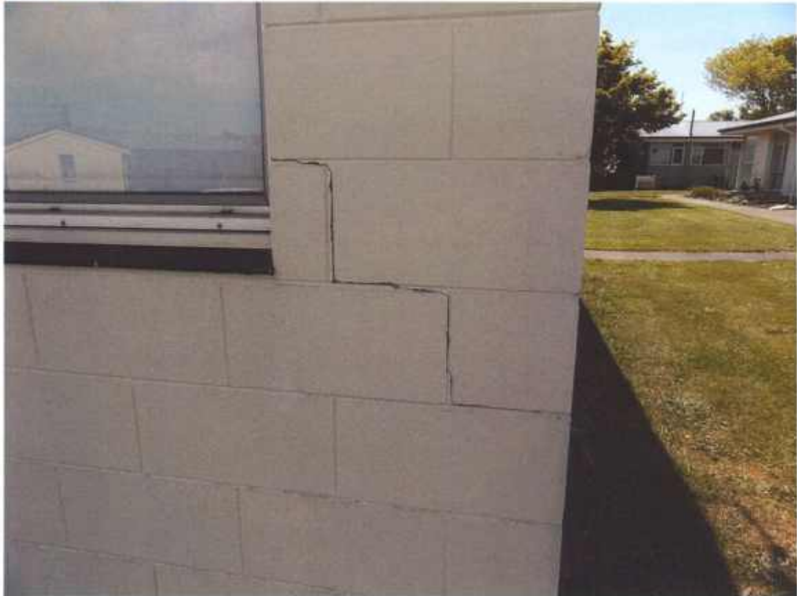
Figure 6 Cracking in the mortar of the concrete masonry wall (around the corner of unit No 1 block A facing north)
