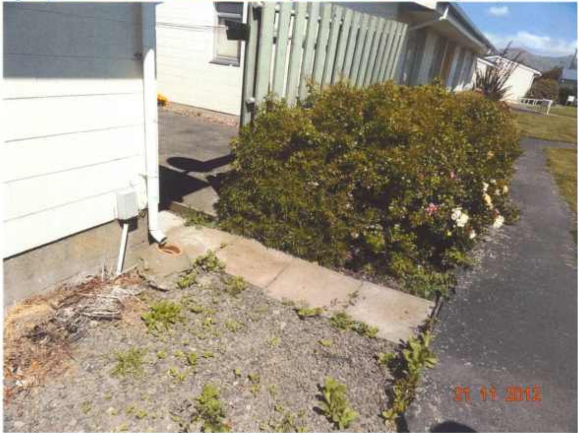
Figure 38 Settlement under the waste water trap (unit No 16 Block D, facing south)
