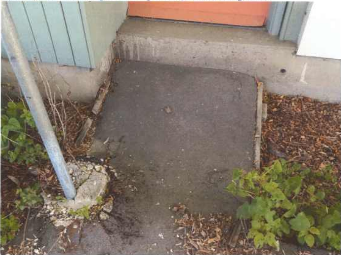
Figure 17 Detail of cracking (at doorstep of unit 5 Block B facing south)
