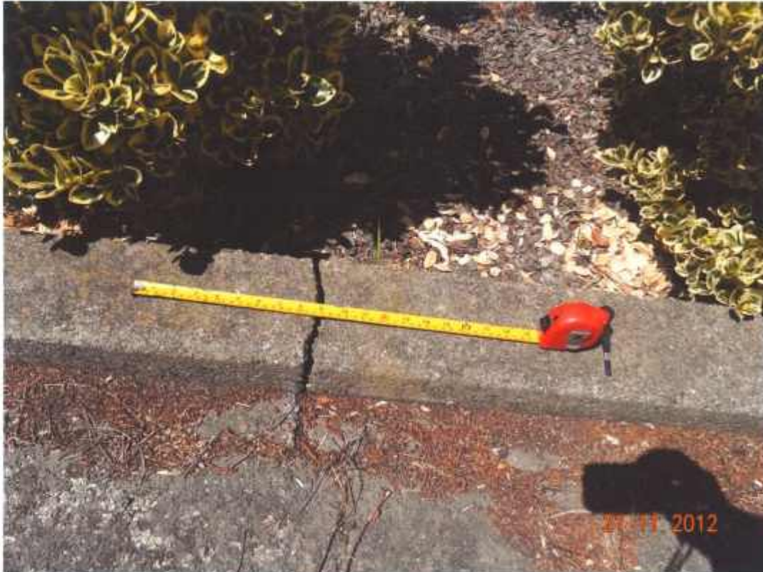
Figure 32 Other detail of crack in kerb (to No 8, west of Block C, facing East)
