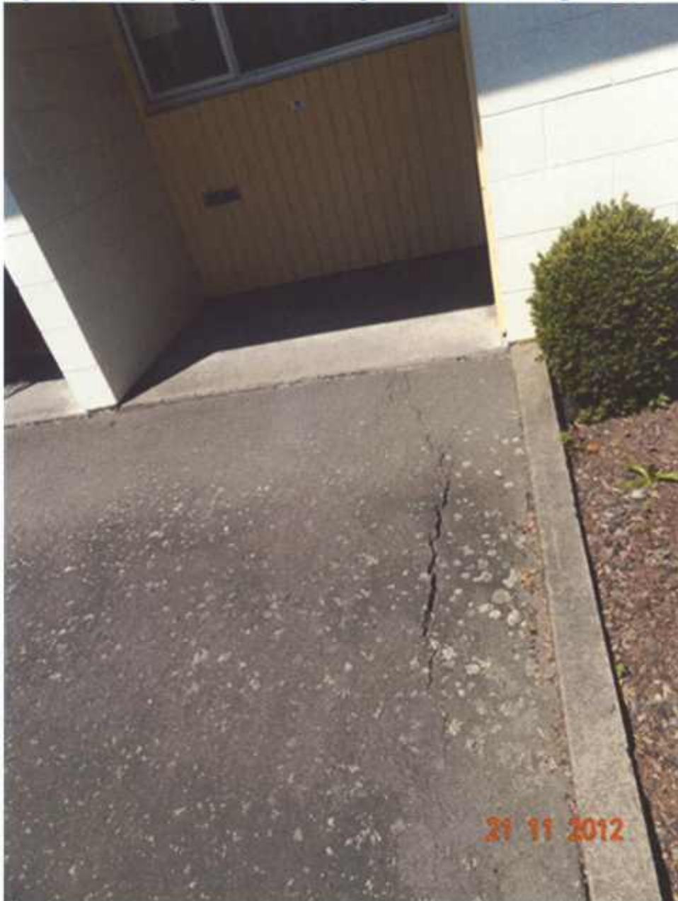
Figure 48 Crack in asphalt of the doorstep (No 18 Block E, facing east)
