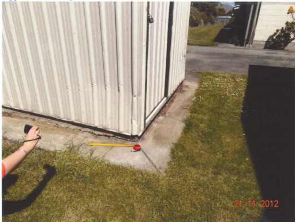
Figure 25 Settlement under west side of the mini-container, also cracks along the concrete (opposite unit No 13 of Block C)
