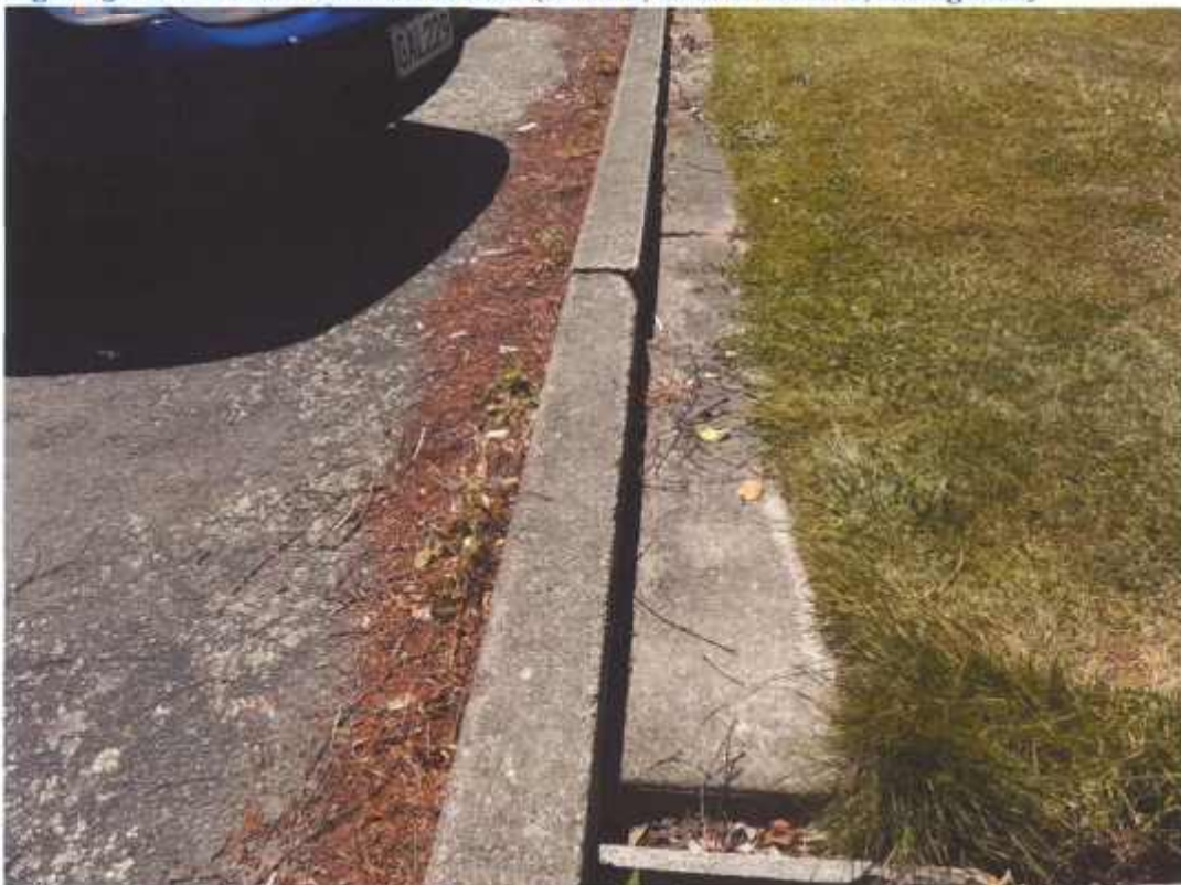
Figure 32 Other detail of crack in kerb (to No 8, west of Block C, facing East)
