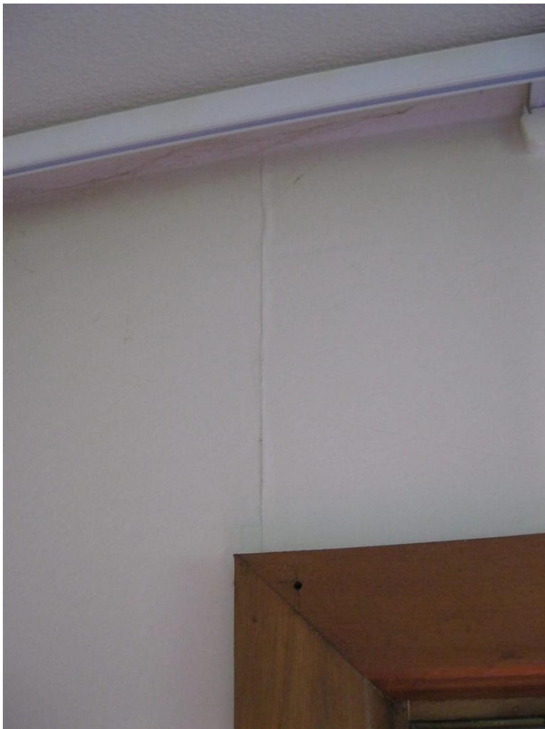
Photograph 6 Vertical cracking in plasterboard wall lining.
