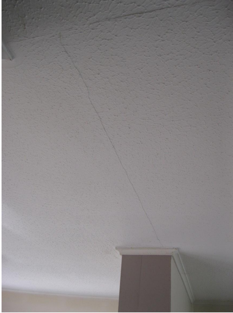
Photograph 7 Cracking to plasterboard ceiling lining where the original chimneys were removed.
