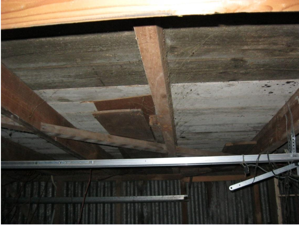
Photograph 7 Bracing at the roof level.
