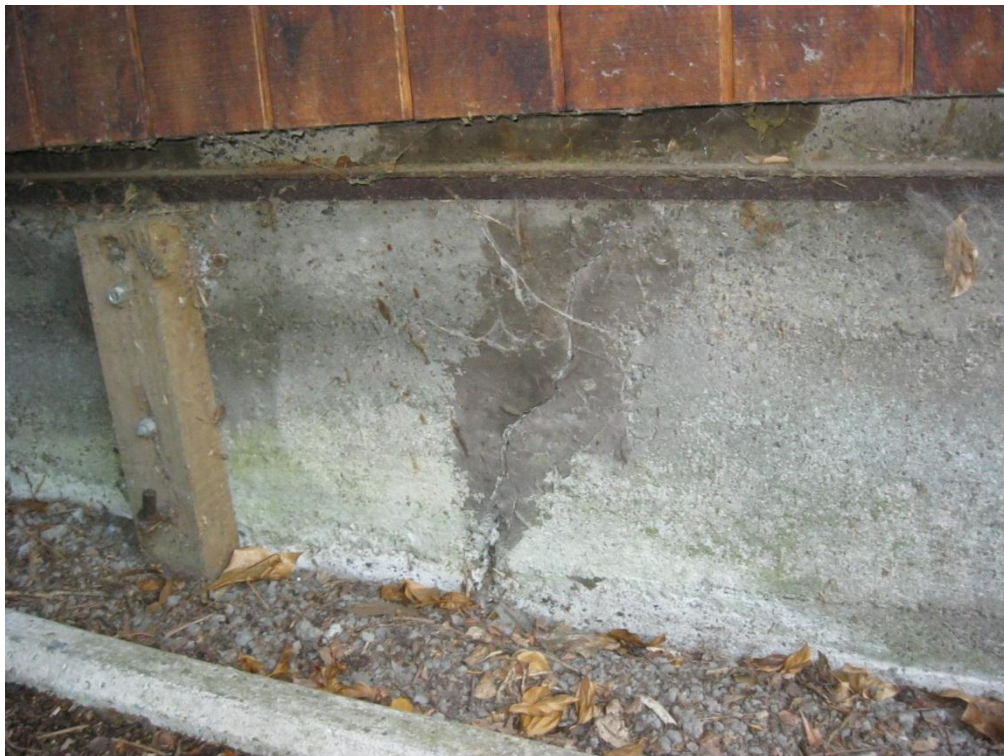
Photograph 10 Cracking of the concrete perimeter beam foundation- longitudinal wall
