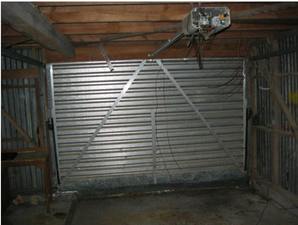
Photograph 8 View of the corrugated steel doors from the inside.
