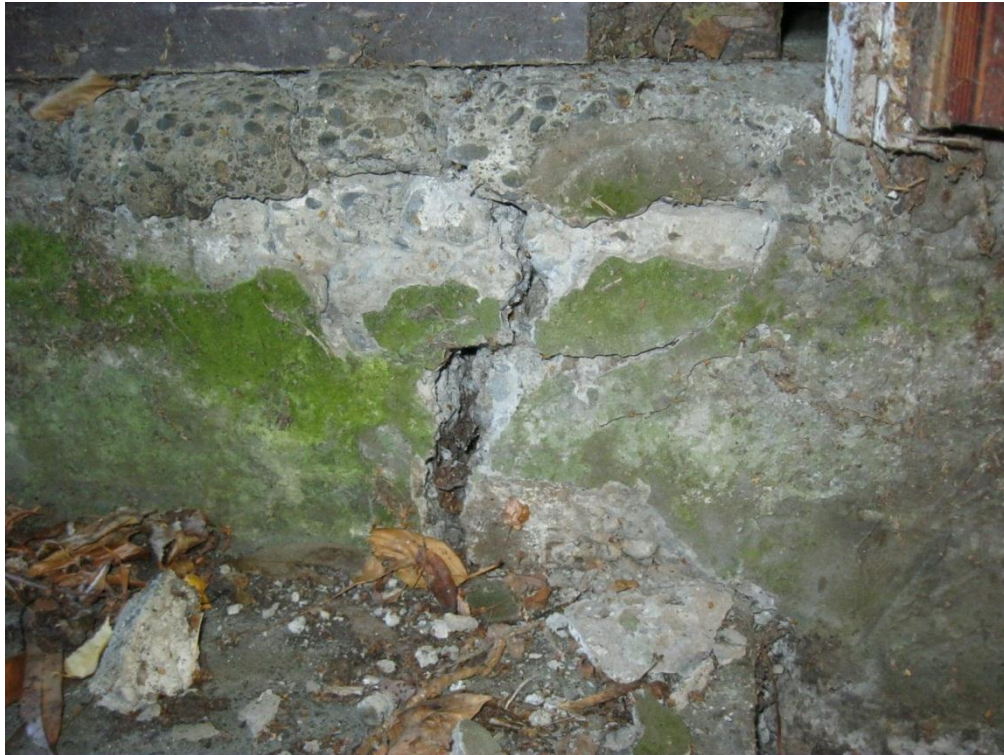
Photograph 9 Cracking of the concrete perimeter beam foundation- longitudinal wall
