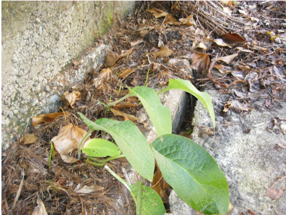
Photograph 11 Lateral spreading between foundation of the building and surrounded pathway.
