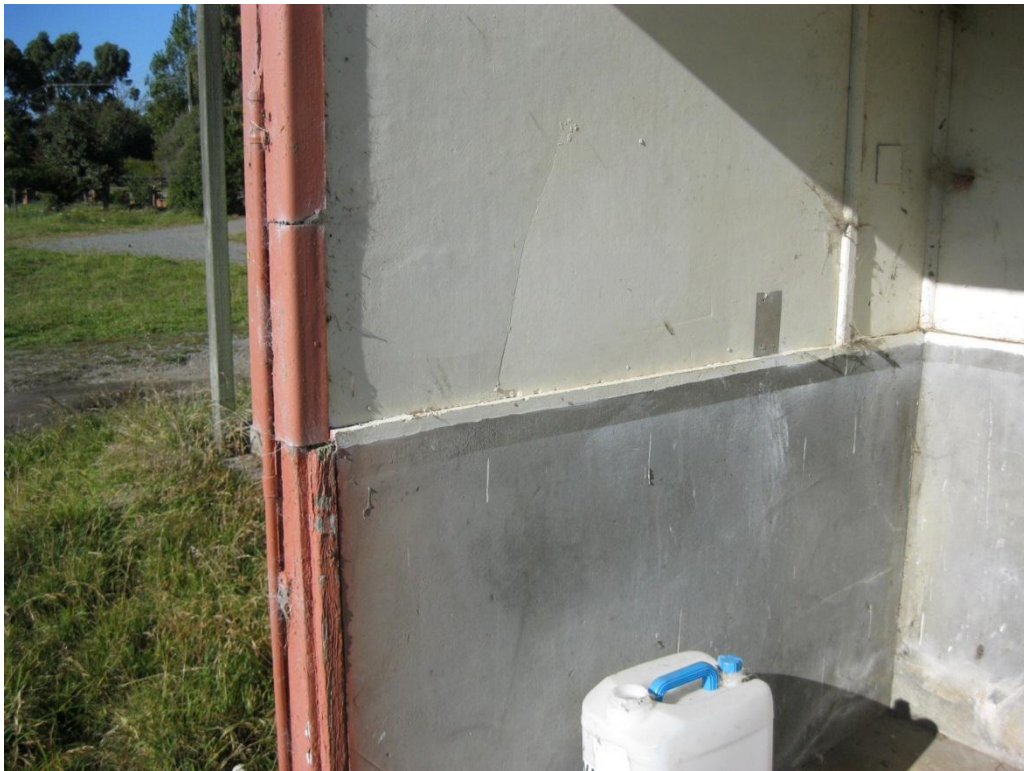
Photograph 6 Cracking to the timber frame lining that is not believed to be earthquake related.
