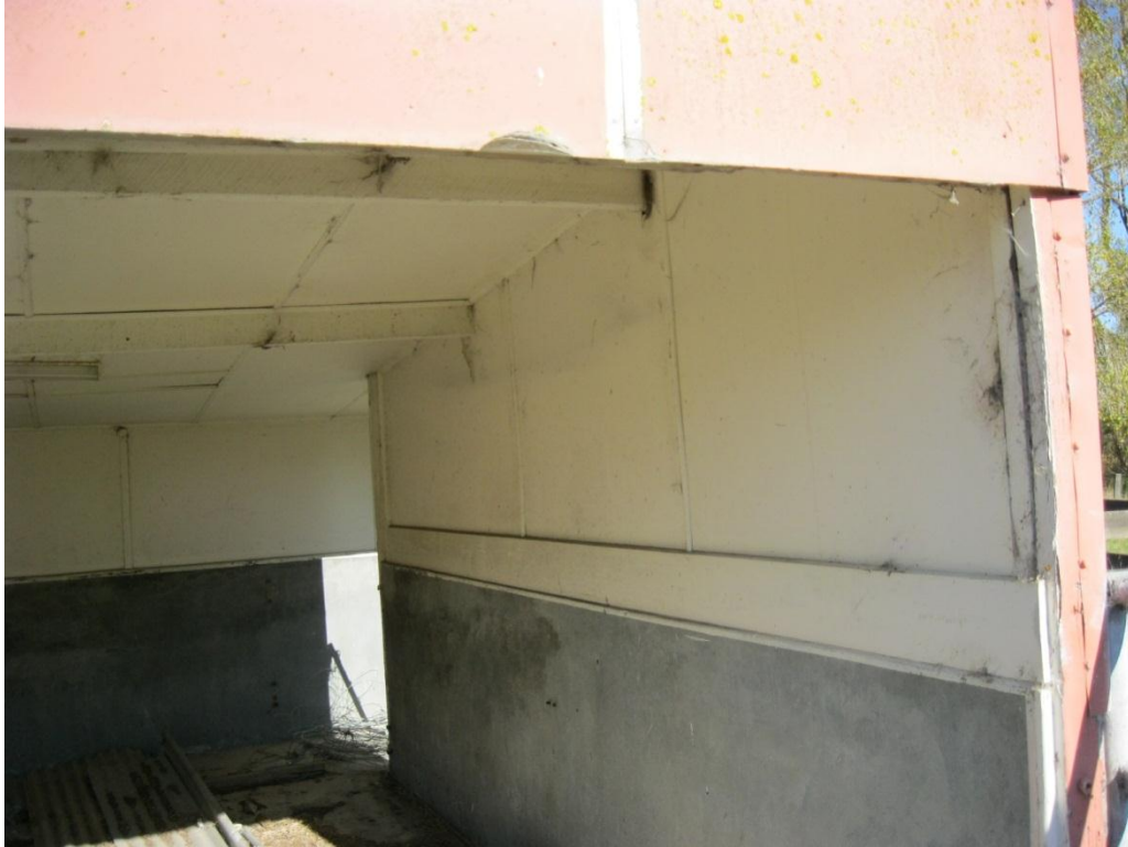
Photograph 5 View of the interior at the south-eastern wall of the building. Wall and roof linings and roof joists are clearly visible.
