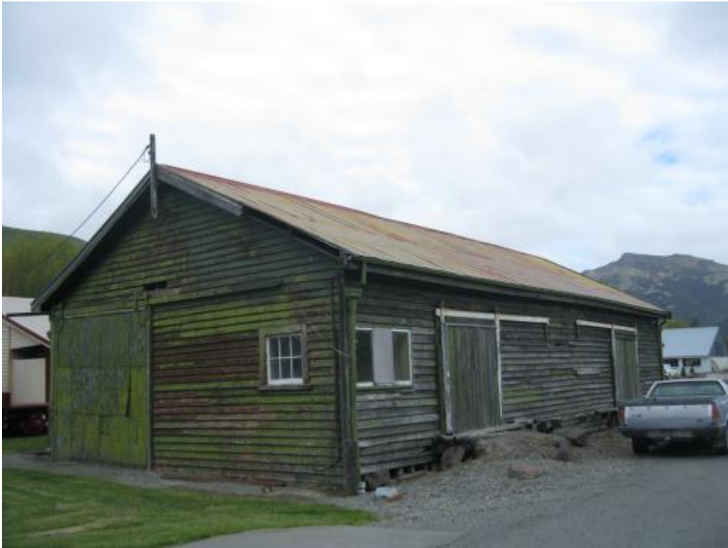
Photograph 1 View of Barn from the north.
