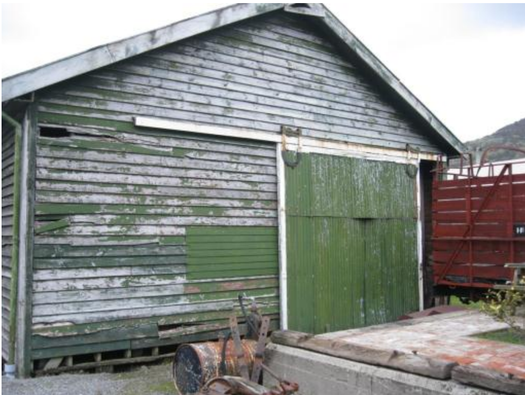
Photograph 4 Southwest elevation of the barn.
