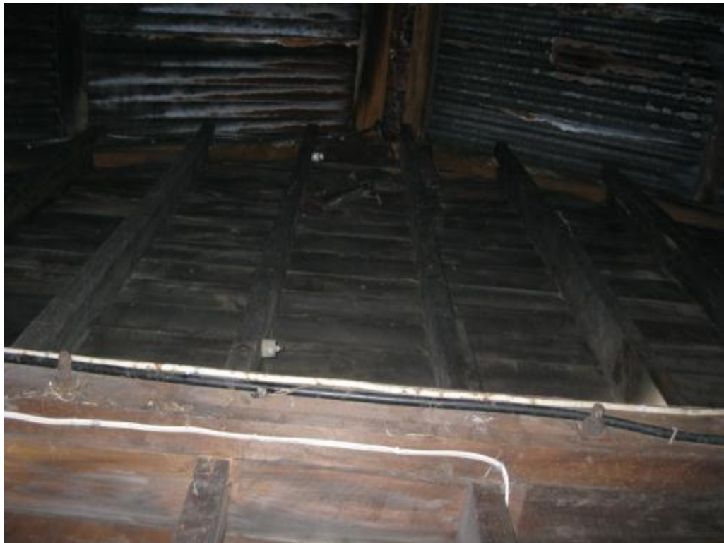
Photograph 8 Gable end of timber framed wall.
