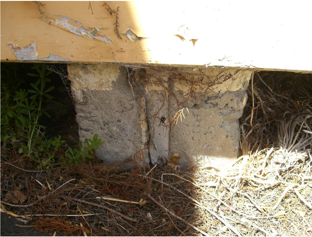
Photo 5: View of a concrete pile under the kitchen area of the building
