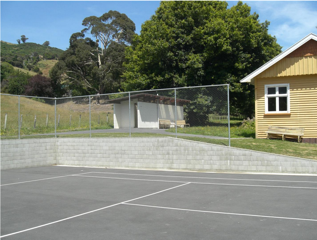
Photo 9: Concrete cantilevered wall on the east side of the hall
