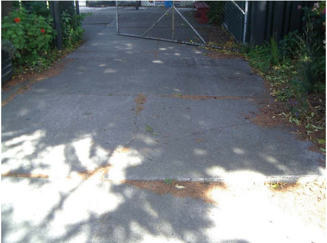
■ Figure 8 Damaged paving slabs at Linwood Resource Centre
