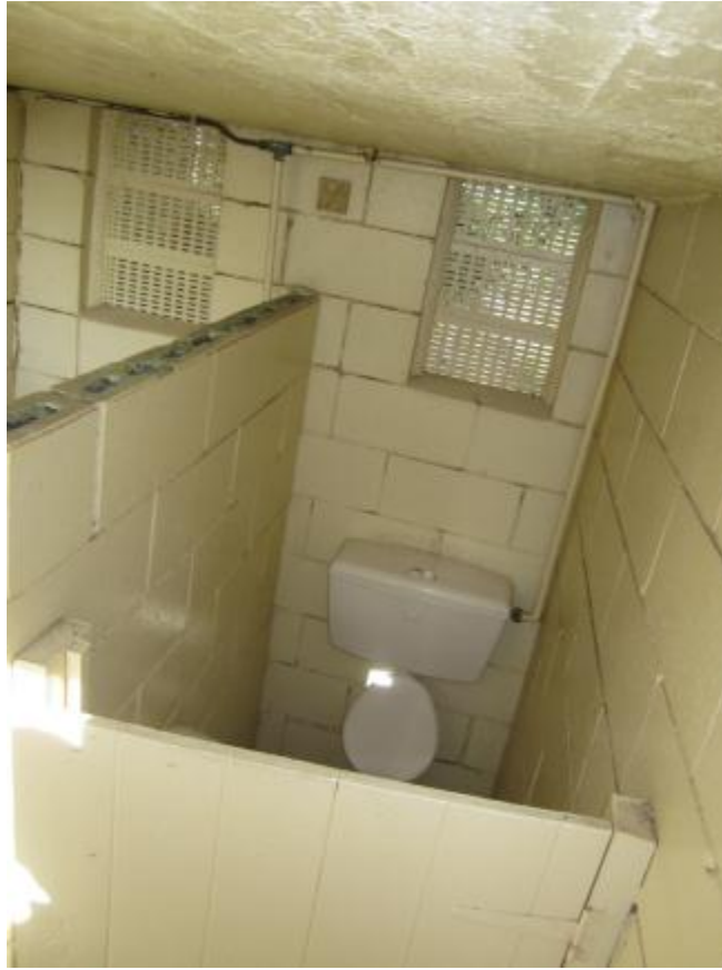
Photograph 3 Partial height wall on left and full height wall on right
