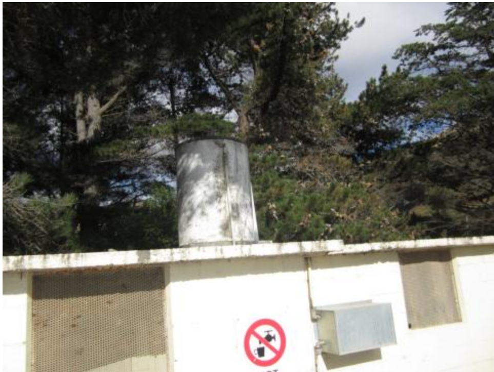
Photograph 4 Water storage tank on roof of structure
