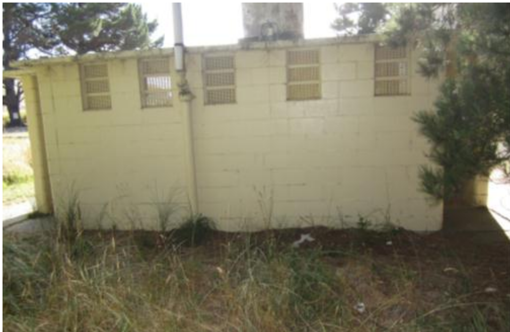
Photograph 2 Western elevation of structure
